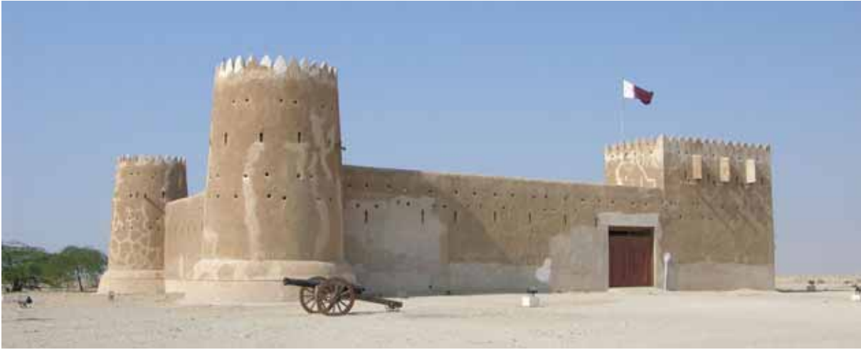
Plate 6. Qal'at Al-Zubarah, State of Qatar. The fort after the preservation works carried out by Qatari Authorities (© UNESCO; photo by Guido Licciardi).
