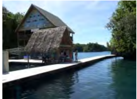
Figure 29. The Dolphins Pacific Research facility at Ngeruktabel.
