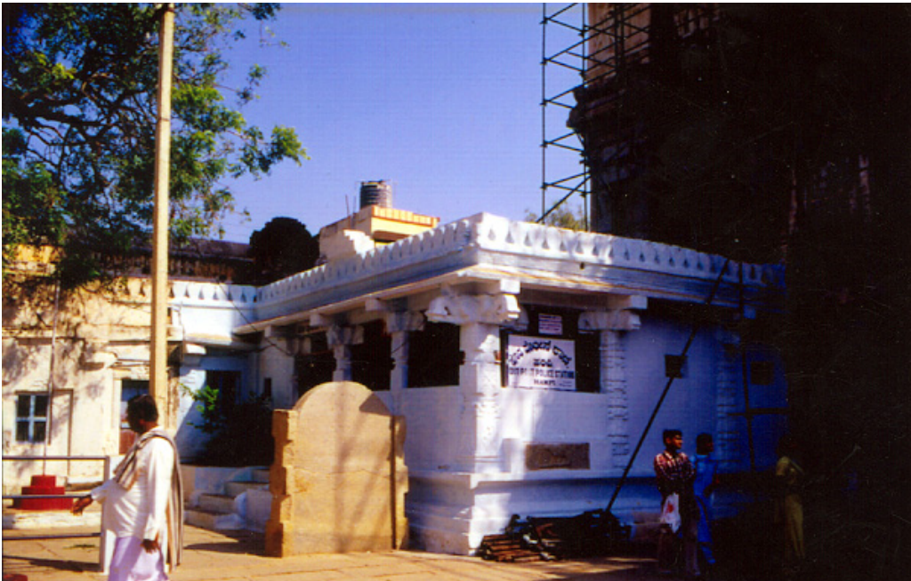
PLATE CII VIRUPAKSHA TEMPLE, INNER COURTYARD: ENCROACHMENTS
