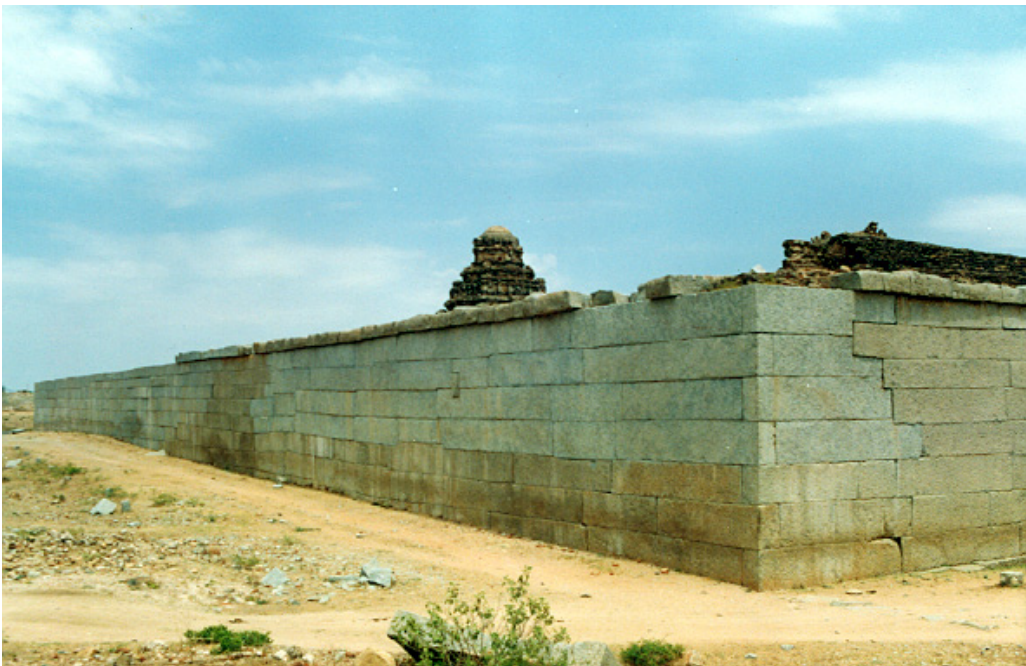
PLATE LII CHANDRASEKARA TEMPLE, ENCLOSURE WALL: AFTER CONSERVATION
