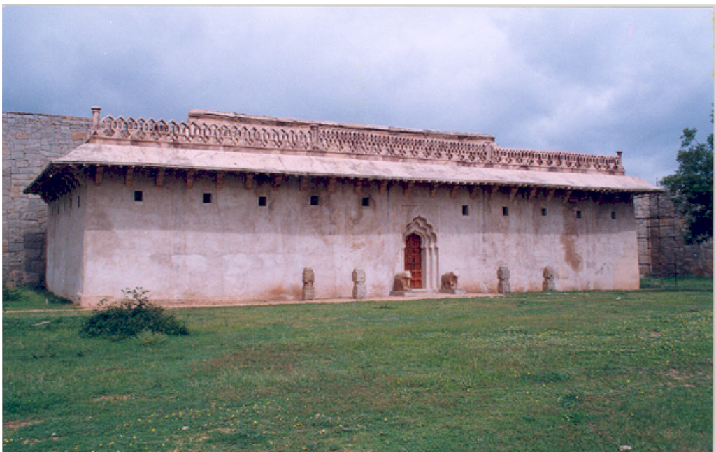
PLATE XXXIV ZANANA ENCLOSURE: TREASURY BUILDING
