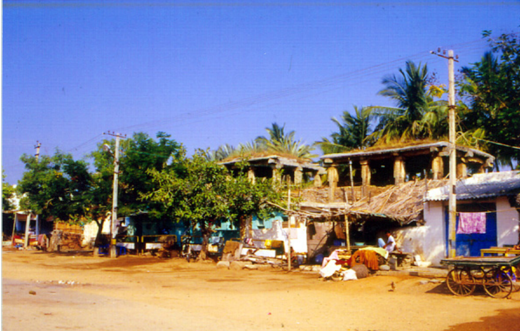
PLATE CV VIRUPAKSHA BAZAAR, MANTAPAS: ENCROACHMENTS
