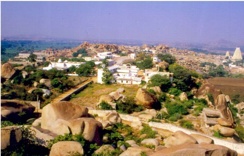
PLATE CVIII RATNAKUTA HILL: ENCROACHMENTS
