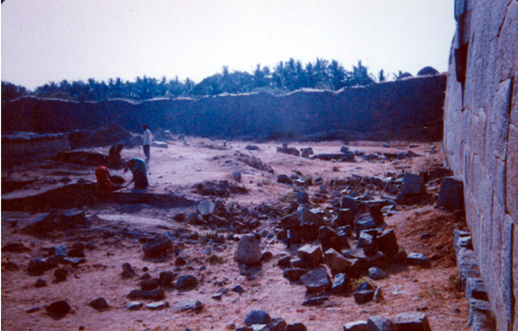
PLATE XCV HARIHARARAYA PALACE, ROYAL GARDEN: BEFORE EXCAVATION
