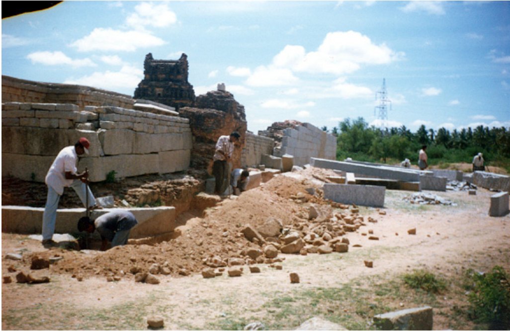
PLATE LI CHANDRASEKARA TEMPLE, ENCLOSURE WALL: DURING CONSERVATION
