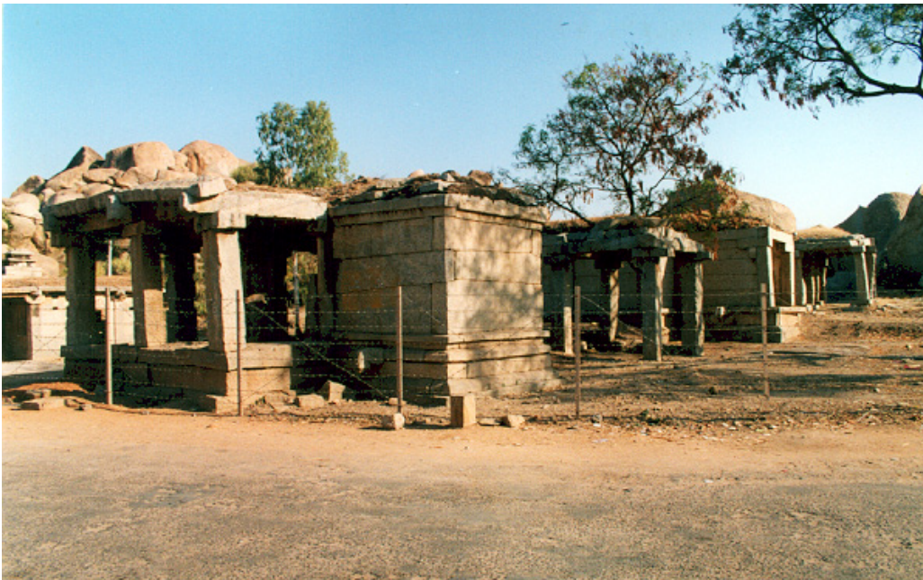
PLATE CXIV ROAD LEADING TO HAMPI: AFTER REMOVAL OF ENCROACHMENTS
