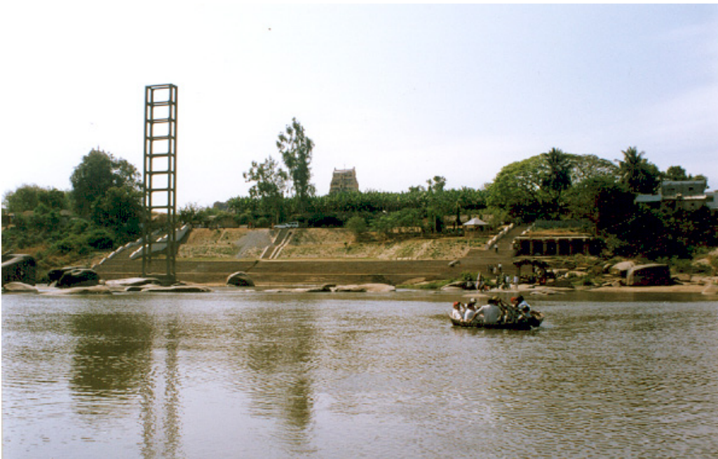
PLATE CXXIV SUSPENSION BRIDGE ACROSS TUNGABADHRA NEAR VIRUPAKSHA TEMPLE
