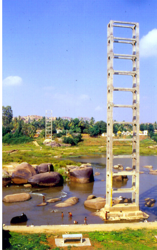
PLATE CXXV SUSPENSION BRIDGE ACROSS TUNGABADHARA NEAR VIRUPAKSHA TEMPLE
