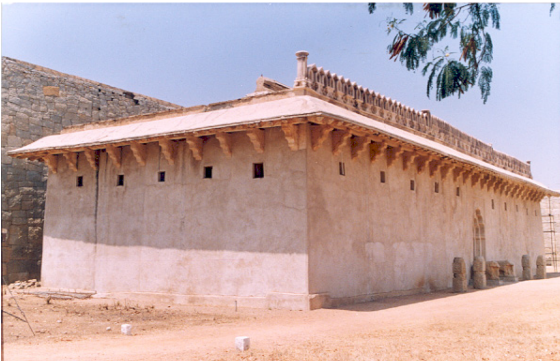
PLATE LVIII ZANANA ENCLOSURE, TREASURY BUILDING: AFTER CONSERVATION
