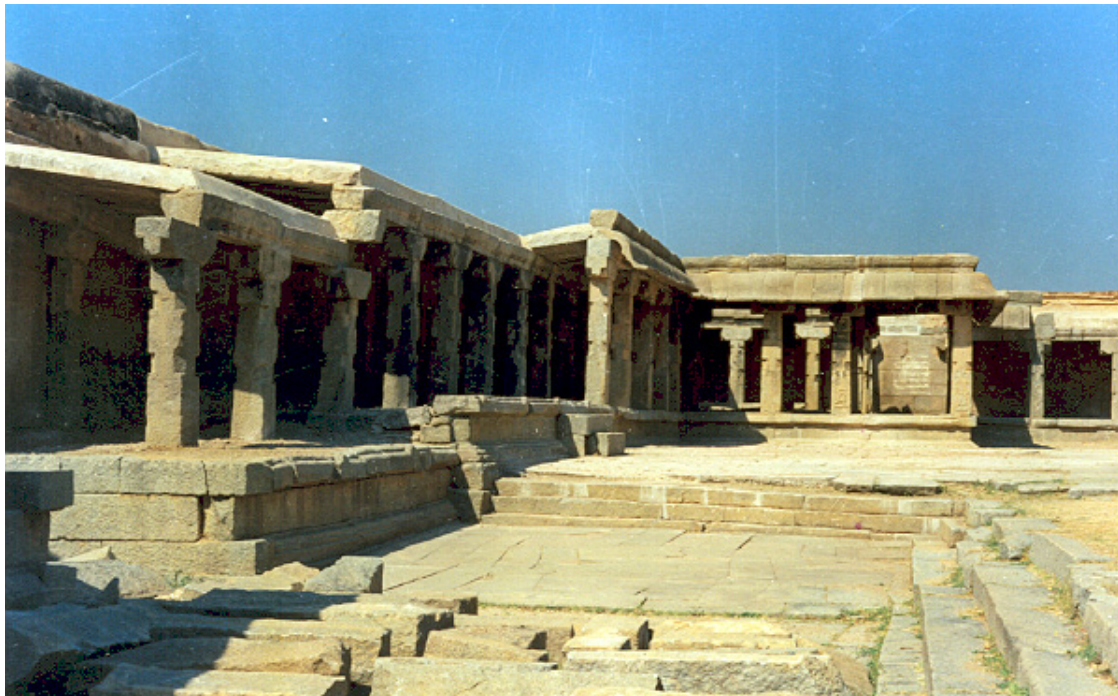
PLATE LXVI KRISHNA TEMPLE, CLOISTERED MANTAPA AND FLOORING: AFTER CONSERVATION
