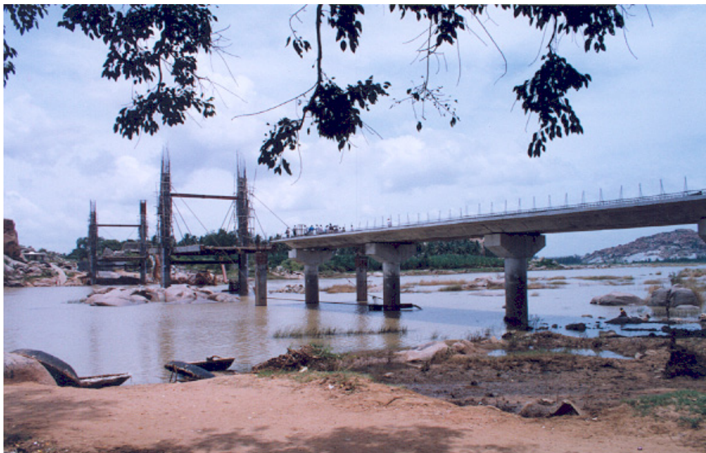
PLATE CXXVI BRIDGE ACROSS TUNGABADHARA NEAR TALARIGHATTA GATE
