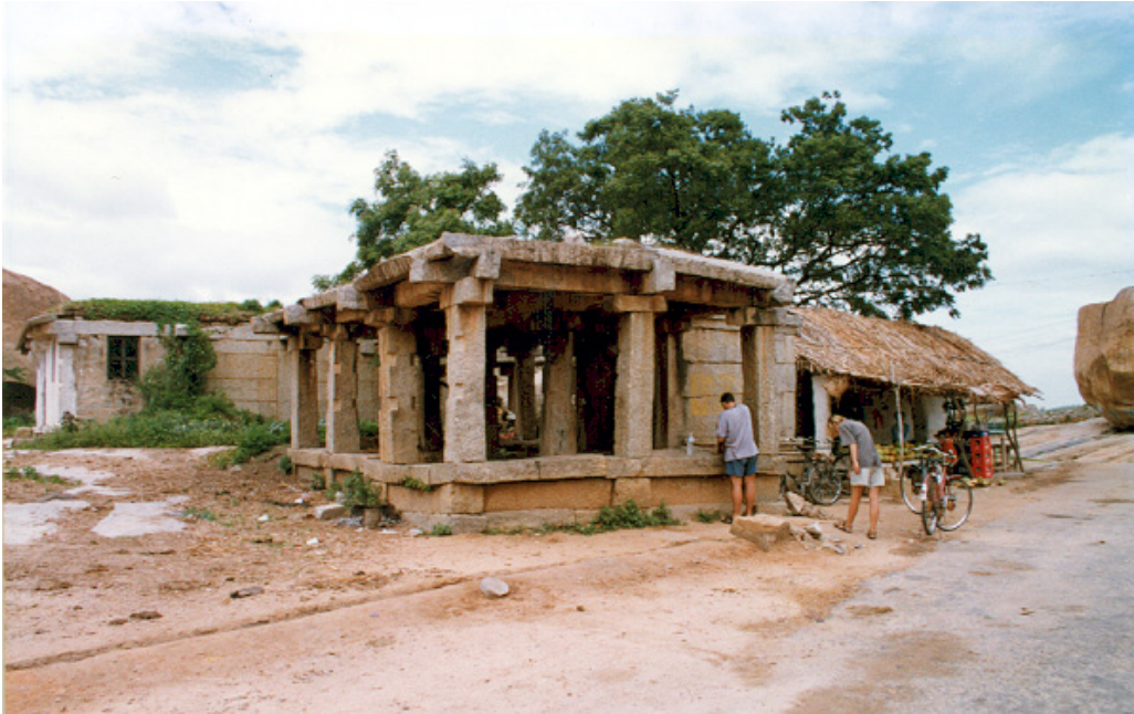
PLATE CXIII ROAD LEADING TO HAMPI: ENCROACHMENTS
