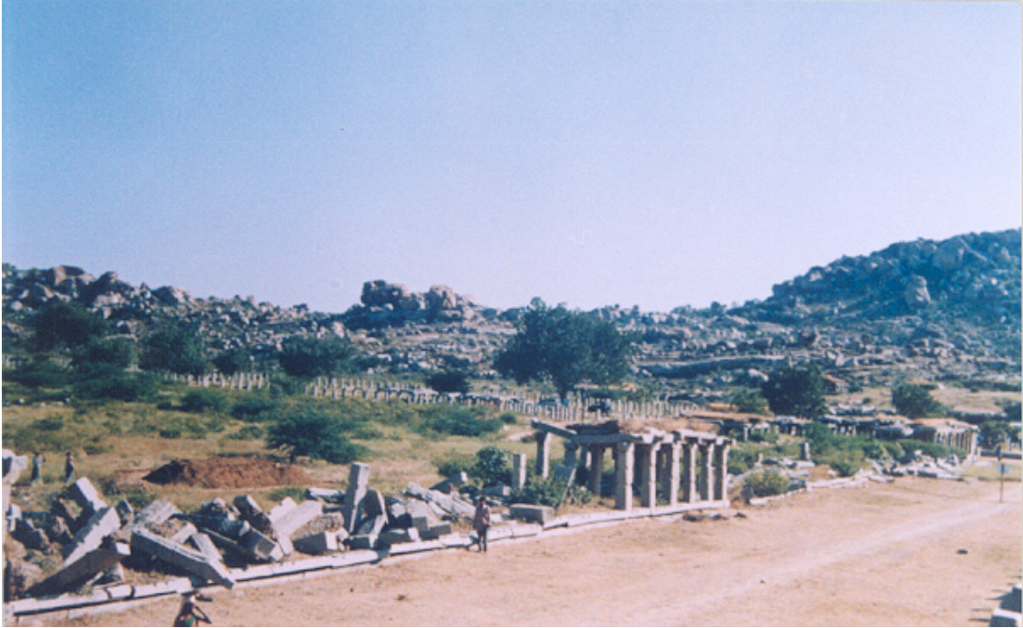
PLATE LXXXIII SIVA TEMPLE, BAZAAR: BEFORE CONSERVATION
