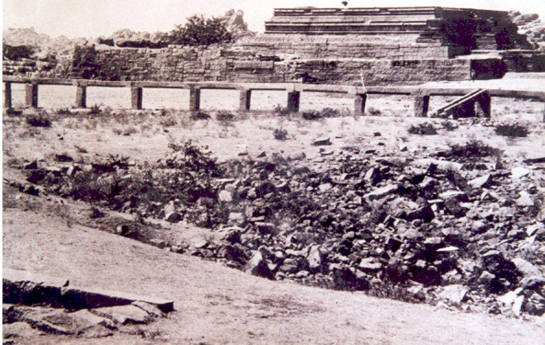
PLATE LXXXVII ROYAL ENCLOSURE, STEPPED TANK: BEFORE EXCAVATION
