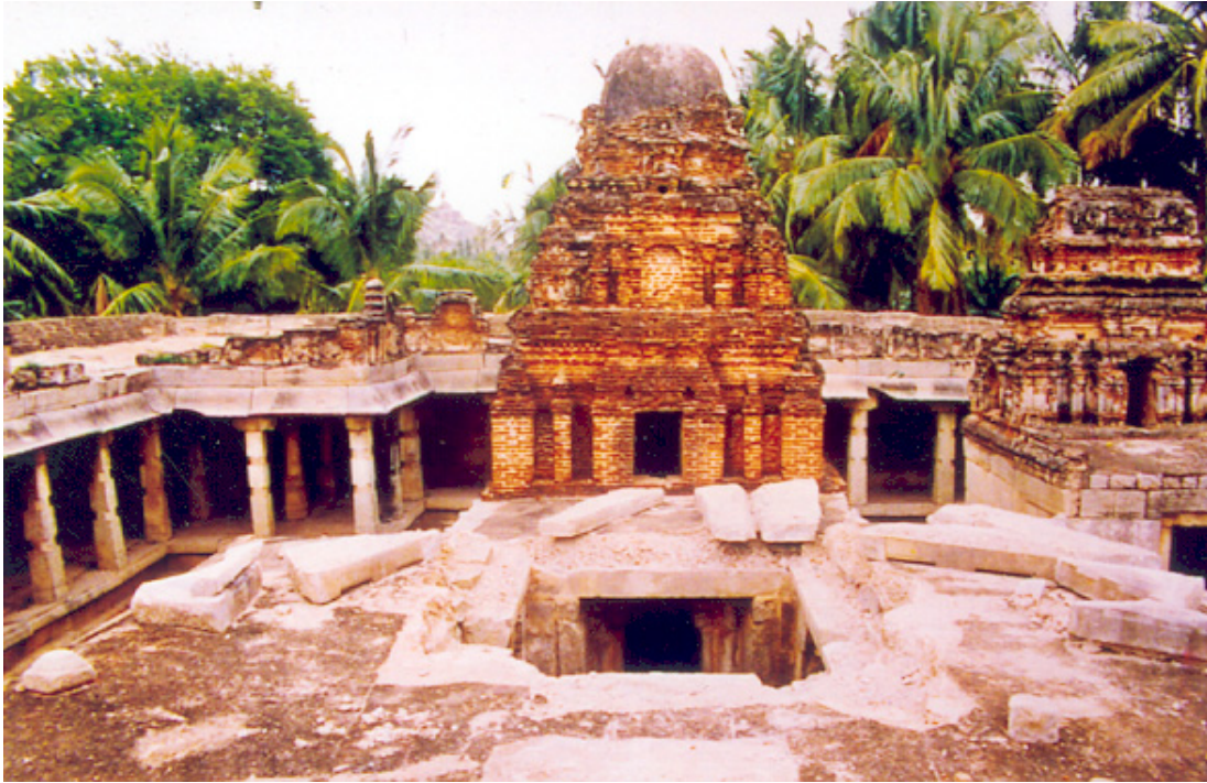
PLATE LXI CHANDIKESVARA TEMPLE, ROOF: BEFORE CONSERVATION
