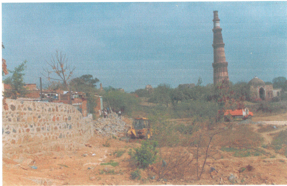
ENCROACHMENTS, ILLEGAL CONSTRUCTIONS IN THE BUFFER ZONE
