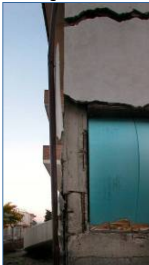
Fig. 48 & 49 Interior and exterior of a damage reinforced concrete building in San Giuliano di Puglia after the Molise earthquake illustrating that the frame is on the verge of collapse. While this building will be difficult or impossible to repair to an earthquake-safe condition, the traditional house in Orta in Figure 46, with a similar amount of debris on the floor has lost a negligible amount of its total capacity, and can be easily repaired.
