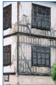
Fig. 42 Large 3 story house in himiş construction, Safranbolu, Turkey, 2000. Safranbolu is now on the World Heritage List because of its unique collection of intact Turkish vernacular houses.
