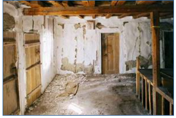
Fig. 45 RIGHT: Interior of himiş house after the Orta earthquake showing the “working” of the masonry panels. This view shows the inherent flexibility of the structures, but the inevitable disruption of the mud and lime plaster leads people, including both the owners and the government inspectors to assume that the buildings has lost strength when it has not.
