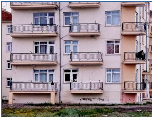
Fig. 50 LEFT: RC apartment building in Orta after 2000 earthquake shows cracking in the infill walls.
