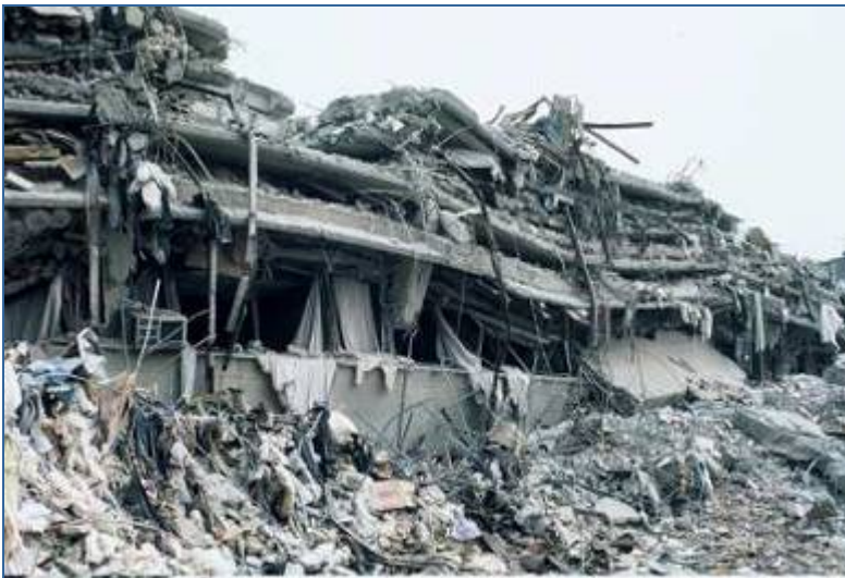
Fig. 19: “Pancake” collapse in Mexico City, 1985.
