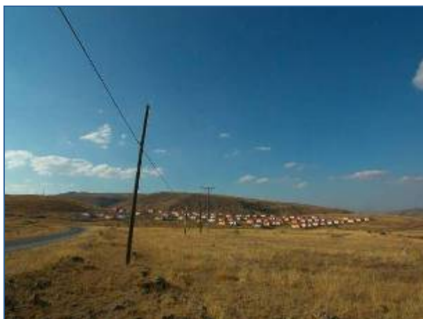
Fig. 54 Elden New Village, a government constructed re-location settlement of 87 houses.
