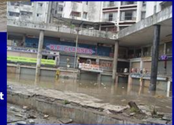
Floods in Surat, Gujarat August 2006
