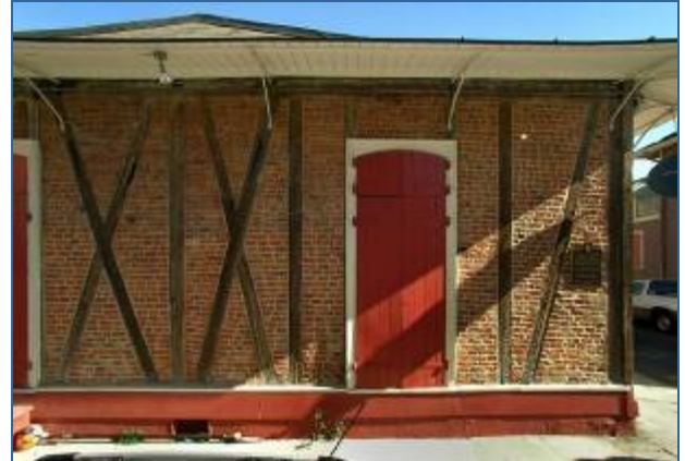
Fig. 17: Colomage construction in the French Quarter of New Orleans, 2006.
