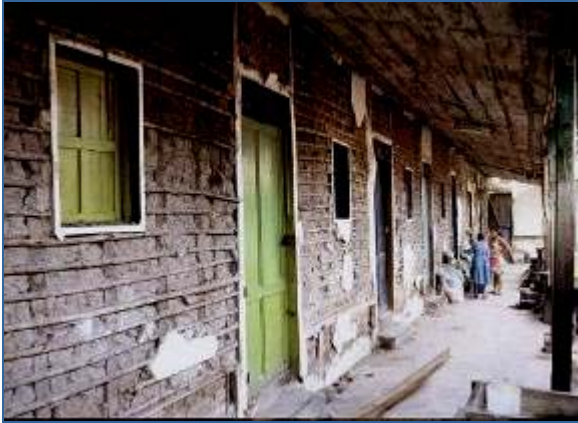
Fig. 16: Bahareque construction in San Salvador showing effects of 1986 earthquake. The loss of the stucco shows that the wall underwent deformations without loss of its underlying structural integrity.
