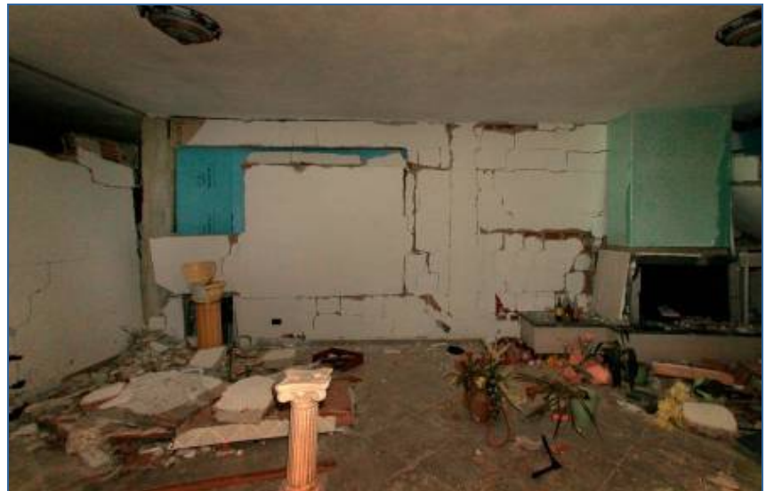
Fig. 48 & 49 Interior and exterior of a damage reinforced concrete building in San Giuliano di Puglia after the Molise earthquake illustrating that the frame is on the verge of collapse. While this building will be difficult or impossible to repair to an earthquake-safe condition, the traditional house in Orta in Figure 46, with a similar amount of debris on the floor has lost a negligible amount of its total capacity, and can be easily repaired.
