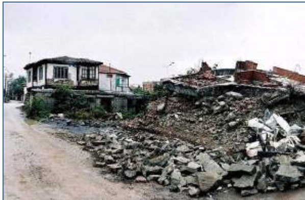
Fig. 3 Surviving hımış house next to a row of collapsed reinforced concrete buildings, Adapazari, Turkey, 1999.
