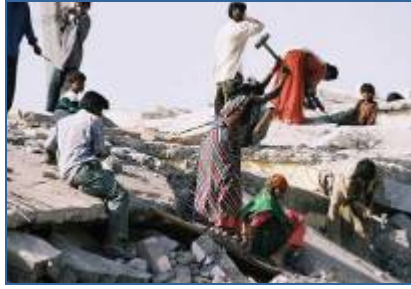
Fig. 4 Demolition workers on collapsed RC infill building in Bhuj, 2001 one month after the Gujarat Earthquake. Women work alongside men in heavy construction tasks in India.
