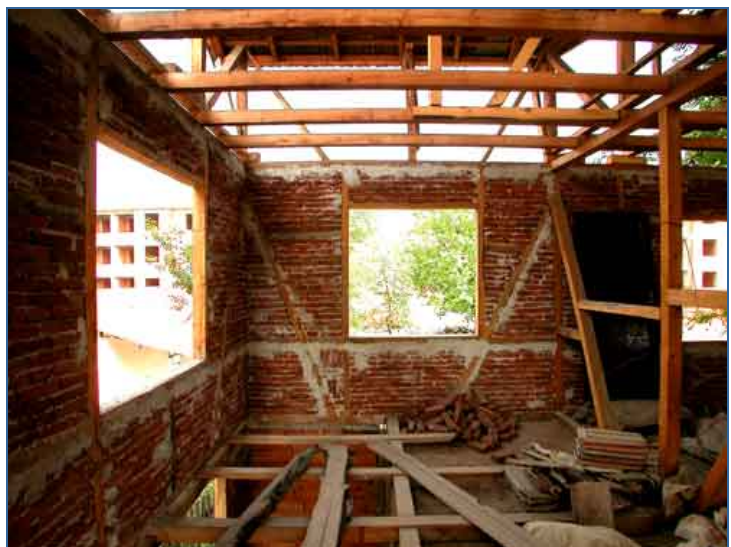
Fig. 65 & 66 After witnessing the destruction of RC buildings in Duzce while his father's hımış house survived undamaged, this resident of Düzce decided to stop construction of a new RC house and change it to hımış construction.
