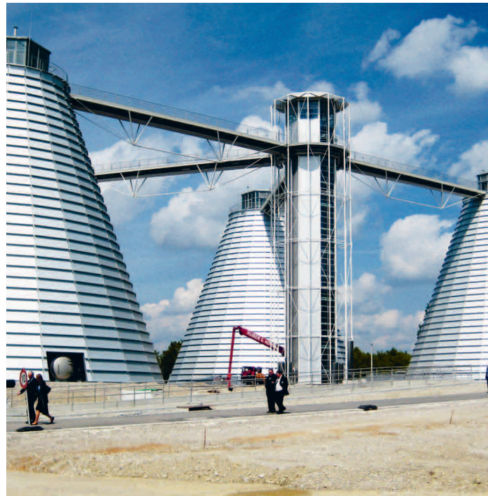
Wastewater treatment plant Munich, Germany 2010
