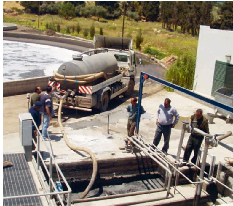
Wastewater treatment plant in Palestine, Ramallah 2005
