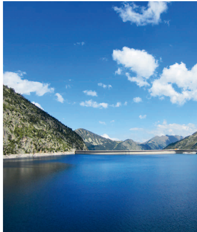
Reservoir in France 2012
