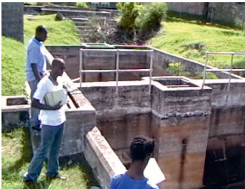
Students viewing a primary clarifier that has been emptied for renovations, Jamaica 2010
