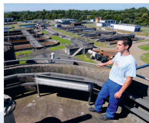
Municipal wastewater treatment plant in St. Augustin, Germany 2010
