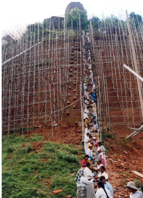
Restoration works at one of the stupas
