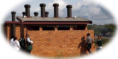
Water and sanitations facilities
