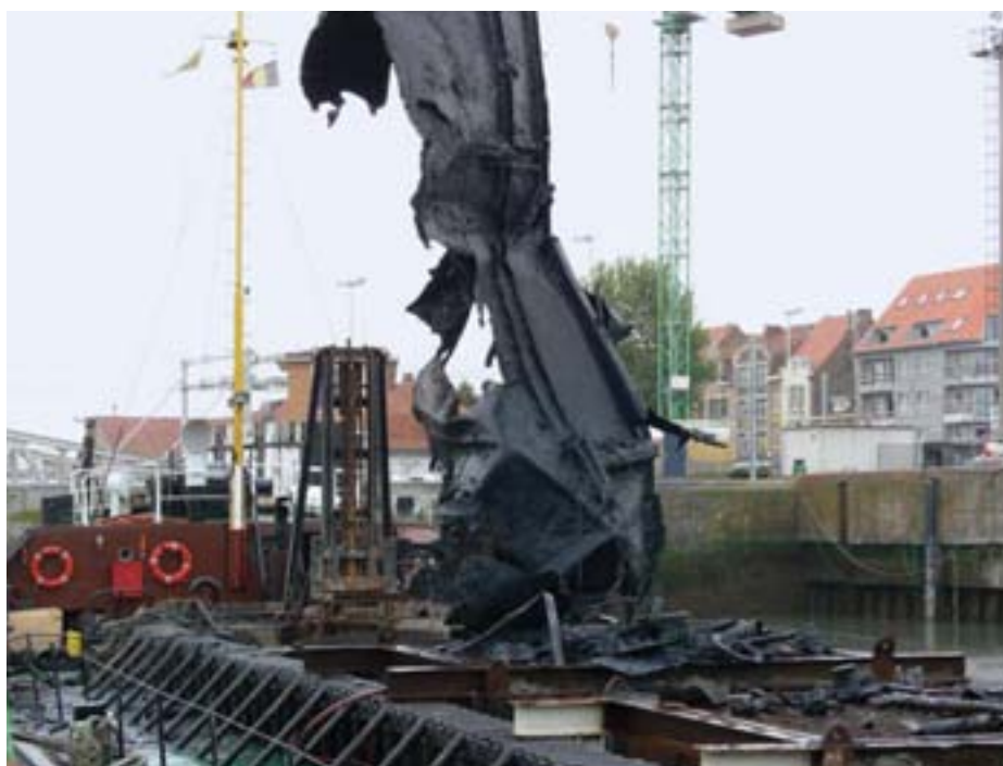
FIGURE 3 The VIOE was contacted by the Maritime Access Division for advice during the salvaging of a World War I wreck which was causing an obstruction in an inner harbour sluice in Zeebrugge. © VIOE
