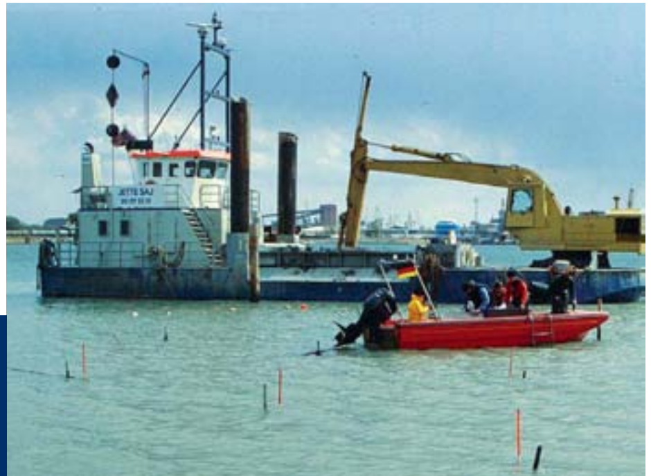
FIGURE 5 Infrastructural construction work and archaeology in Wismar Bay. During dredging work for a sport boat harbour a 15th century ship wreck was found and excavated by the Authority for Culture and Preservation of Monuments (Förster 2000). Picture: Landesamt für Kultur und Denkmalpflege, Archäologie und Denkmalpflege Schwerin.
