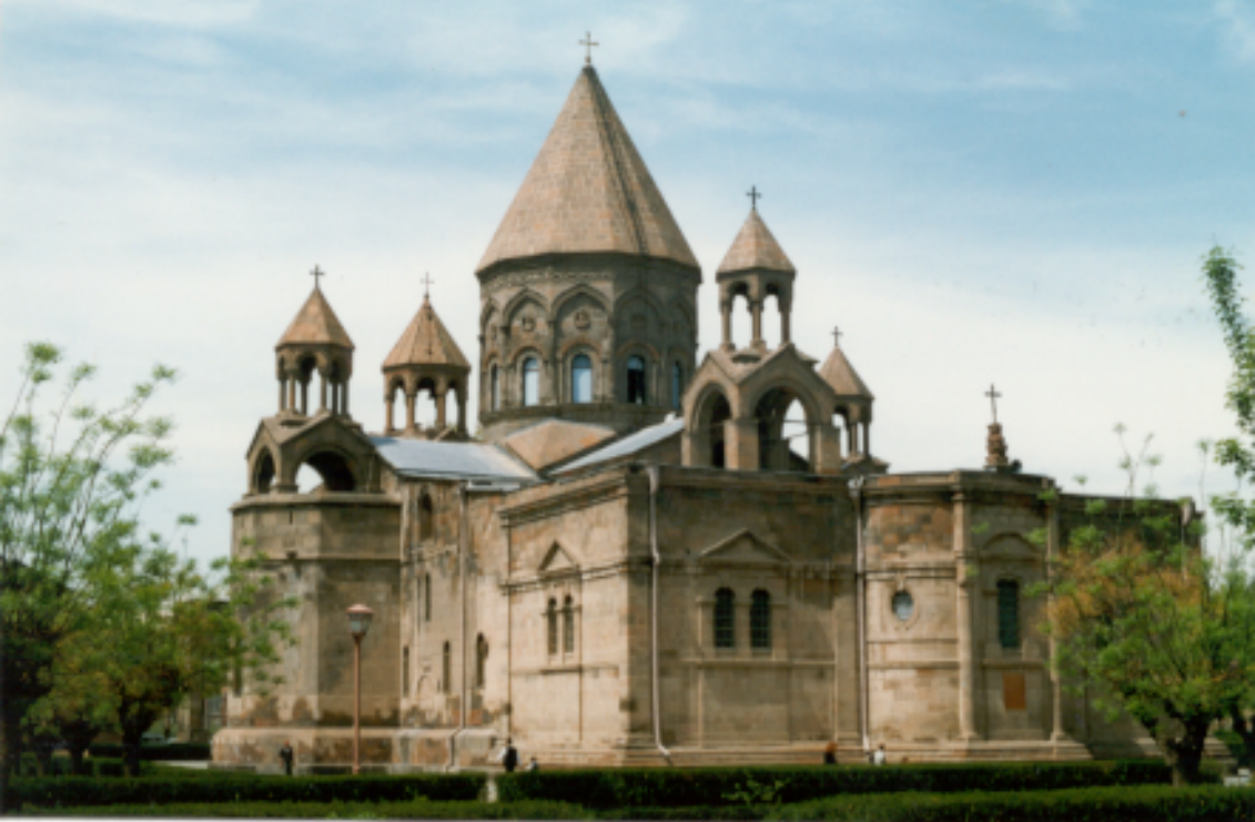
Pic. 2 Mother Cathedral, 303AD, view from South-East
