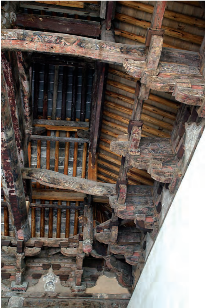
Photograph-6-10 Spar frame within Main Hall of Huishan Temple (III)
