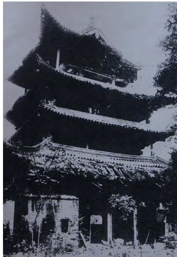
Photograph-5-10 Ancient photograph of Drum Tower of the Kernel Compound of Shaolin Temple
