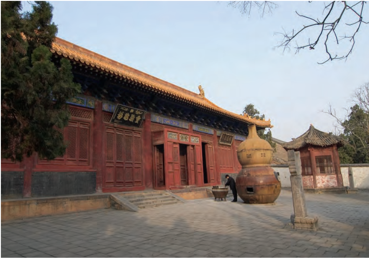
Photograph-1-17 Resting Hall of Zhongyue Temple
