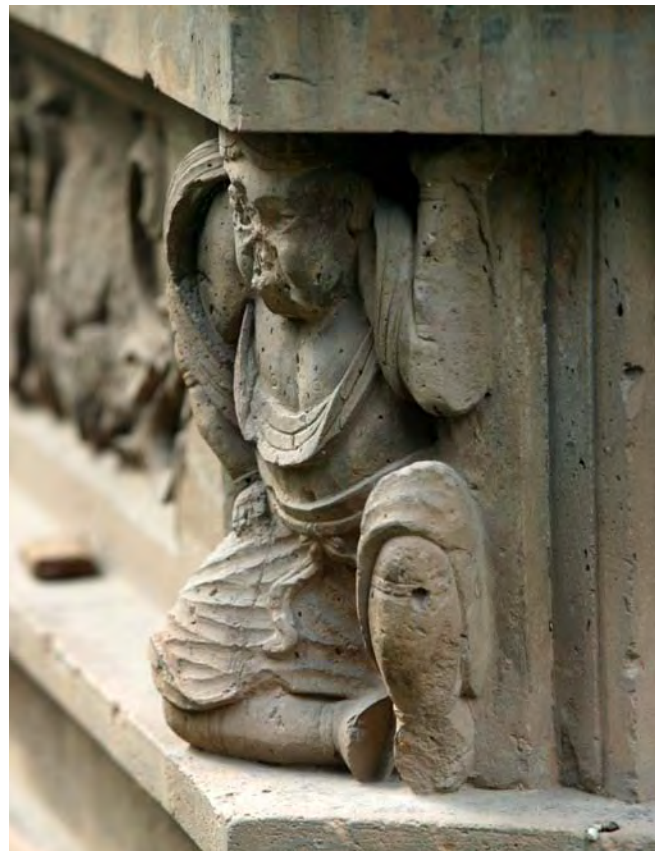
Photograph-5-58 Detail of Pagoda of Yugong ( II )
