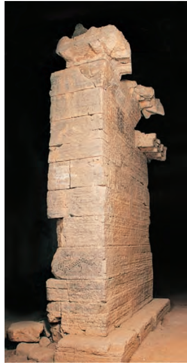
Photograph-2-2 West Structure of Shaoshi Que Gates
