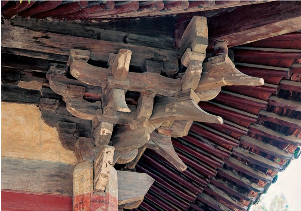
Photograph-5-32 Bracket set on Main Hall of Chuzu Temple of Shaolin Temple ( II )
