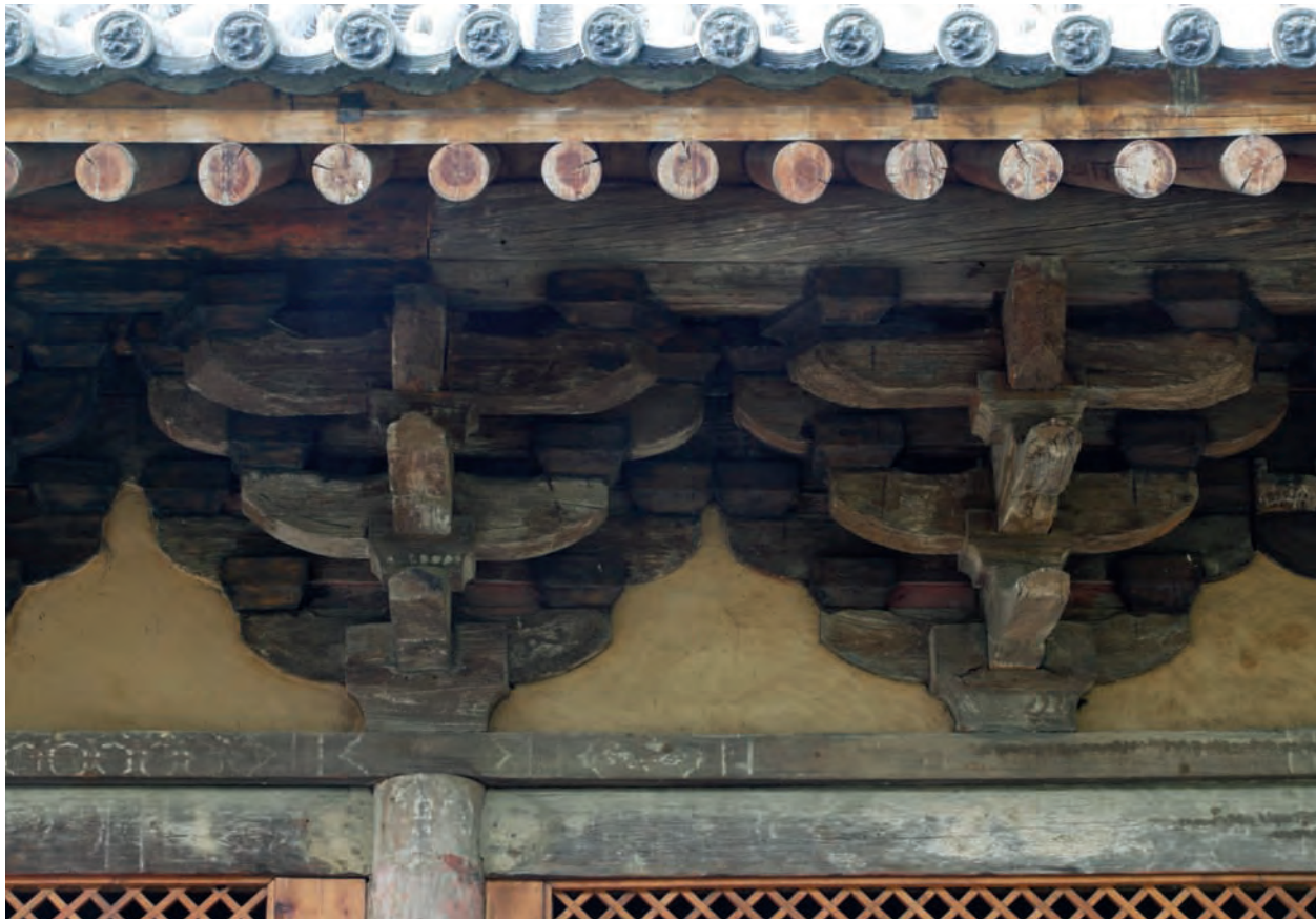
Photograph-6-6 Bracket set on column and capital of Main Hall of Huishan Temple
