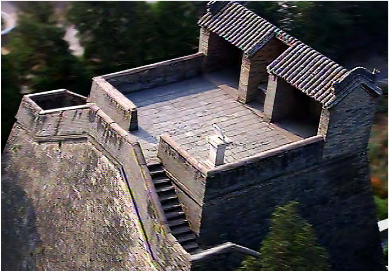
Photograph-8-3 East and west rooms on the top of Observatory
