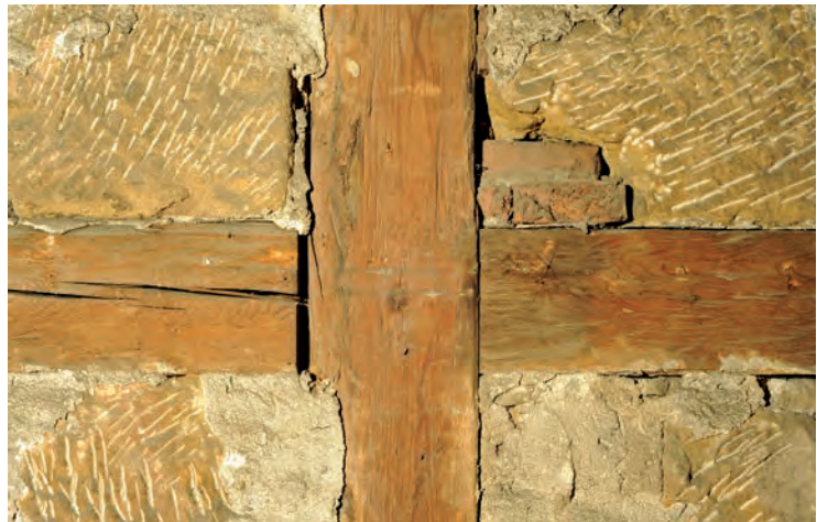
75_Detail of intersecting half-timbered beams
