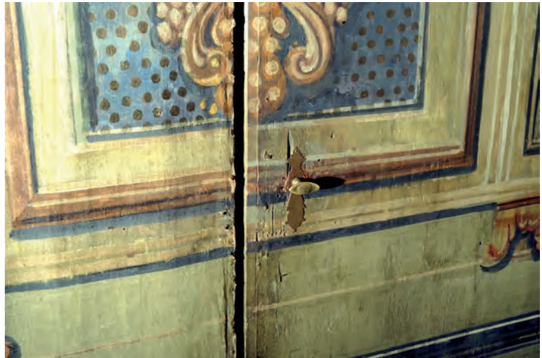
70_Access door to the first tier
