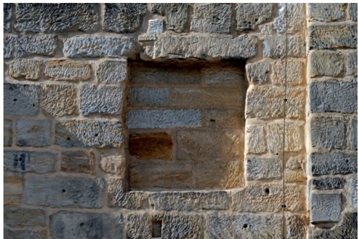
14_Detail of blocked up wall opening
