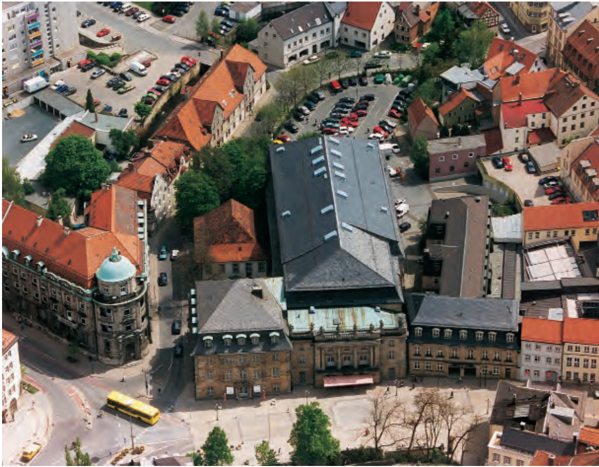
01_Aerial photograph of the Margravial Opera House with adjacent Redoutenhaus as seen from the west
