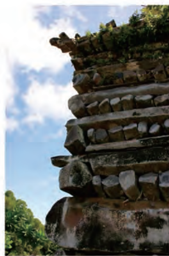
Photo 13 Northeast corner of the outer wall
