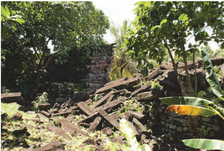
Photo 17 Collapse of the north perimeter wall seen from the inside
