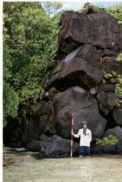
Photo 26 Stonework in the southwest corner of Pahnwi
