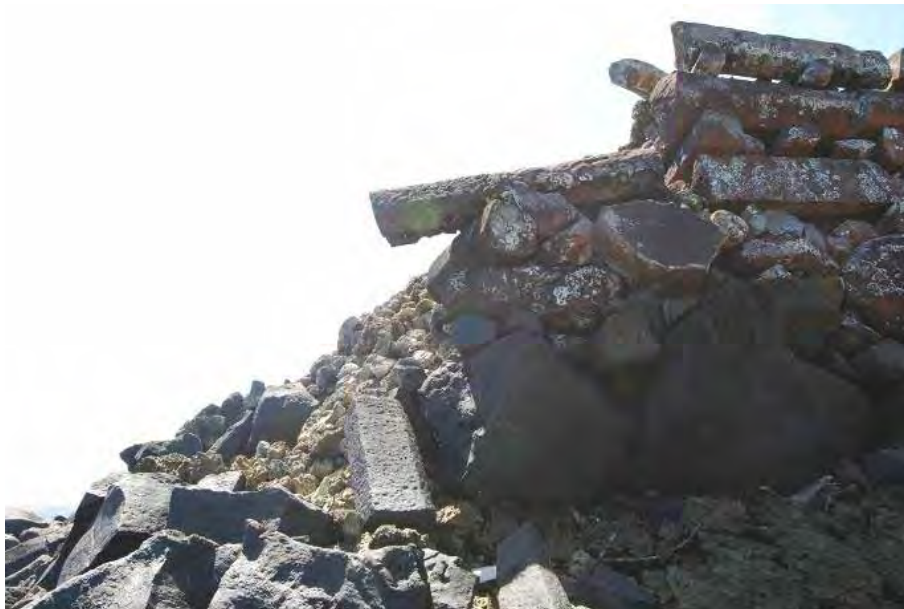
Figure 6.1. Example of collapse of a basalt structure in Nan Madol.
