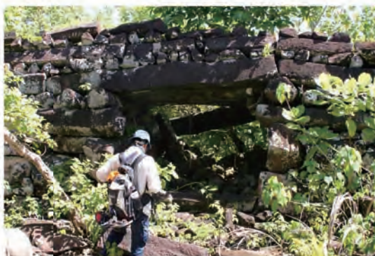
Photo 21 Collapse of the ceiling above the entrance in the enclosure around the burial ground
