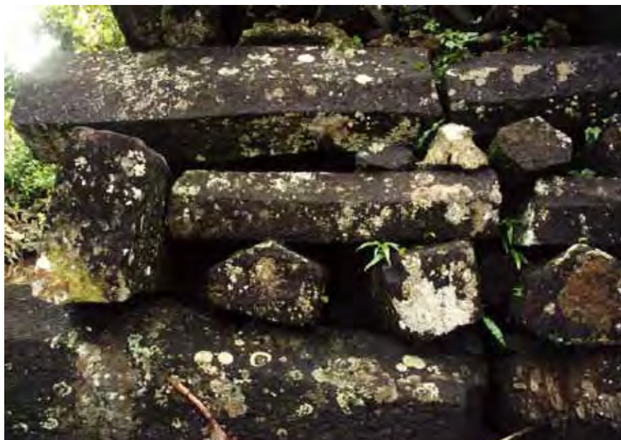
Figure 2.5. Lelu, header-stretcher detail of Foton compound corner.
