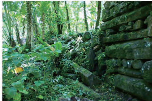
Photo 3 Collapse of the northeast outer wall
