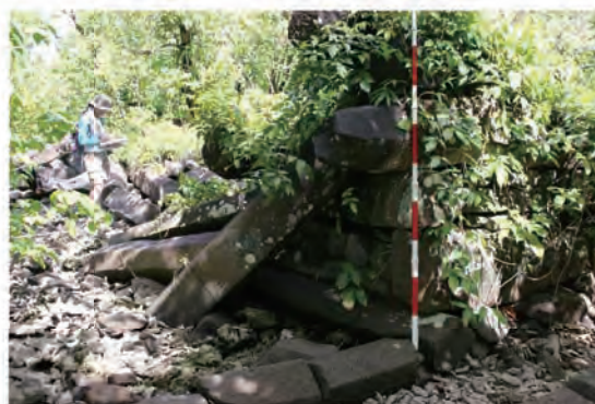
Photo 23 Collapse of the southwest corner of the perimeter wall and lush vegetation on Idehd
