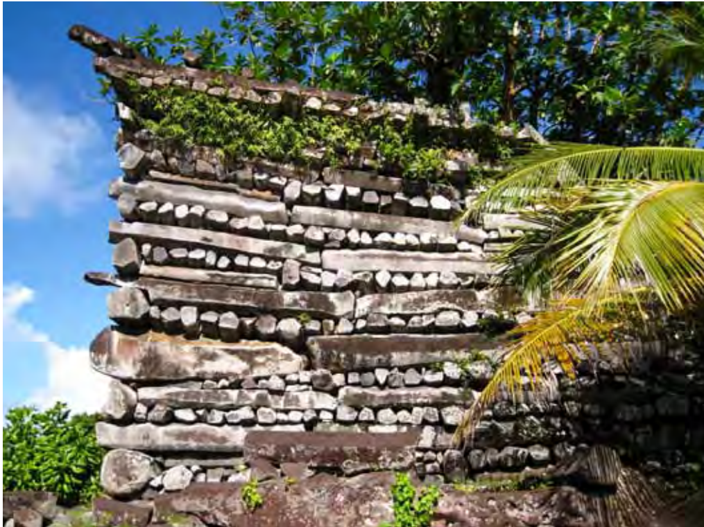
Figure 2.7. Columnar basalt used in a wall built by in a header-stretcher technique Nandowas Islet (#113) (Photo by Takuya Nagaoka, 2012).
