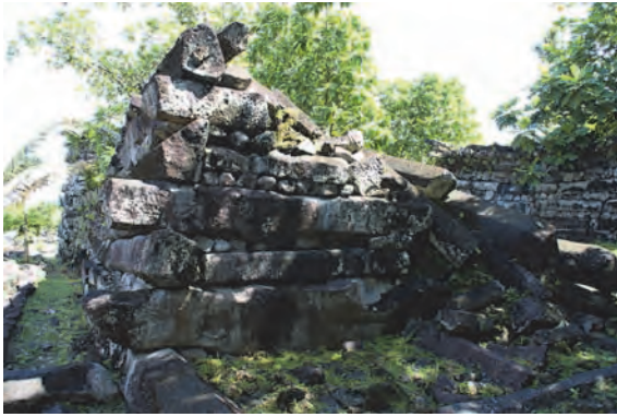
Photo 15 Collapse of the perimeter wall on the north side of the entrance
