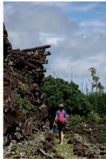
Photo 14 Southeast corner of the outer wall
