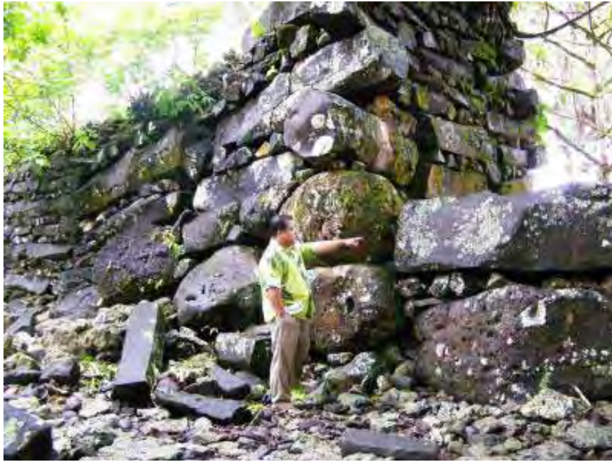
Figure 2.10. Lelu, wall of Kinyeir Fulat showing header-stretcher pattern of columnar basalt lengths
