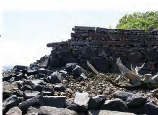
Photo 20 Southeast corner of the perimeter wall
