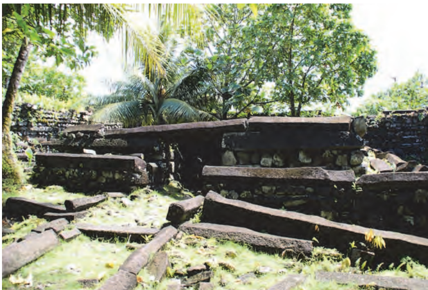
Photo 19 Collapse of the basalt column around the opening of the central stone chamber
