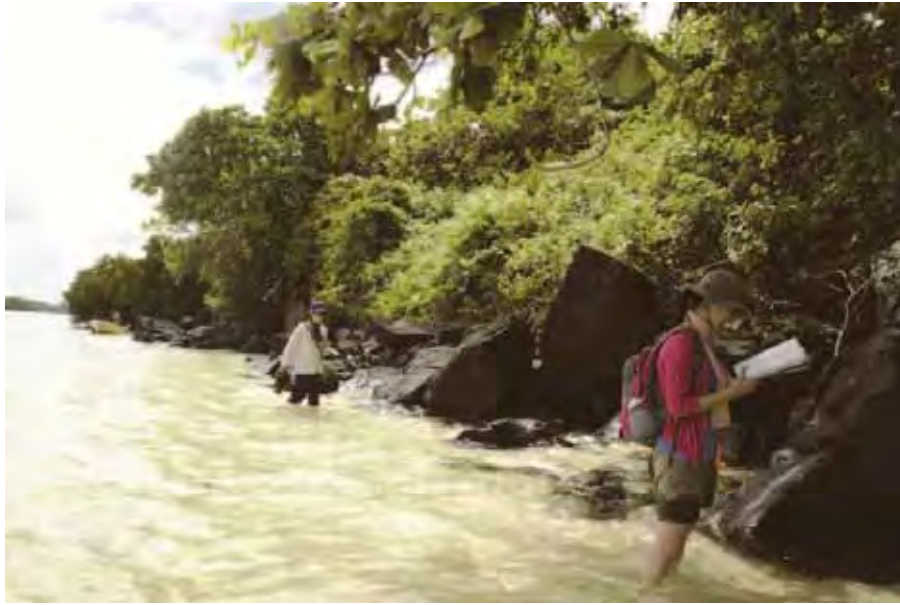
Figure 4.7. Collapse of the stone wall and the sedimentation of sand (Kataoka et al. 2012:25, Photo 28).
