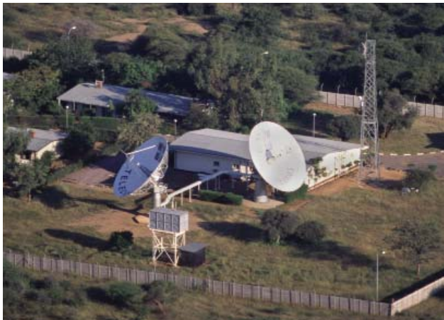
Botswana has a sound telecommunications infrastructure
