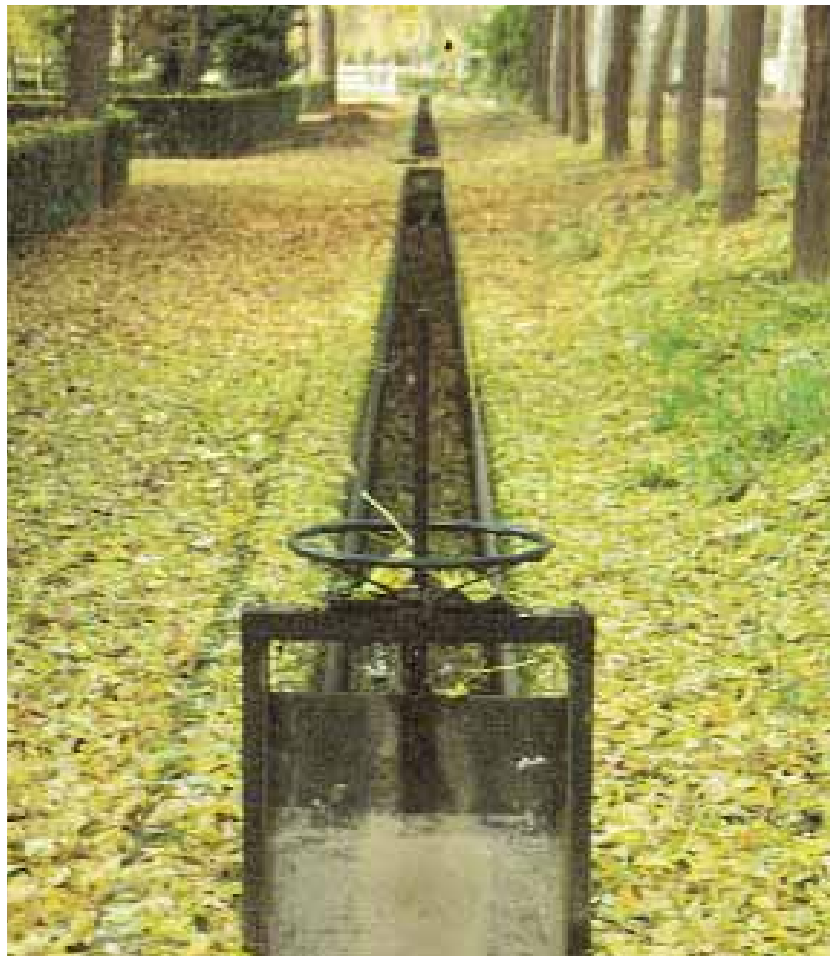
Bautista de Toledo. This project considered the need to filter water into the man-made river that separated Raso de la Estrella from the Jardín de la Isla, protecting the garden from flooding. The dam was also used for a mill that obtained the energy from the waterfall.
