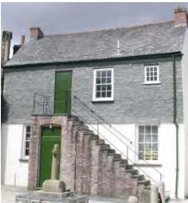
Murdoch House (c1660, Listed Grade II*). Mining engineer William Murdoch (1754-1839) lived here whilst he worked on local mines as an engine erector for Boulton & Watt of Birmingham. He made a small working model of the world's first steam locomotive in 1784 and also invented gas lighting in this house in 1792.
