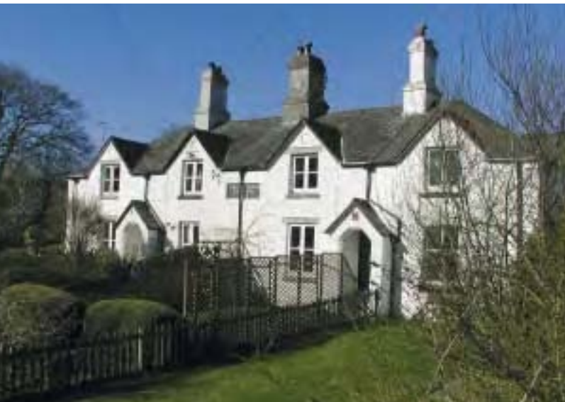
Bedford Cottages. Following the discovery, in 1844, of the immensely rich copper lode at Devon Great Consols, there was a large influx of workers to the Tavistock district. In response to a serious shortage of housing and gross overcrowding (which became a local scandal) 268 'model' industrial workers' cottages were built in and around Tavistock (between 1845 and 1866) by Francis the 7 th Duke of Bedford.
