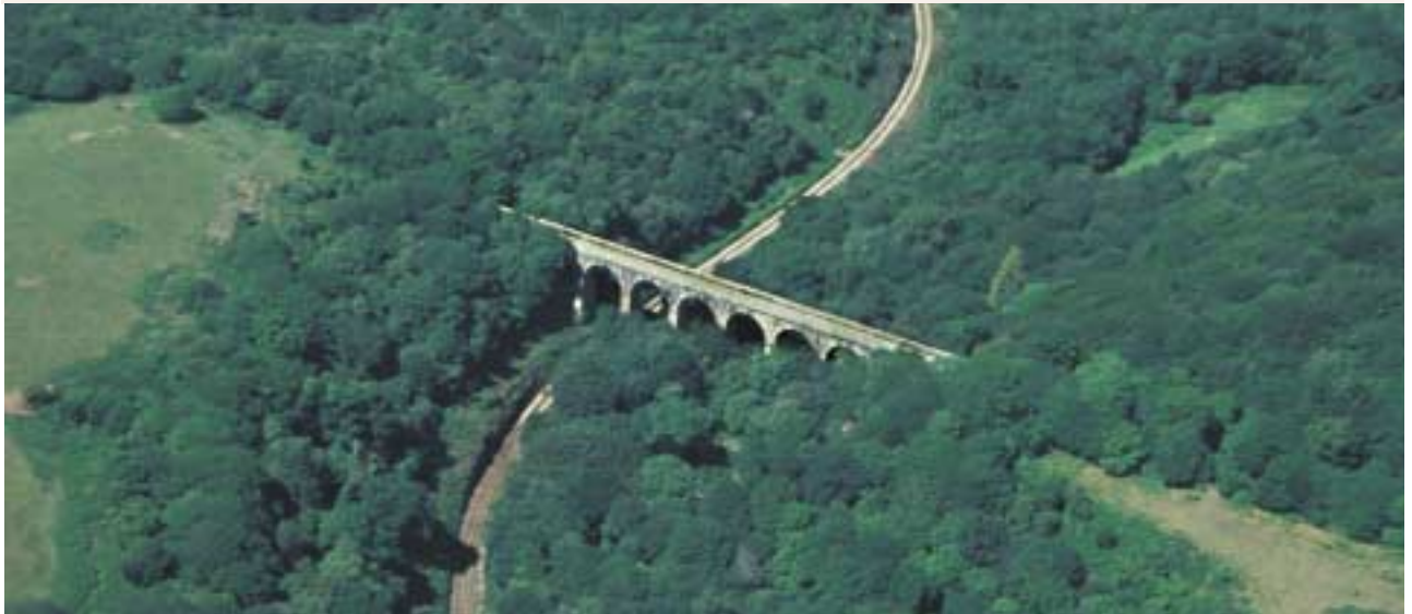
Treffry Viaduct & Aqueduct (1842, Scheduled Monument). This is the earliest granite construction of its kind in the region and stands 27m over the river with a span of 200m.
