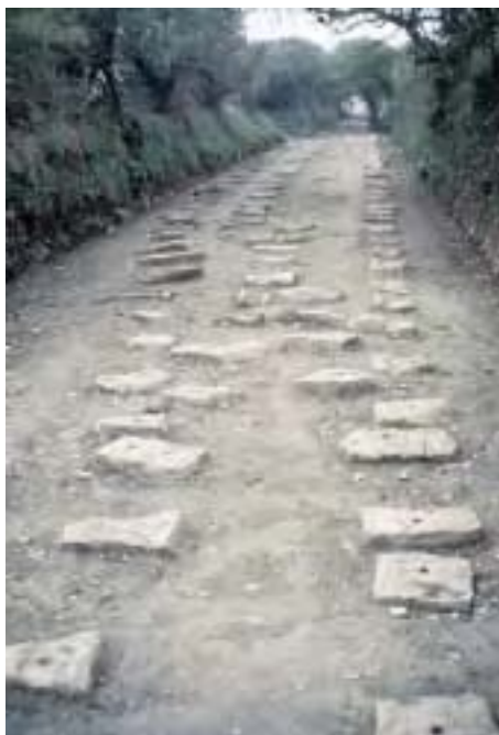
The Poldice Plateway following works to enable it's use as part of the Mineral Tramways Trail network.
