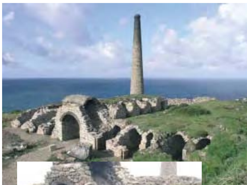
The Brunton arsenic calciner with its associated flues, condensing chambers and chimney at Botallack was built circa 1908. The site is designated a Scheduled Monument. Unfortunately the scrapping of its ironwork in 1914 started a chain of deterioration and in recent decades the flue and chamber roofs suffered progressive collapse and the site was included on English Heritage's Buildings At Risk Register in 2002 and 2003. The site was recently acquired by the National Trust. Funding was received from Objective 1 together with a grant from English Heritage to undertake extensive conservation works in 2004, project managed by Cornwall County Council. These works have enabled the site to be made safe and secure: over 175 tonnes of contaminated material (arsenic) have been removed from the site; its walls and roofs, together with the chimney have been stabilised by re-pointing and limited rebuilding, whilst the interpretation of the site has been greatly enhanced through the full reconstruction of a pair of the condensing chambers. As a result the site is no longer 'at risk'.
