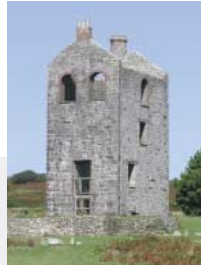
South Phoenix Mine (Listed Grade II). Houseman's engine house was once converted into a mine office.
