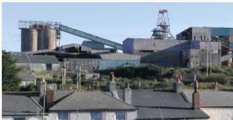
South Crofty Mine (A5). New Cook's Kitchen Shaft headgear and mill.
