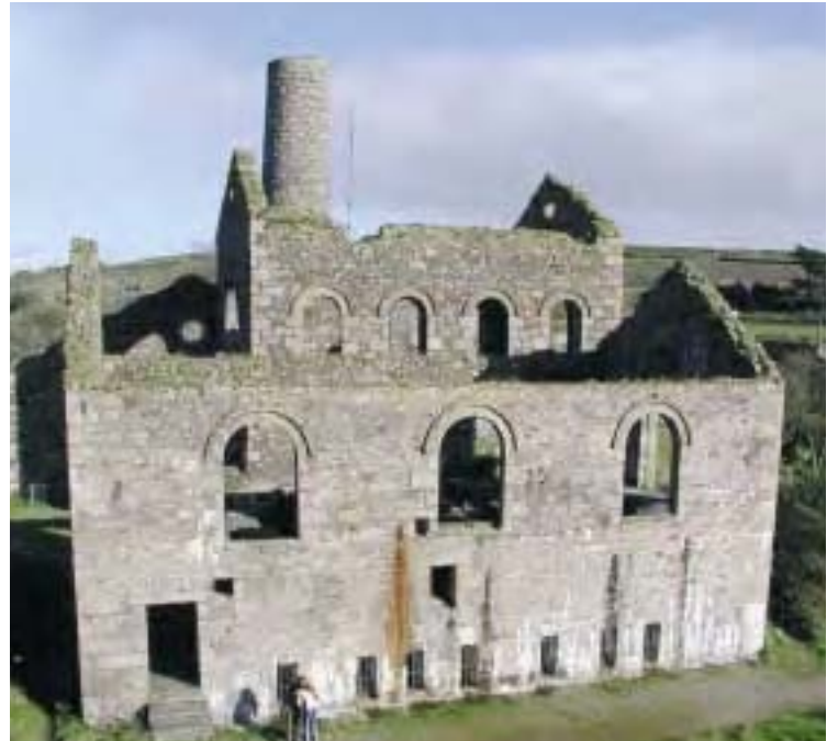
Basset Mines, Marriott's Shaft complex (1900, Scheduled Monument, Listed Grade II).
