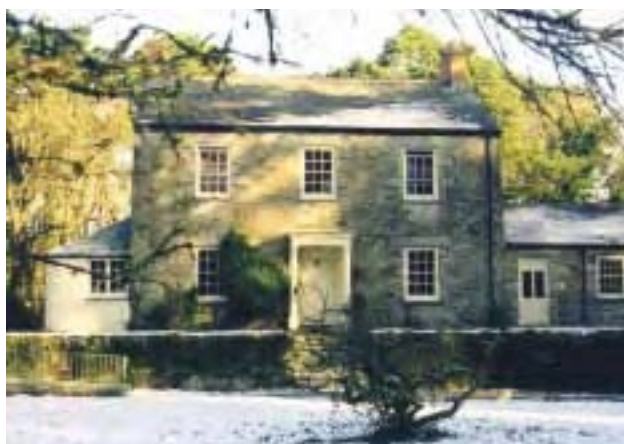
Godolphin Mine Count House (Listed Grade II). This serves as a Warden's base and an education centre for the National Trust.
