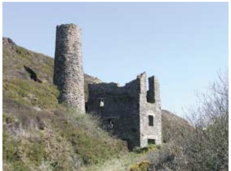
Tywarnhayle Mine, (1826, Listed Grade II)
