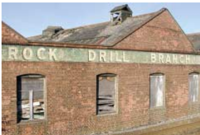
Holman Brothers Rock Drill Works (late-nineteenth century).
