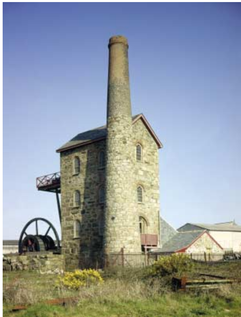
East Pool Mine (A5, 1887, Listed Grade II*). The North Whim at Mitchell's Shaft was designed by Francis Michell of Redruth and made by Holman Brothers of Camborne in 1887. It was the last traditional Cornish beam whim to be built and is now preserved by the National Trust.
