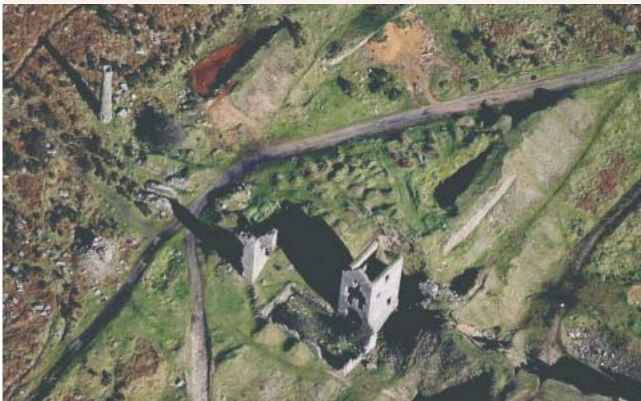
South Caradon Mine (Scheduled Monument). The remains of two pumping engine houses, side-by-side, represent an unusual example within the nominated Site.
