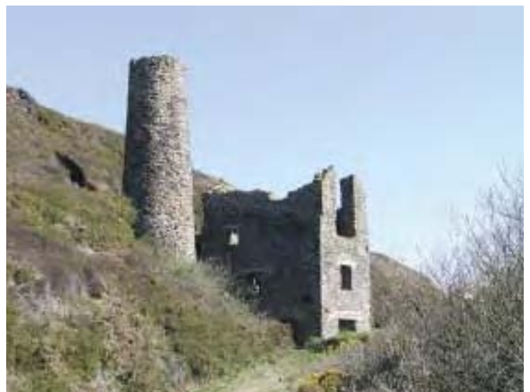
Tywarnhayle Mine, (1826, Listed Grade II)
