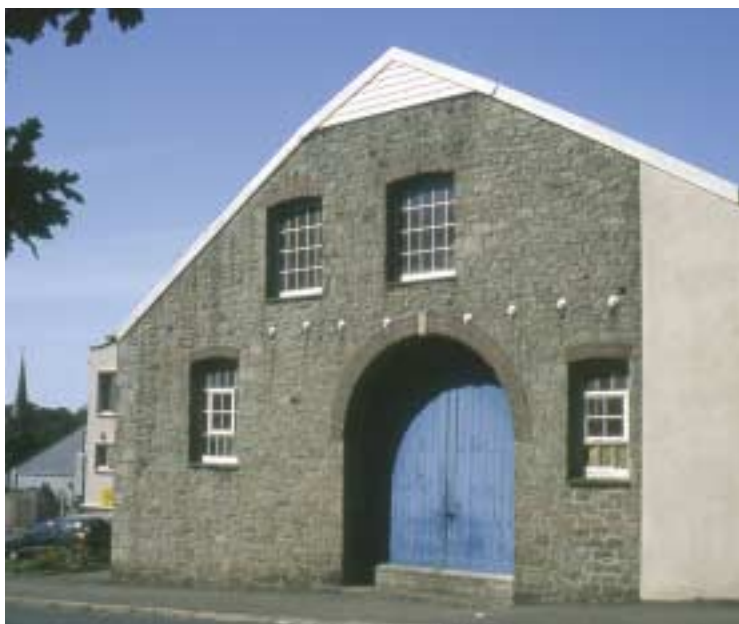
Charlestown Foundry established by J & R Michell in 1827. By the 1850s it was producing complete engines. The foundry had the distinction of casting the last pumping engine to be made in Cornwall in 1911.
