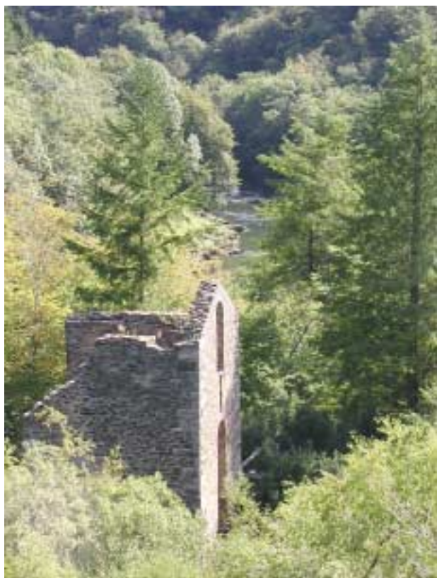
Gunnislake Clitters Mine (Scheduled Monument, Listed Grade II). Some mines are located in the Tamar Valley itself and here the topography imparts an unusual character, some having been worked beneath the river bed. This engine house pumped river water for dressing purposes.
