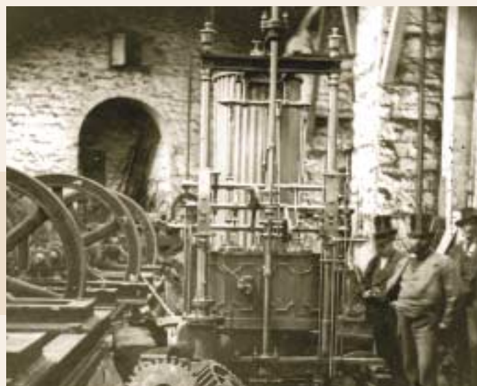
Harvey's Foundry Hayle (A2), 1876, where a blacksmith's workshop developed into the largest steam engine foundry in the world. Pictured in the 'erecting shop' this engine was supplied to the Kimberley Diamond Mines, South Africa.
