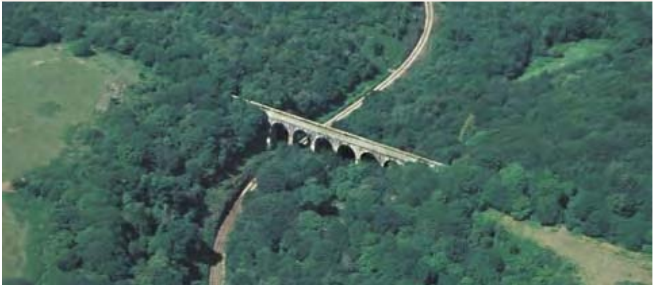
Treffry Viaduct & Aqueduct (1842, Scheduled Monument). This is the earliest granite construction of its kind in the region and stands 27m over the river with a span of 200m.
