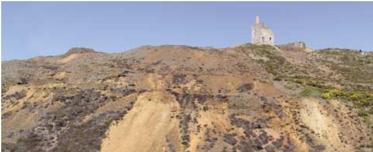
United Hills Mine, John's Shaft (1861, Listed Grade II) on the skyline above Tywarnhayle Valley.
