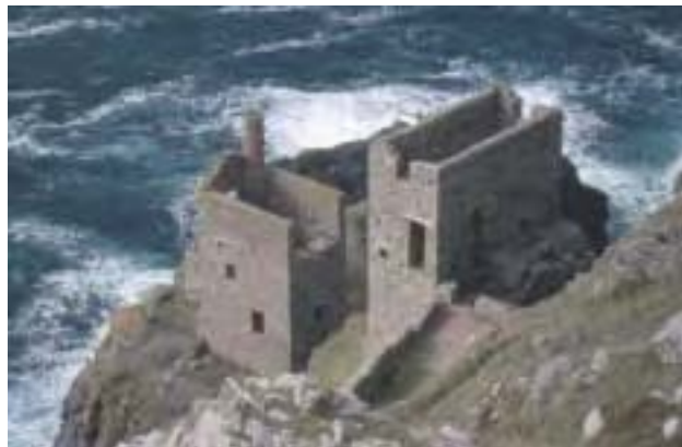
Botallack Mine, Crowns engine houses (lower pumping house 1835, higher whim house 1862, Listed Grade II).
