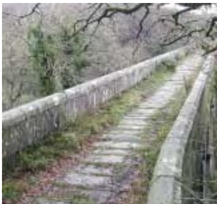
The granite sleepers of the 1835 industrial tramway also acted as lintels for the Carmears Leat that flowed immediately beneath.
