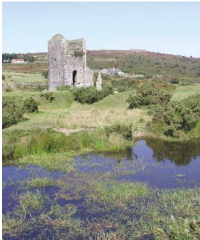
Wheal Jenkin (1886, Scheduled Monument, Listed Grade II), Bellingham's Shaft pumping engine house.
