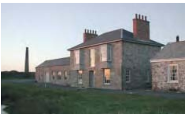
Botallack Mine, Count-house (Listed Grade II). A count-house ('account house') was the mine's office and they were the scene of customary count-house dinners for adventurers and mine management when the accounts were presented. Miners also received their pay from here.
