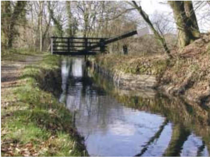
Lock gate, Tavistock Canal. To provide a current, the canal was to drop roughly one foot per mile .
