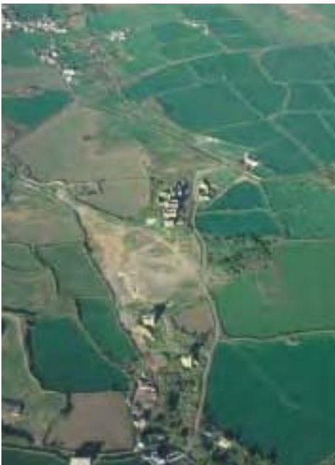
View along the surface of the Great Flat Lode (named for its unusually shallow inclination of around 45 degrees).
