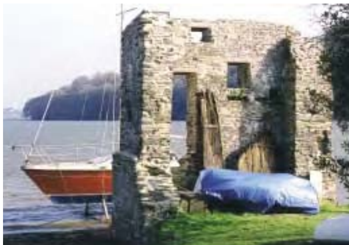
Carnon Stream Mine (1823, Listed Grade II). The remains of this creek-side engine house mark the unique Carnon Stream Mine that worked tin gravels in the river bed from shafts sunk within artificial islands out in the river itself.
