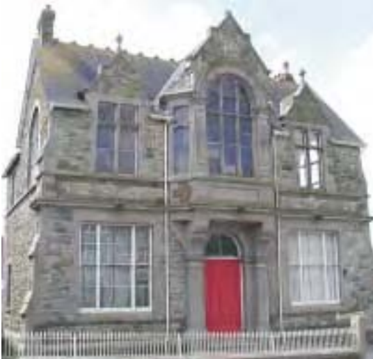
The School of Science & Art (1883) stands next to the Robert Hunt Museum (1890) in Clinton Road. It was built as a memorial to its founder by the Miners' Association of Devon and Cornwall. The Redruth School of Mines was based here and extra-mural classes continued until the 1950s.
