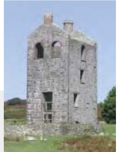
South Phoenix Mine (Listed Grade II). Houseman's engine house was once converted into a mine office.
