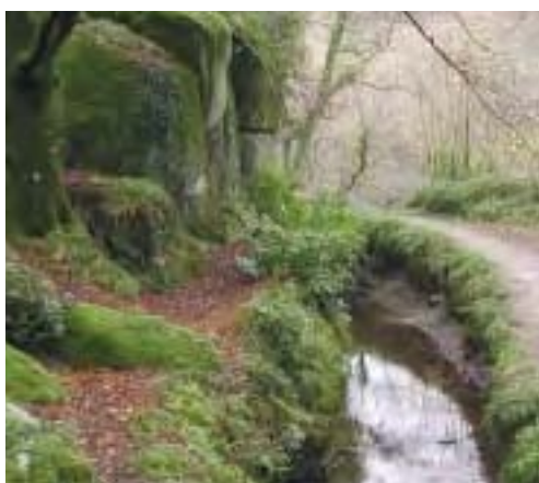
The Fowey Consols leat (1820s) is the earliest civil engineering construction built by Treffry in the Luxulyan Valley. It supplied the Fowey Consols waterwheels and the largest concentration of water power on a nineteenth century copper mine.
