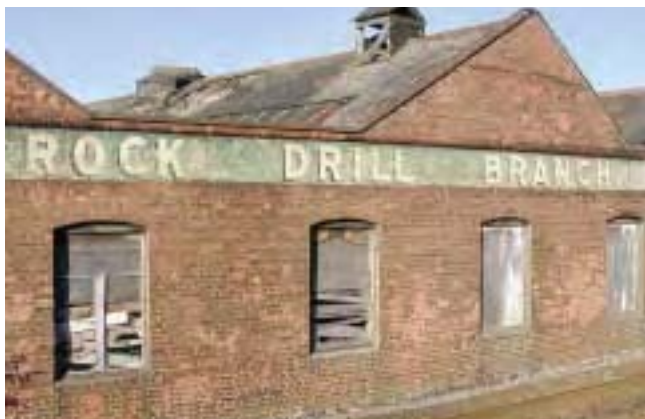
Holman Brothers Rock Drill Works (late-nineteenth century).
