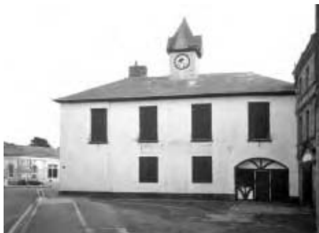
24 Foundry Square, Hayle, before renovation works. This building was the main office of the Harvey's Foundry that manufactured steam engines and mining machinery which was used across the globe.
