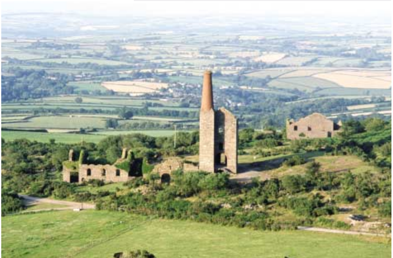
Phoenix Mine, Prince of Wales Shaft, (1907, Listed Grade II). The outstanding engine house was built for the last big pumping engine made in Cornwall (by Holman's Foundry, Camborne). It is a distinctive landmark within the Area and is a monument to spectacular failure and misplaced optimism. The adjacent single-phase group of buildings includes the remains of the boiler house, compressor house, winding-engine house and mill.
