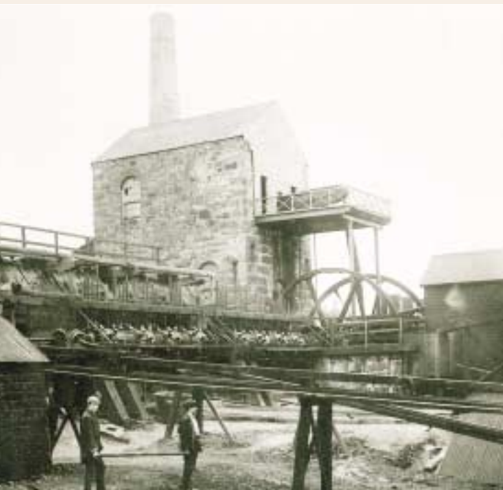
Cornish stamps at South Crofty Mine (A5), c 1907. Revolving cams raised and dropped the heavy stamp heads to crush the tin ore.
