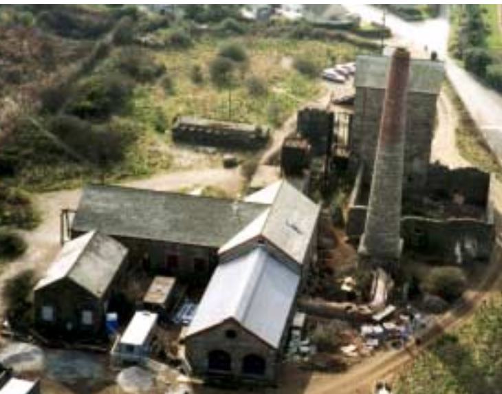
The Taylor's Shaft complex (1920s, Scheduled Monument, Listed Grade II*) at East Pool & Agar Mine during restoration in 1999.
