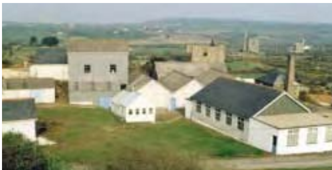
King Edward Mine (Complex Listed Grade II*)
