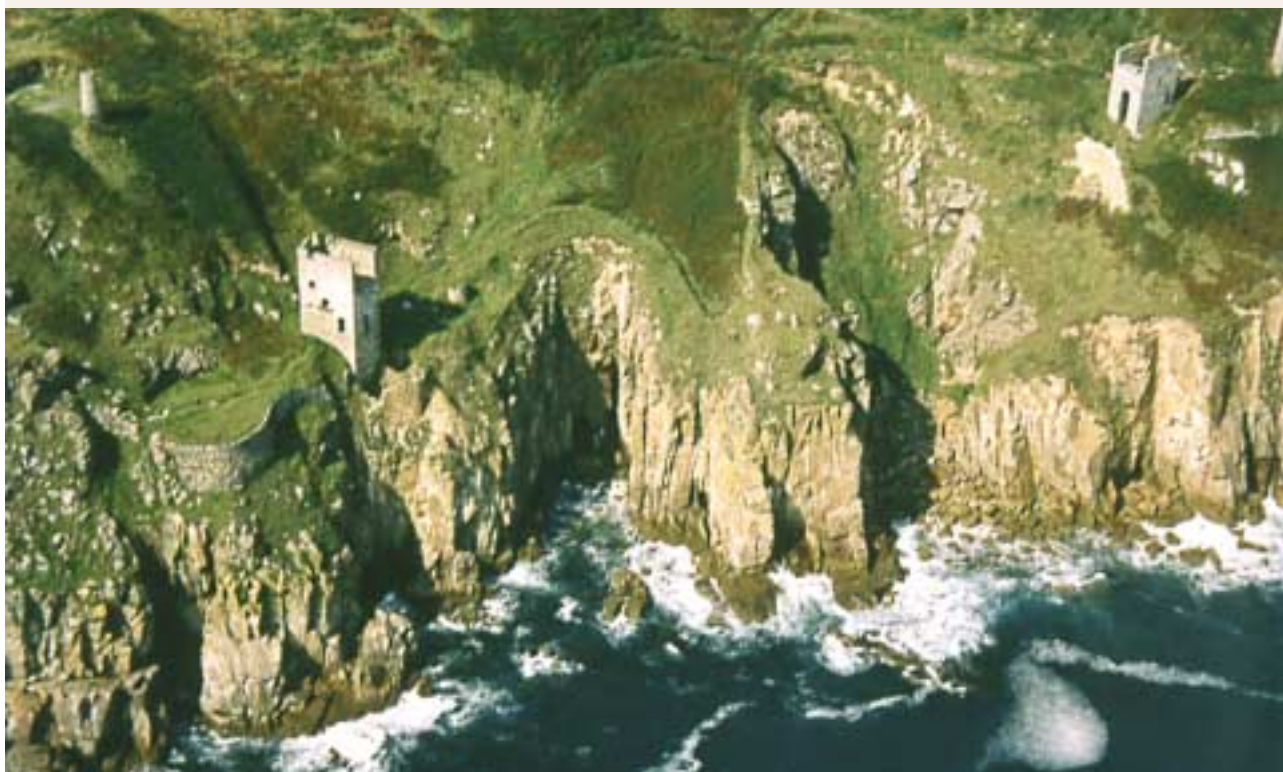
Wheal Trewavas (1838, Scheduled Monument, Listed Grade II). The cliff-side engine houses, shafts and capstan platform are amongst the most spectacular in their situation.
