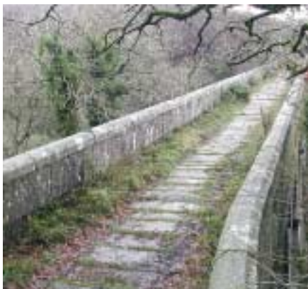
The granite sleepers of the 1835 industrial tramway also acted as lintels for the Carmears Leat that flowed immediately beneath.
