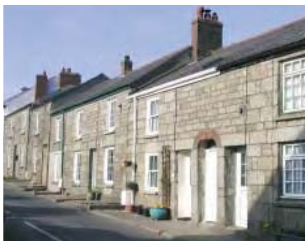
Praze-an-Beeble. Distinctive terraced housing with cut-granite facades. Red brick arches, at intervals, mark traditional passageways (known as opes) leading to premises behind.
