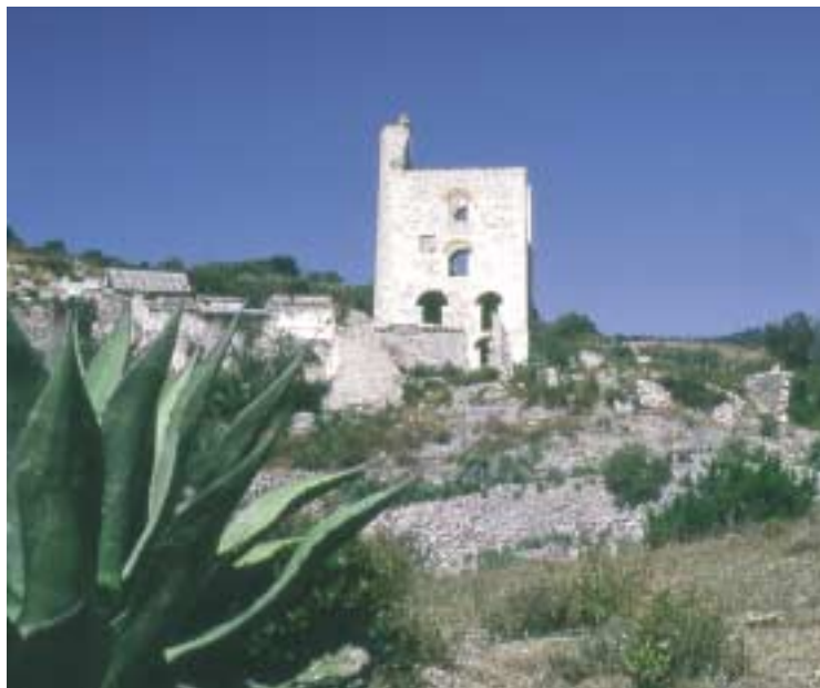
Mina San Pedro la Ravia, Pachuca, Mexico. This pumping engine house is one of eight Cornish engine houses to survive in the Pachuca-Real del Monte silver mining district, in the Sierra Madre north-east of Mexico City. The engine houses, in particular, are now under the care of The Historic Archive and Museum of Mining in Pachuca.
