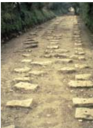
Poldice Plateway (1809). The bed of Cornwall's first plateway survives with many of its granite sett stones still in situ.
