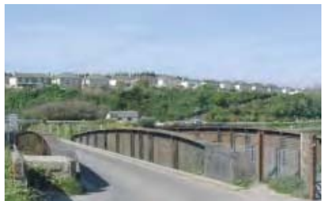
Railway swing bridge (1877, Listed Grade II).
