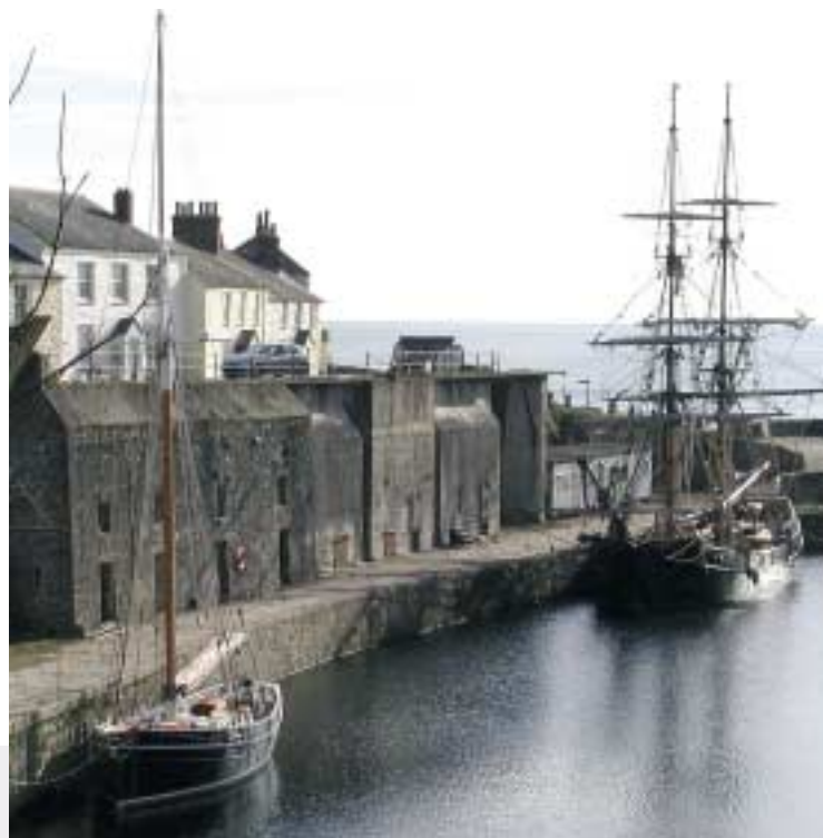
Charlestown Harbour. Inner basin (1798, extended in 1871, Listed Grade II*)
