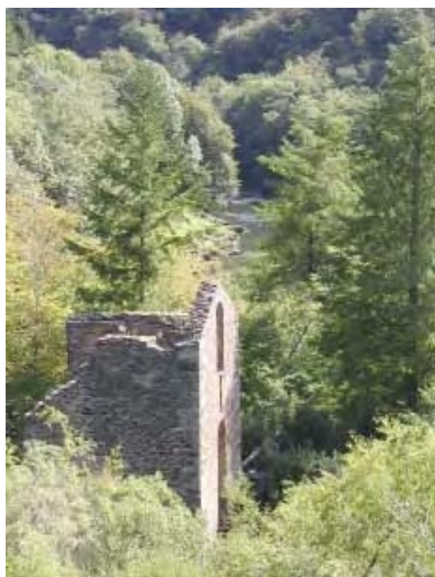
Gunnislake Clitters Mine (Scheduled Monument, Listed Grade II). Some mines are located in the Tamar Valley itself and here the topography imparts an unusual character, some having been worked beneath the river bed. This engine house pumped river water for dressing purposes.
