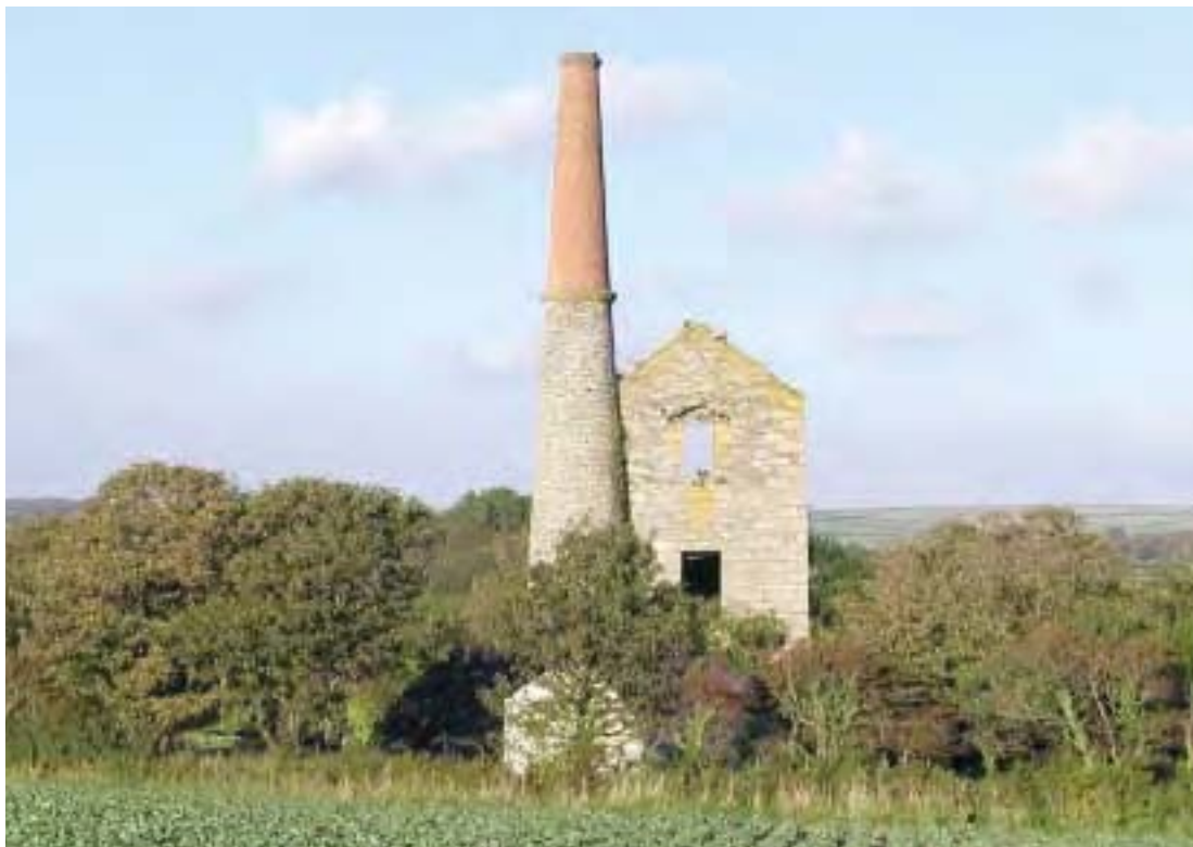
Wheal Vor (Wheal Metal, Listed Grade II). Wheal Vor was an ancient mine associated with the Godolphin family and was the site of the first Newcomen engine in Cornwall, installed during the second decade of the eighteenth century. It was the richest tin mine in Cornwall at its peak in the 1830s. It employed 1,100 persons and was one of the few mines to possess its own smelter.
