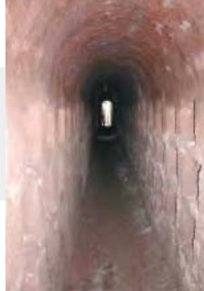
The access tunnel to Man-Engine Shaft showing some of the one hundred alcoves used for the storage of miners' belongings while underground.
