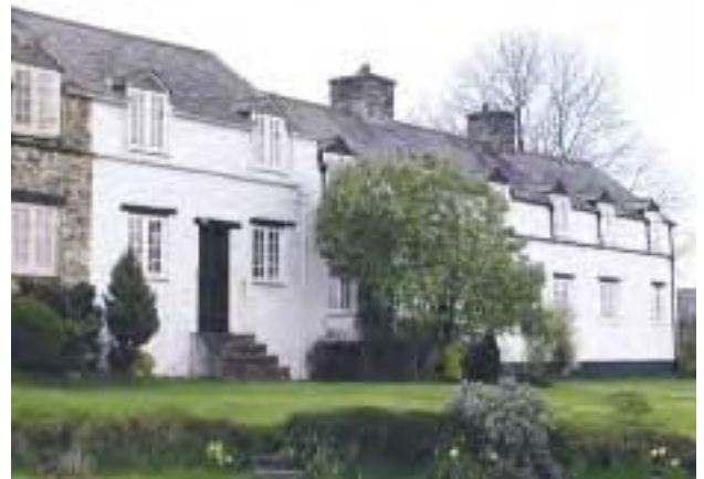
Wheal Josiah Cottages (1854, Listed Grade II) built by the company for key personnel.
