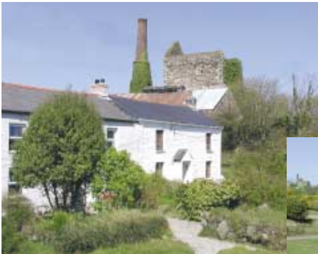
Wheal Busy (Listed Grade II). Rural terraced miners' cottages at this mine where a succession of ten big pumping engines worked – Newcomen, Watt and a range of Cornish engines – from 1725 to 1929.
