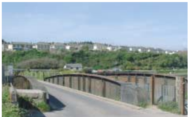
Railway swing bridge (1877, Listed Grade II).
