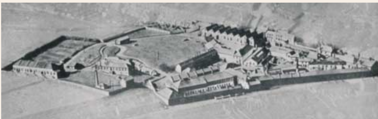
Bickford-Smith's Fuse Works and Foundry Row at Tuckingmill (A5). Early twentieth century aerial photograph (surrounding landscape ghosted by photographer). Today, in countries such as France and Russia, 'Bickford' is synonymous with safety-fuse.
