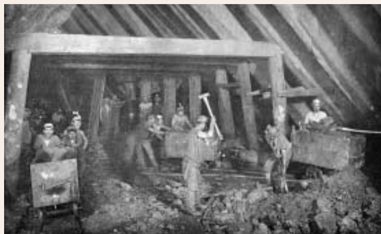
Close-set heavy timbering in the 412 fathom level of Dolcoath Mine. J. C. Burrow, 1893. Shortly after this photograph was taken, the massive timbers collapsed due to a heavy rock fall. Seven miners were killed.
