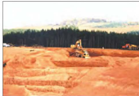
Gravel extraction within the East Devon AONB at Blackhill Quarry.
