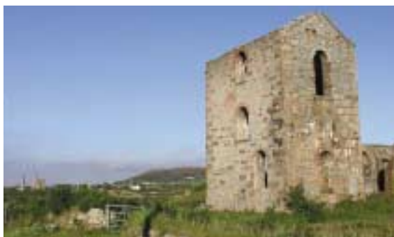
Dolcoath Mine, New East Shaft Whim. One of the four surviving Cornish engine houses of this historic mine.
