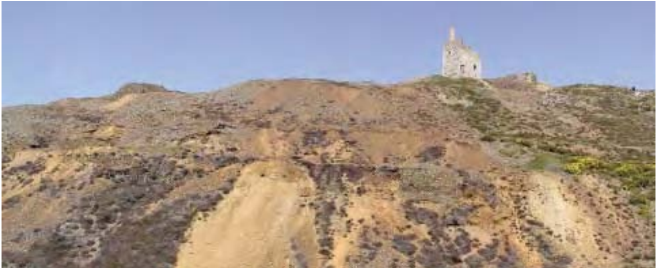
United Hills Mine, John's Shaft (1861, Listed Grade II) on the skyline above Tywarnhayle Valley.
