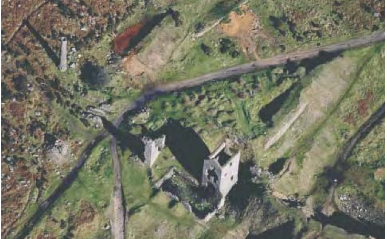
South Caradon Mine. The remains of two pumping engine houses, side-by-side, represent an unusual example within the nominated Site.
