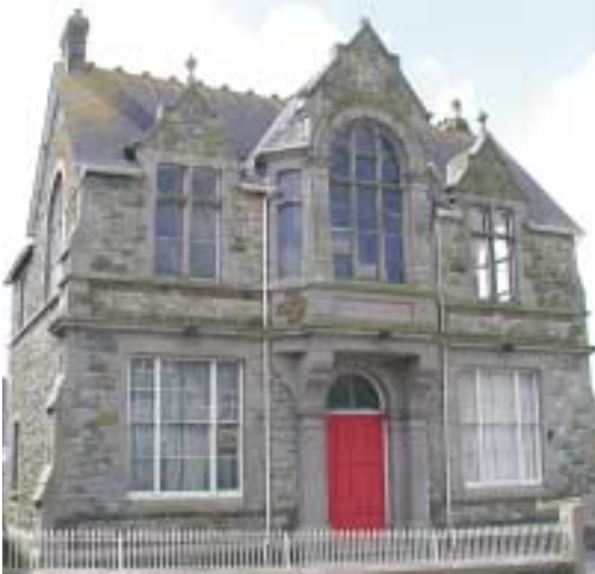
The School of Science & Art (1883) stands next to the Robert Hunt Museum (1890) in Clinton Road. It was built as a memorial to its founder by the Miners' Association of Devon and Cornwall. The Redruth School of Mines was based here and extra-mural classes continued until the 1950s.
