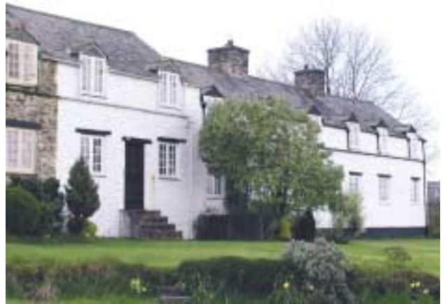
Wheal Josiah Cottages (1854, Listed Grade II) built by the company for key personnel.
