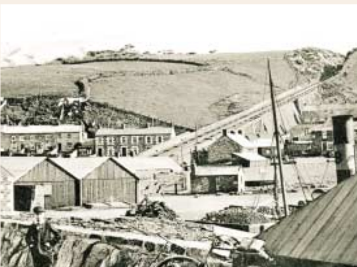
The inclined plane of the Portreath branch of the Hayle Railway (A5). This was operated by a steam whim at the top of the incline.
