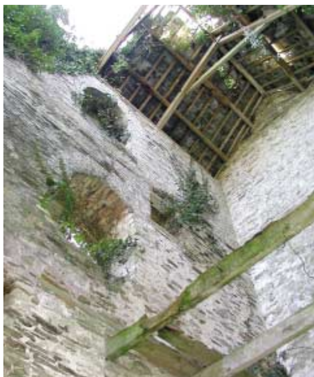
East Holmbush Mine (A10i). Interior of engine house.
