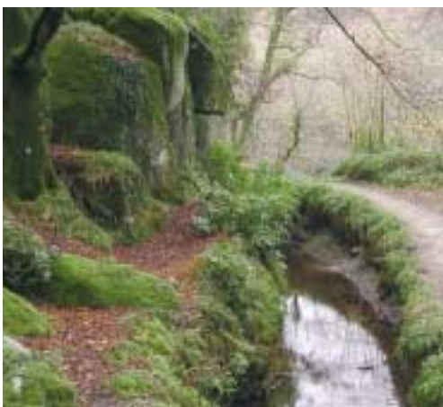
The Fowey Consols leat (1820s) is the earliest civil engineering construction built by Treffry in the Luxulyan Valley. It supplied the Fowey Consols waterwheels and the largest concentration of water power on a nineteenth century copper mine.
