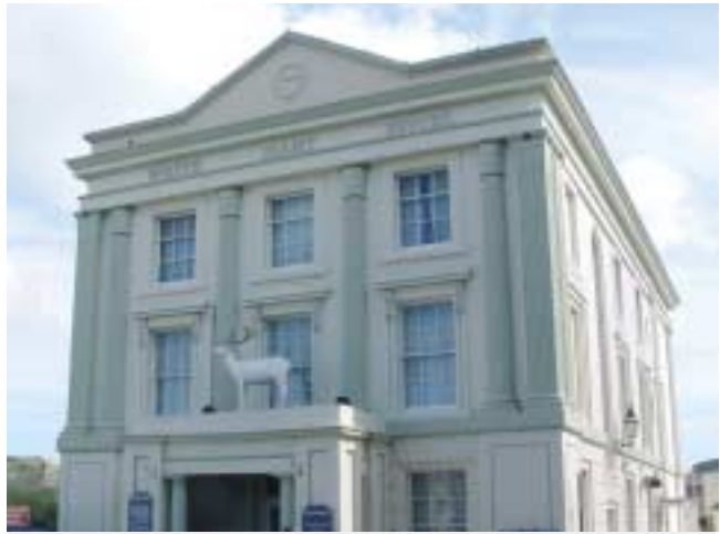
White Hart Hotel (1838, Grade II*). This stands in Foundry Square opposite the site of the former Hayle Railway terminus of 1834.
