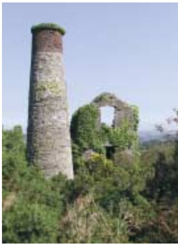
Marke Valley Mine (1876, Scheduled Monument, Listed Grade II). Whim engine house that served Salisbury Shaft.
