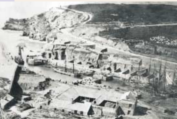
Portreath Harbour (A5), c 1860. Copper-ore was loaded into the schooners from the storage bins along the quay.
