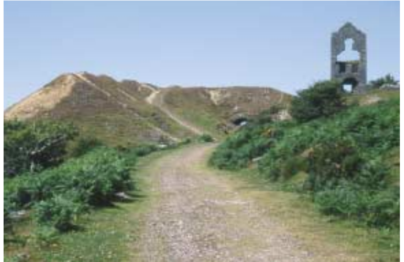
South Caradon Mine (Scheduled Monument). The horse-drawn tramway track-bed passes through a tunnel beneath dumps and past the engine houses at Rule's and Holman's shafts.
