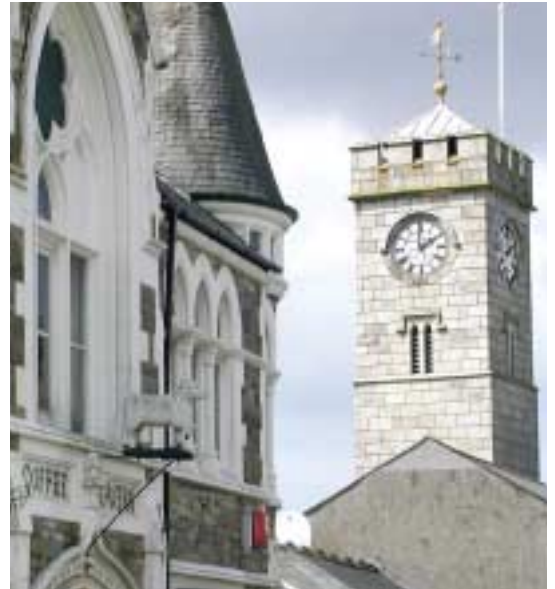
The Coffee Tavern (1880, Listed Grade II) and Town clock (1828, Listed Grade II).
