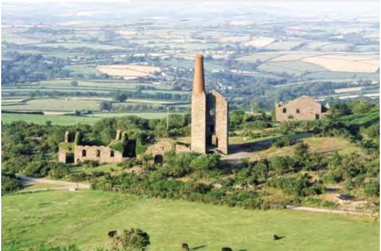
Phoenix Mine, Prince of Wales Shaft, (1907, Listed Grade II). The outstanding engine house was built for the last big pumping engine made in Cornwall (by Holman's Foundry, Camborne). It is a distinctive landmark within the Area and is a monument to spectacular failure and misplaced optimism. The adjacent single-phase group of buildings includes the remains of the boiler house, compressor house, winding-engine house and mill.
