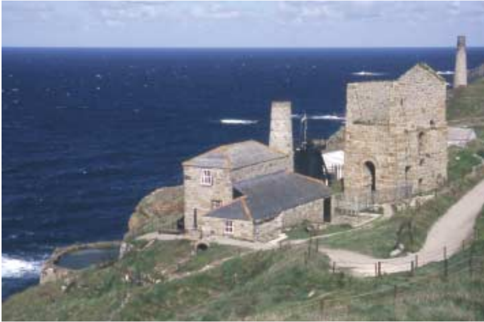
Levant Mine (whim engine house 1840, pumping engine house 1835, Listed Grade II). Levant produced £200,000 worth of high-grade copper-ore in the first ten years of working. One hundred years later it was the last of the larger copper mines to close, having also been rich in tin.
