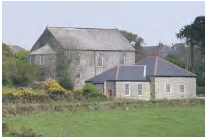
Porkellis chapels (1814 Listed Grade II, 1866 Listed Grade II*). The early nineteenth century chapel at Porkellis was converted into a schoolroom when the larger 1866 chapel was built alongside, using dressed granite from a demolished engine house. It has hardly been modified since its construction, which is rare, and it contains a central row of box pews with rows of benches on each side which were the free seats.
