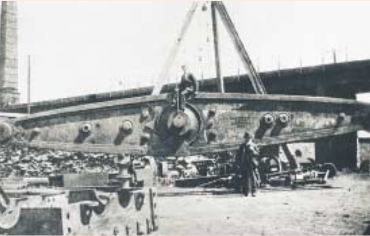
Harvey's Foundry, Hayle (A2), c1890. Harvey's were noted for the production of large beam pumping engines. A cast-iron 'bob' is pictured in their yard. Hayle railway viaduct behind.
