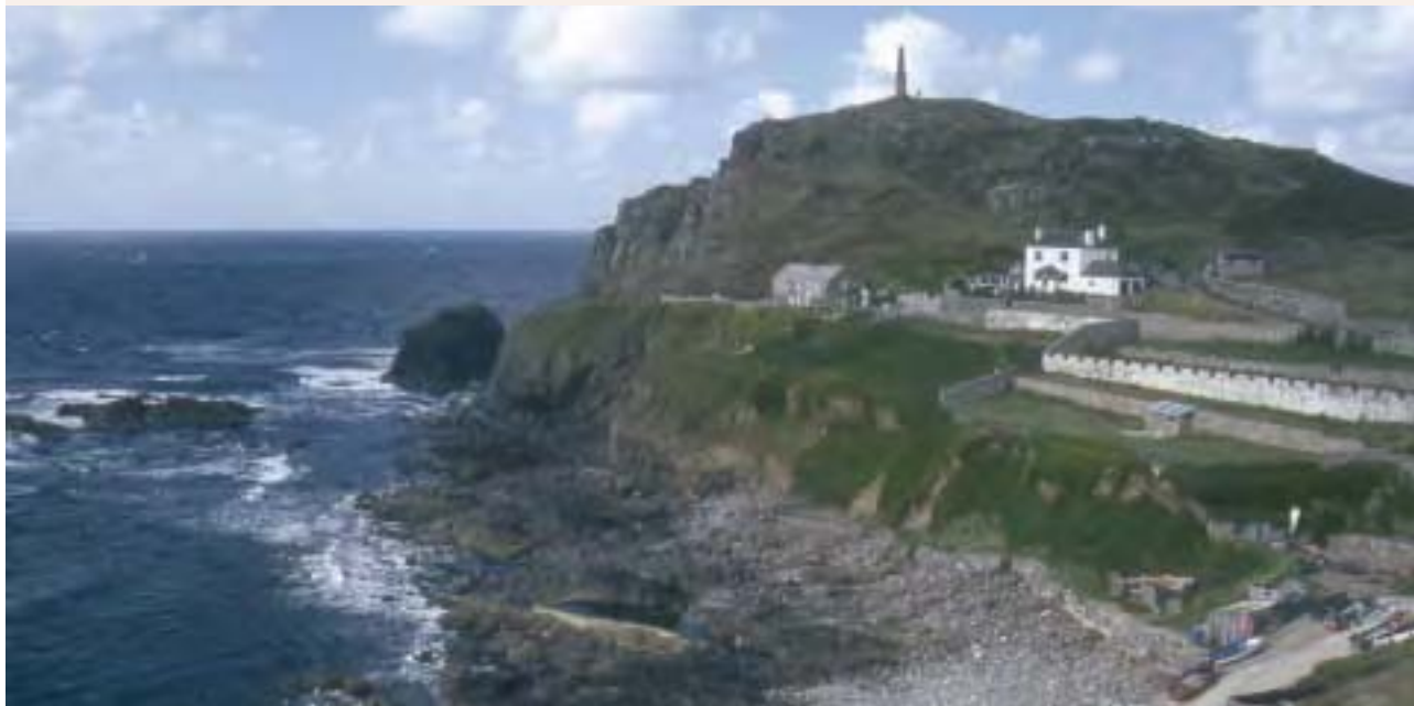
Cape Cornwall. The ornate stack (1850s, Listed Grade II) of Cape Cornwall Mine, which crowns the summit of England's only cape, is one of a number of mining structures that serve as prominent sea-marks along this rugged stretch of coastline; the white building was the mine's count house. Priest's Cove was St Just's harbour for centuries.
