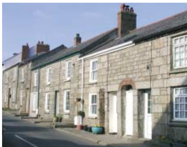
Praze-an-Beeble. Distinctive terraced housing with cut-granite facades. Red brick arches, at intervals, mark traditional passageways (known as opes) leading to premises behind.
