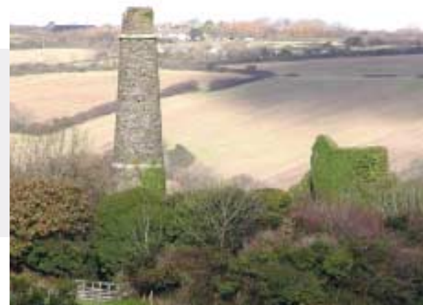
Cusvey Mine. The engine house and stack date from the 1820s and are amongst the earliest that survive in the nominated Site.
