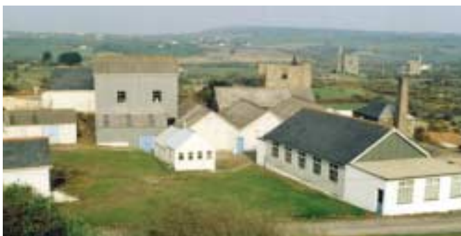
King Edward Mine (Complex Listed Grade II*)
