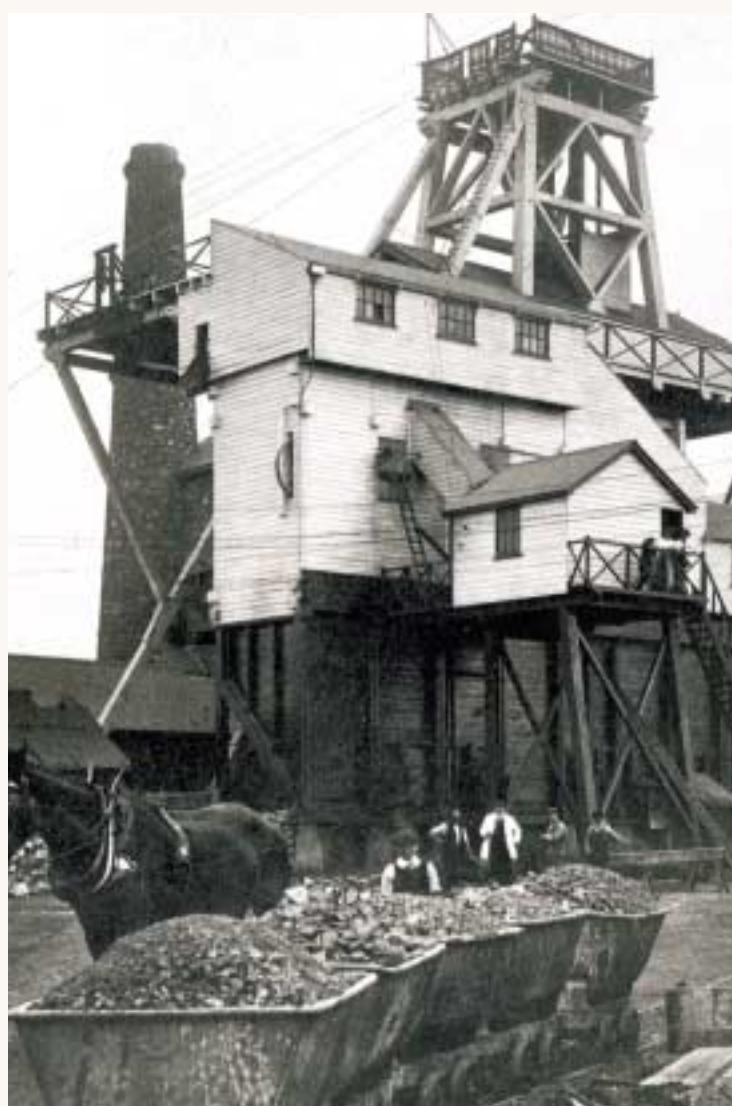
Robinson's Shaft, South Crofty Mine (A5), c 1910. In front of the engine house is the new headgear and rock-breaker plant. The train of wagons are filled with ore and are on the horse-drawn tramway which led to the mill.
