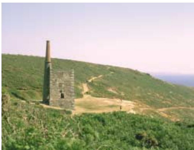
Wheal Prosper (1860, Scheduled Monument, Listed Grade II). The cliff-slope engine house was acquired by the National Trust in 1969 and consolidated during 1970/71.
