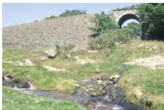
Liskeard and Caradon Railway bridge (Listed Grade II) and embankment at South Caradon Mine. The Seaton Stream in foreground.
