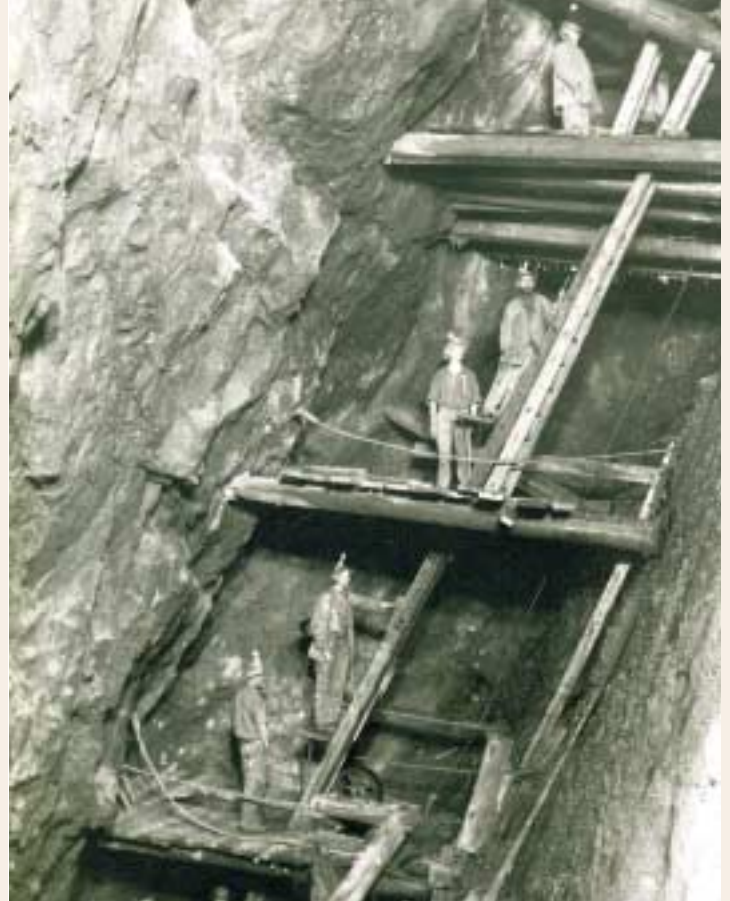
The man-engine at Dolcoath Mine, photographed by J C Burrow and published in 1893. The man-engine was a means of ascending and descending the mine by stepping on and off the platforms of the reciprocating engine-rod.
