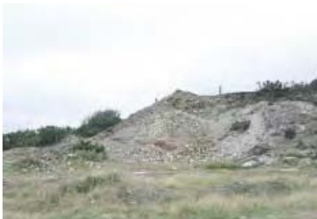
Mine spoil heap removal at Wheal Uny, Redruth.
