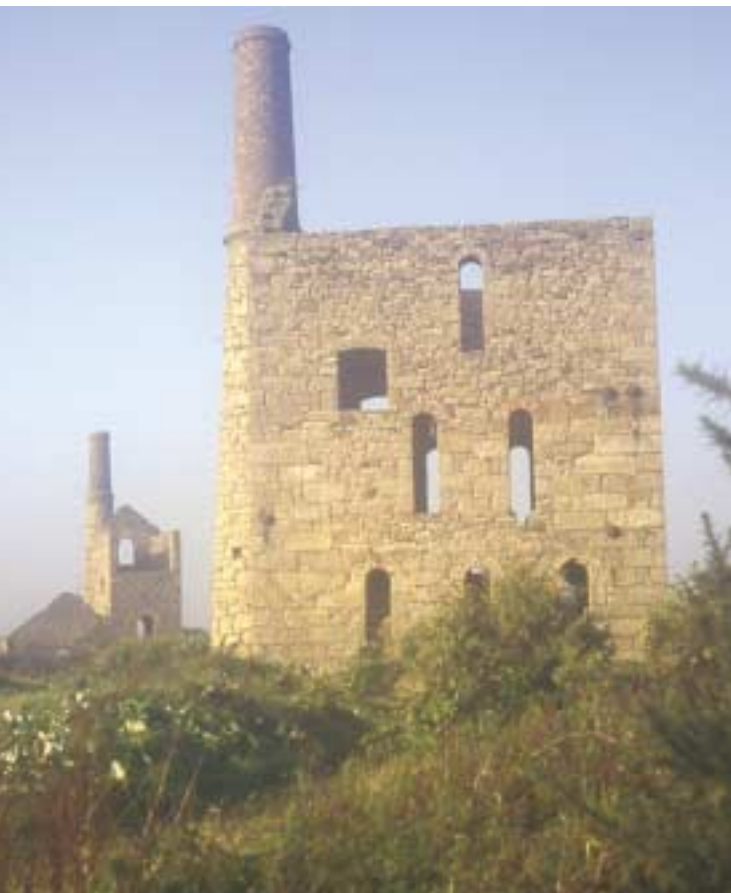
Basset Mines (A5, Listed Grade II). Pumping engine house (foreground) and whim engine house (background) at Pascoe's Shaft, South Wheal Frances section.
