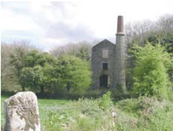
Basset & Grylls Mine (also known as Porkellis United). The pumping engine house at Tyacke's Shaft was built following the tragic flooding of an older section of the mine when water and fine-grained tin 'slimes' collapsed into the workings.
