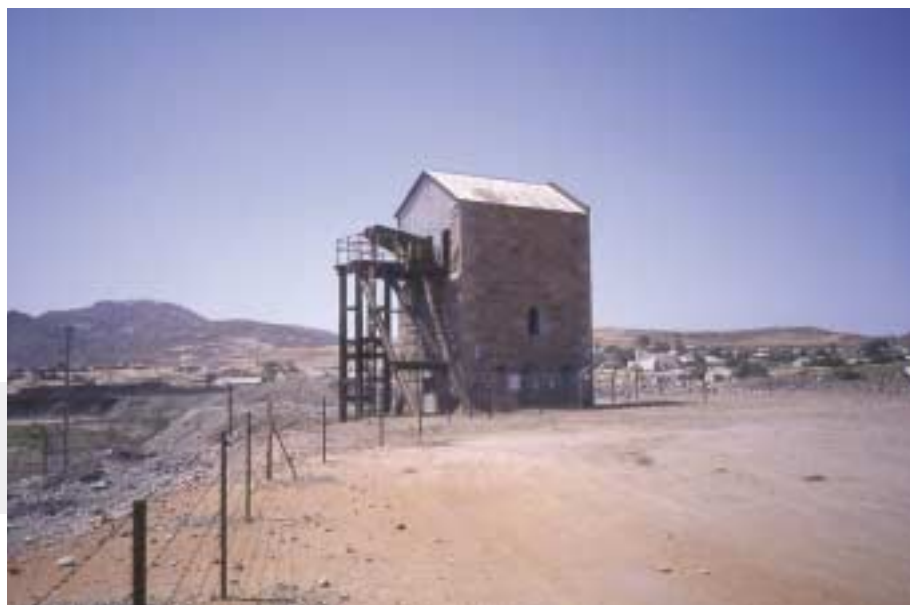
O'okiep Mine, South Africa (National Monument). The beam pumping engine, manufactured by Harvey's of Hayle, is the only such engine to survive in situ in the southern hemisphere.
