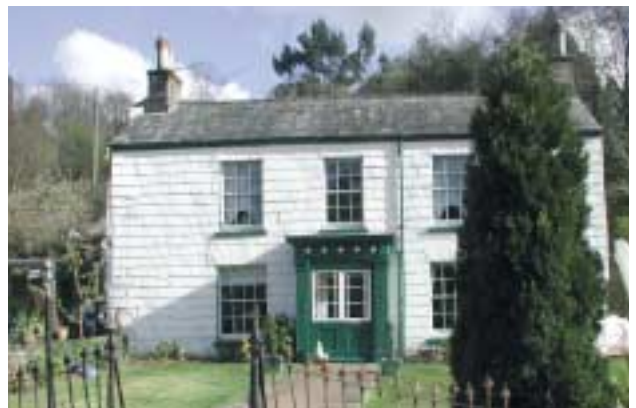
Devon Great Consols, Captains' house. A self-contained community lived in company-built housing on the mine.
