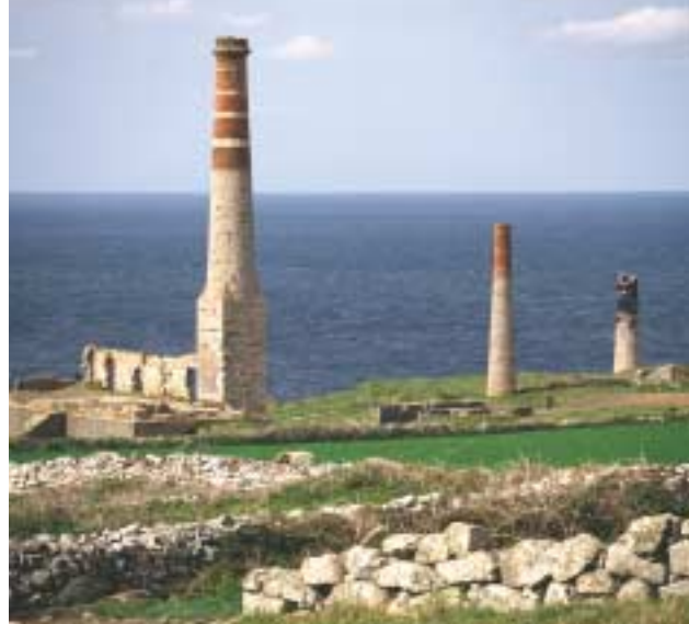
Levant Mine (A1, 1901). The recently consolidated compressor house remains (left) formerly contained an air-compressor made in 1901 by Holman's of Camborne. It was described by The Mining Journal as "the biggest piece of machinery of its kind ever erected in the County."
