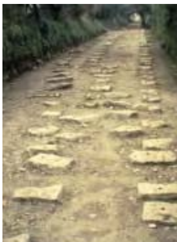
Poldice Plateway (1809). The bed of Cornwall's first plateway survives with many of its granite sett stones still in situ.
