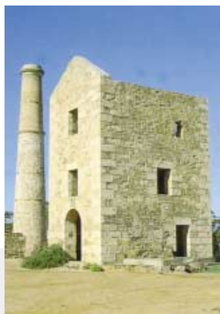
Moonta Mine, South Australia. Hughes engine house (erected 1864) housed one of a number of Cornish engines that were sent to Australian mines around the mid-nineteenth century. There are seven Cornish engine houses surviving in South Australia.
