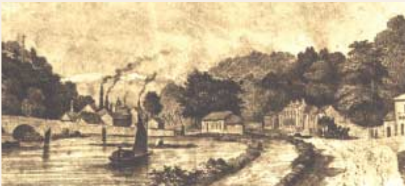
Perran Foundry (A6), late nineteenth century woodcut. A settlement grew up around the great iron foundry and from here iron barges took heavy engine parts to their quay at Devoran for shipment.
