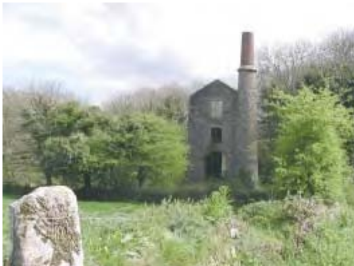
Basset & Grylls Mine (also known as Porkellis United). The pumping engine house at Tyacke's Shaft was built following the tragic flooding of an older section of the mine when water and fine-grained tin 'slimes' collapsed into the workings.
