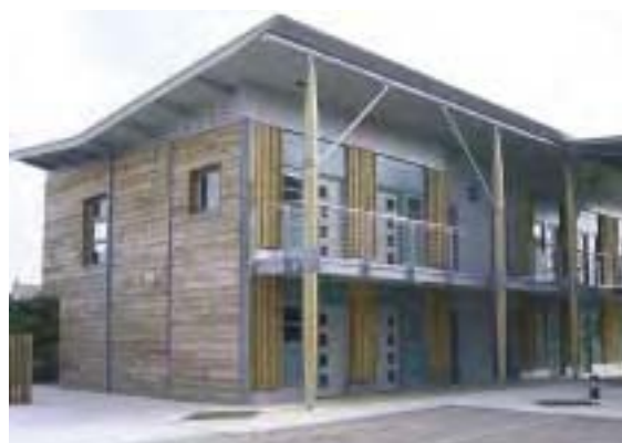
Harvey's Foundry Phase One start-up units. A modern high quality design which respects the historic foundry setting.
