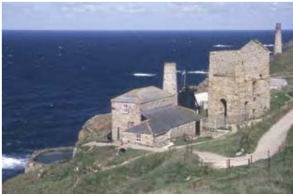
Levant Mine (whim engine house 1840, pumping engine house 1835, Listed Grade II). Levant produced £200,000 worth of high-grade copper-ore in the first ten years of working. One hundred years later it was the last of the larger copper mines to close, having also been rich in tin.
