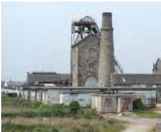
Robinson's Shaft complex, South Crofty Mine, Pool. The effects of neglect and vandalism are readily apparent at this mine site which was decommissioned in 1996. It is hoped that regeneration efforts will secure funding to conserve this important part of Pool's industrial history.
