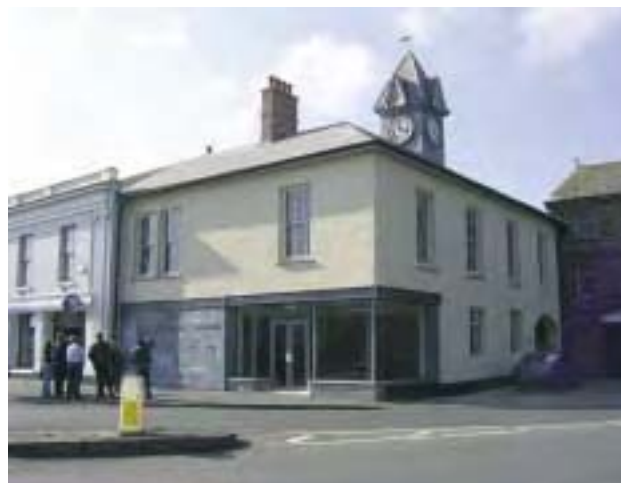
24 Foundry Square after the completion of renovation works. Regeneration efforts have successfully consolidated this important historic building and returned it to use.
