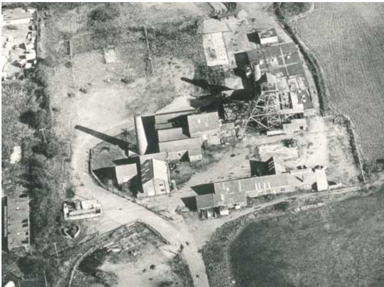
Robinson's Shaft complex, South Crofty Mine (A5, Scheduled Monument, Listed Grade II*). Detailed assessment identifies earlier elements of the mining landscape, such as the circular powder magazine (1850s, bottom left) and the engine house (1903, centre right) adjacent to the shaft with a modern headframe. Most of the surrounding buildings date from the second half of the twentieth century.
