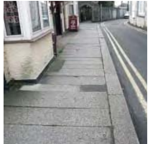
Camborne - street paving. Granite paving slabs are a distinctive element of the urban fabric in towns across Cornwall and west Devon.
