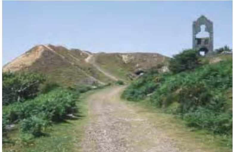
South Caradon Mine (Scheduled Monument). The horse-drawn tramway track-bed passes through a tunnel beneath dumps and past the engine houses at Rule's and Holman's shafts.
