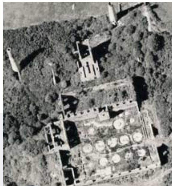
West Basset Mine, New Stamps (1875, Listed Grade II). The stamps were made by the Tuckingmill Foundry and remains of the dressing floors show three different phases - settling and buddling (1875), additional buddle floor (1892), and the installation of Frue vanners (1906).
