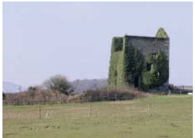
Fowey Consols, Austen's engine house (1834, Listed Grade II). The landmark engine house contained the most efficient Cornish beam pumping engine ever made (William West).
