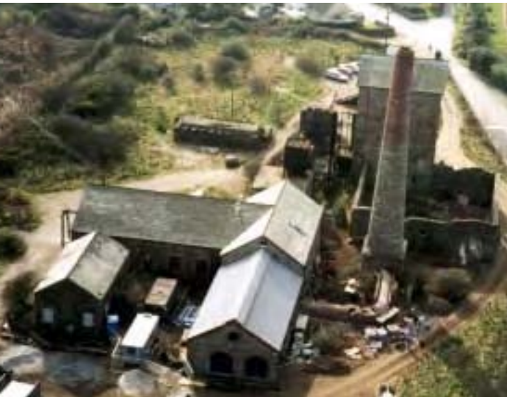
The Taylor's Shaft complex (1920s, Scheduled Monument, Listed Grade II*) at East Pool & Agar Mine during restoration in 1999.
