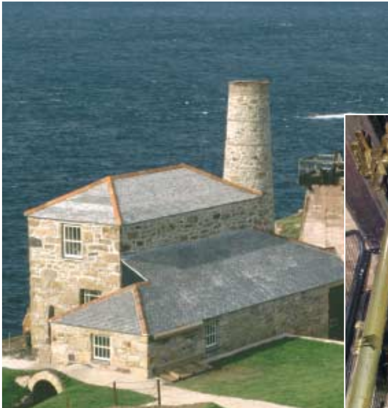
Levant Mine (A1, 1840, Listed Grade II). The restored engine house contains an all-indoor beam whim that was designed by Francis Michell and made by Harvey & Co., Hayle, in 1840. It worked until 1930 and was the first engine to be preserved by the Cornish Engines Preservation Committee, formed in 1935. It is now under the care of the National Trust.
