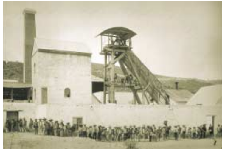
Mina Corteza, Pachuca, Mexico, 1899. Cornish miners and engineers first brought steam engines to the silver mines of Pachuca-Real del Monte in the 1820s.
