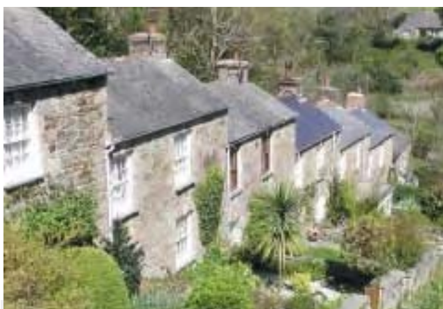
Stippy Stappy (Listed Grade II). A traditional stepped terrace of cottages originally built for ships' captains sailing from Trevaunance Harbour.
