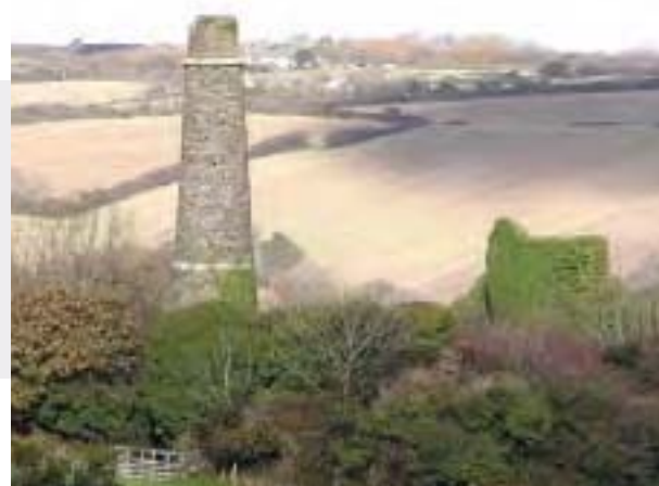
Cusvey Mine. The engine house and stack date from the 1820s and are amongst the earliest that survive in the nominated Site.
