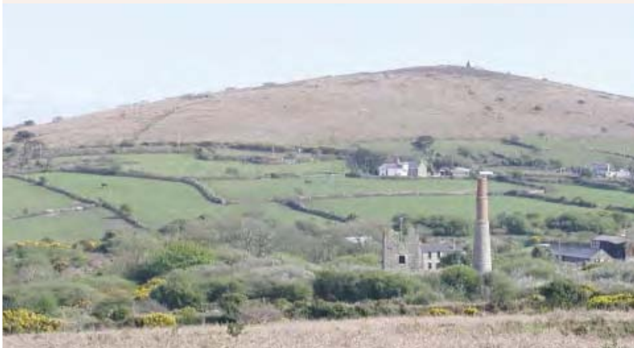
Tregonning Hill and Great Work Mine (Leeds' Shaft, 1850s, Listed Grade II). Great Work was a very rich tin mine with one of the longest recorded histories – over 400 years - of any Cornish mine.
