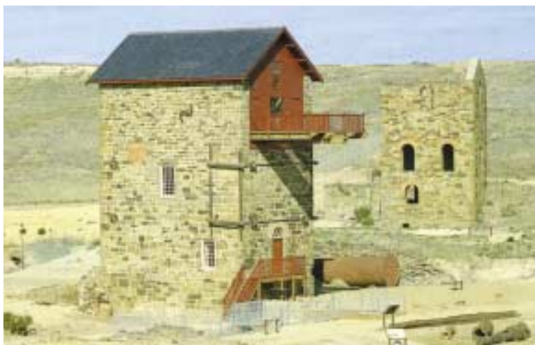
Burra Burra Mine, South Australia. Morphett's pumping engine house (erected in 1858, and reconstructed in 1986) with the whim engine house (1861) behind.
