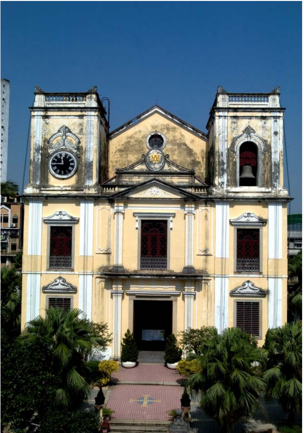
ILLUSTRATION DOCUMENT 17 Façade of St. Lawrence's Church
