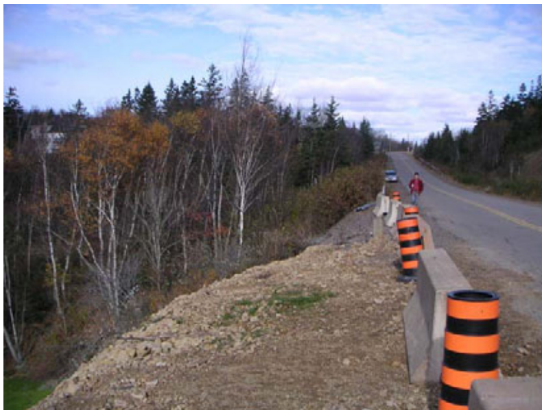
Figure 15 - Poor sight lines to McCarrons River access road (near car in picture)
