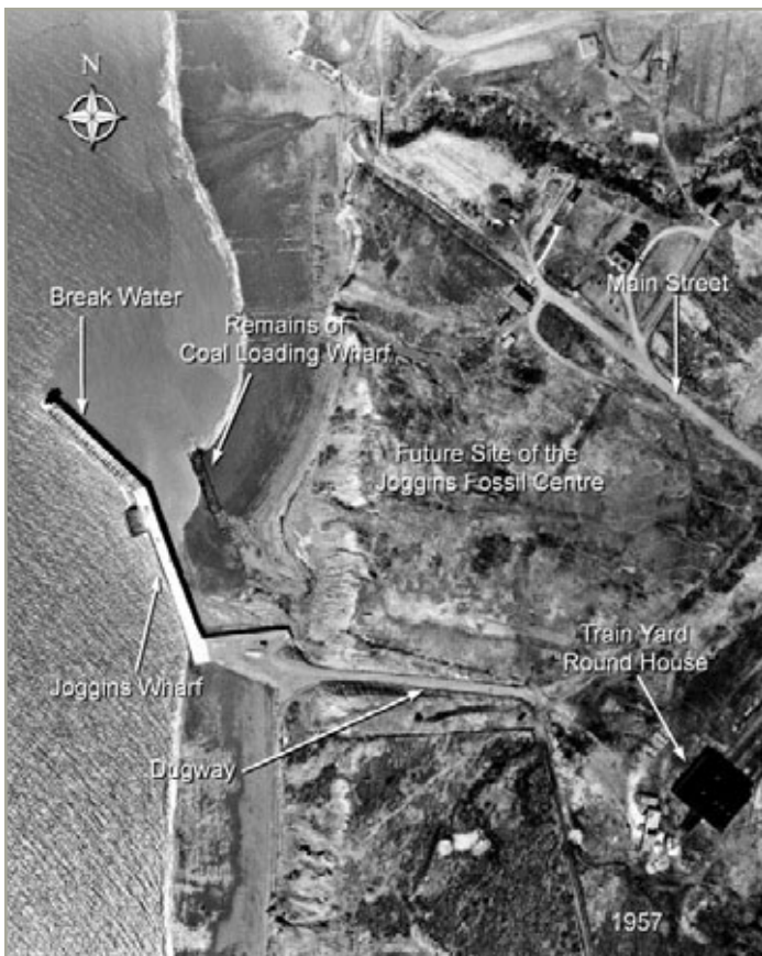
Figure 106 Airphoto of the coal loading wharf and breakwater at the Joggins seam.
