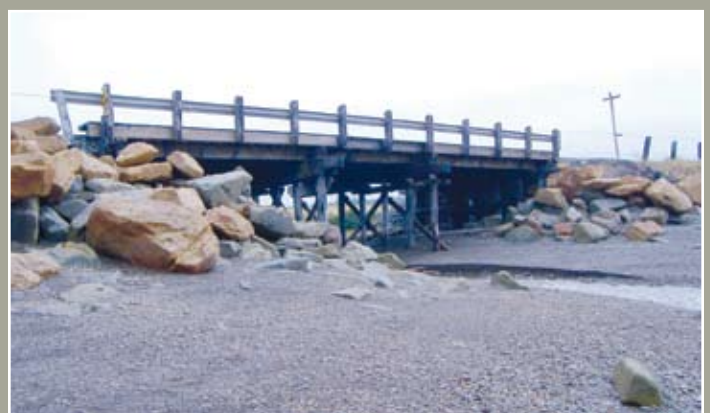
Figure 112 Highway bridge over Little River at Lower Cove.
