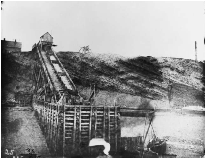
Fig. 6. The new Joggins wharf near Bell's Brook photographed in 1879 by Weston. Note the slide used to transport coal from the mine (just visible over the cliff top) onto waiting ships and the great height of the wharf, designed to deal with 40 ft tides on the Bay of Fundy. Source: GSC/Library and Archives of Canada PA-05119.
