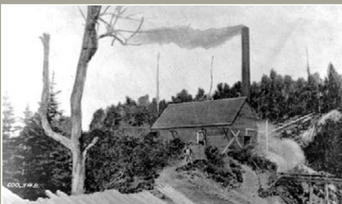
Figure 111 Pump station at MacCarron's River, circa 1910.
