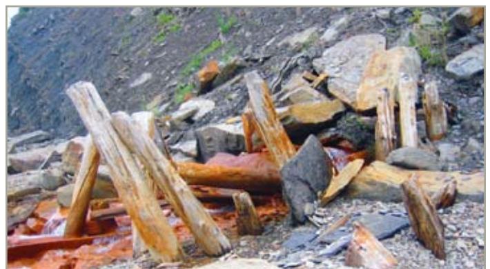
Figure 108 Remnant pilings of the coal loading wharf at the Joggins seam.
