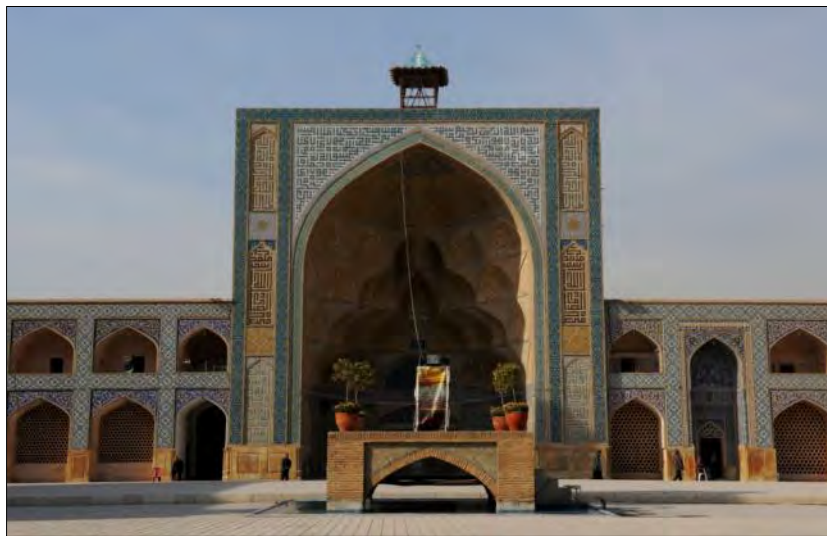
Photo 2-20. The western Ayvān (Soffe' Ostad)(MJIB, Bakhtiar)
