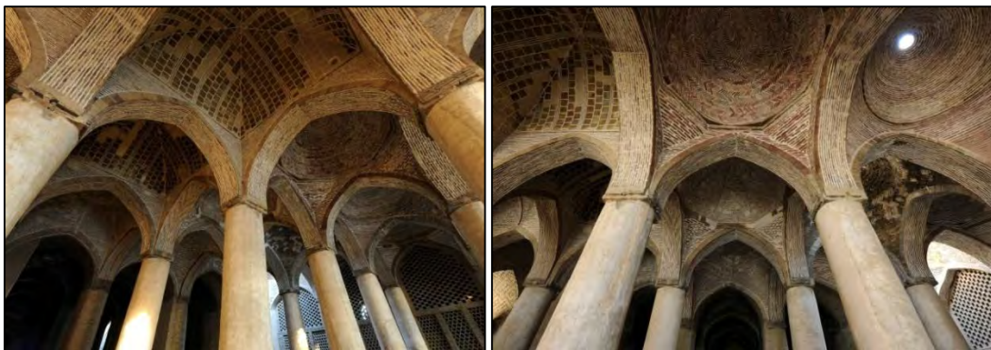
Photo 3-5. Variety of vaulting techniques in Seljuq Shabestan (MJIB, Bakhtiar, 2010)
