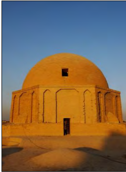
Photo 2-8. Nezam al-Molk dome (MJIB, Bakhtiar)
