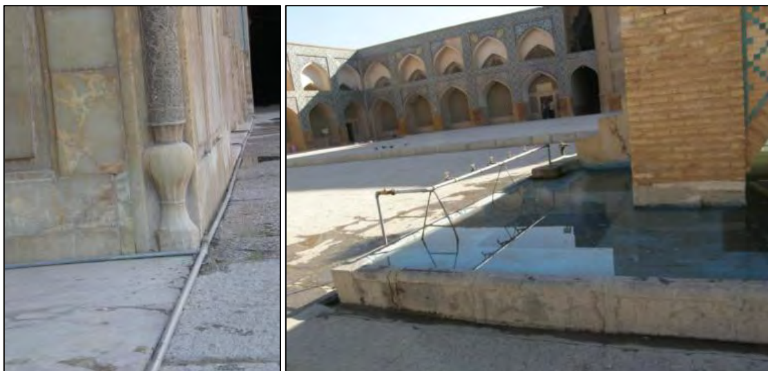
Photo 4-20. Contemporary utilities in the Masjed (MJIB, Jabal Ameli)
