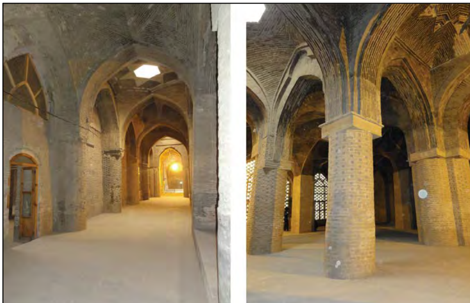
Photo 4-8. The mud brick wall in the library (MJIB, Jabal Ameli)
