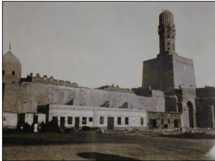
Photo 3-26. General view of Masjed-e Al Hakim (MJIB)
