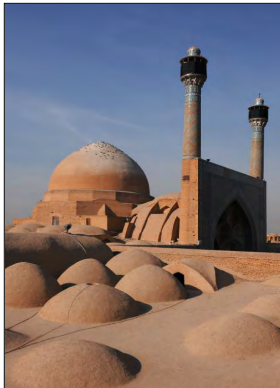
Photo 3-2. Nezam al-Molk dome (MJIB, Bakhtiar, 2010)
