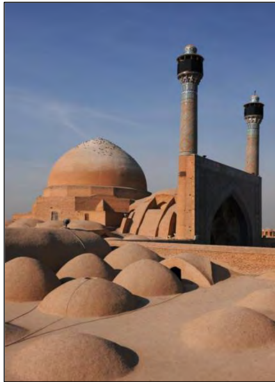
Photo 4. Nezam al-Molk dome (MJIB, Bakhtiar, 2010)
