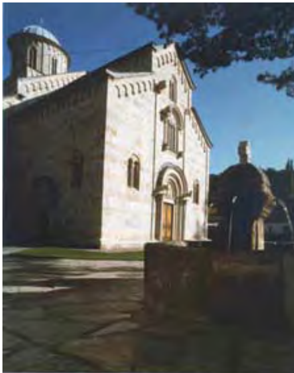
Figure 8. Dečani Monastery, Northwest view of the church /photo by Branislav Strugar/
