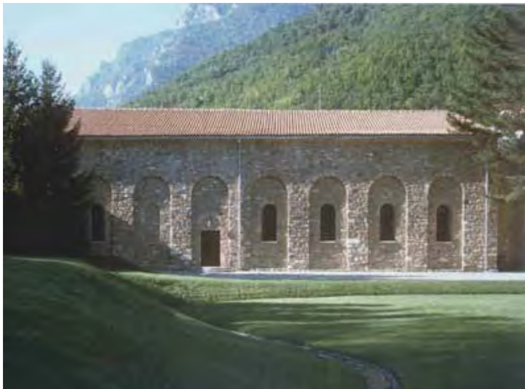
Figure 6. Dečani Monastery, Refectory /photo by Branislav Strugar/
