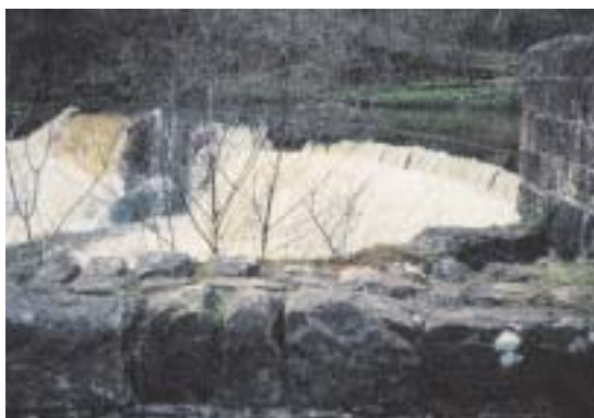
Orbiston, Motherwell, Lanarkshire: the site of the communal building and re-used stone from it at a forge nearby (in 2000).
