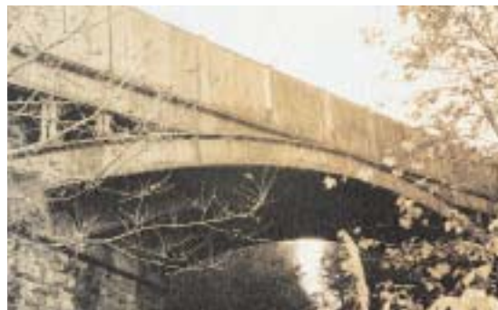
Bonnington Road Bridge
