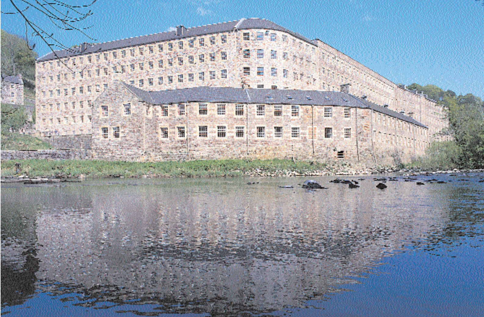
Above: New Lanark Mills Numbers 1-3, and Waterhouses
