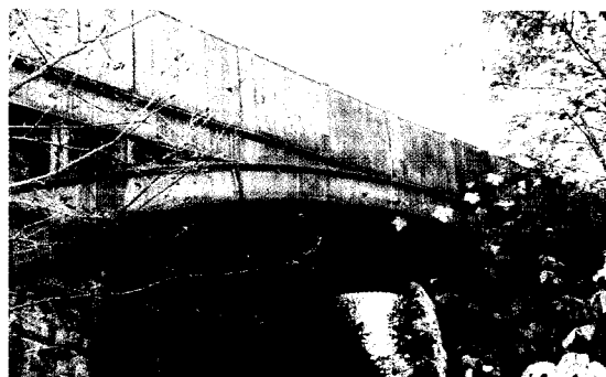
Bonnington Road Bridge
