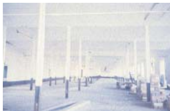
Ditherington Flax Mill, Shrewsbury, England, the world's first iron framed building, erected in 1797.
