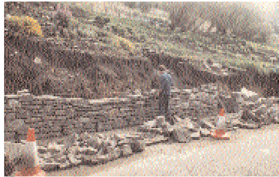
The retaining wall at Braxfield Row (NLCT)
