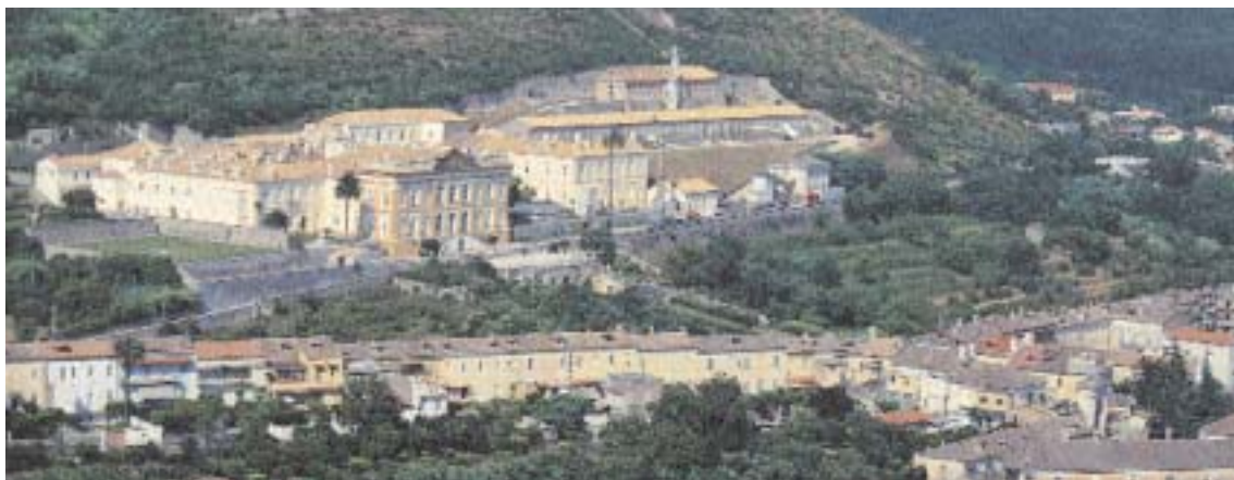
San Leucio, Italy. The only part of the radially-planned town to be completed is in the foreground. The silk works is uphill to the left, arranged around a courtyard, and the terraced Filanda dei Cipressi cotton mill was added to its right in circa 1826-30. (G E Rubino, Università degli Studi di Napoli Federico II)
