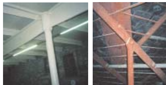
Iron frame and roof in the fireproof link between Mills 3 and 4
