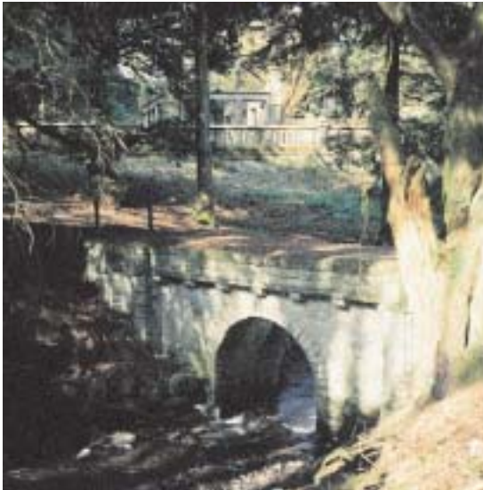
Conservatory Bridge and Conservatory
