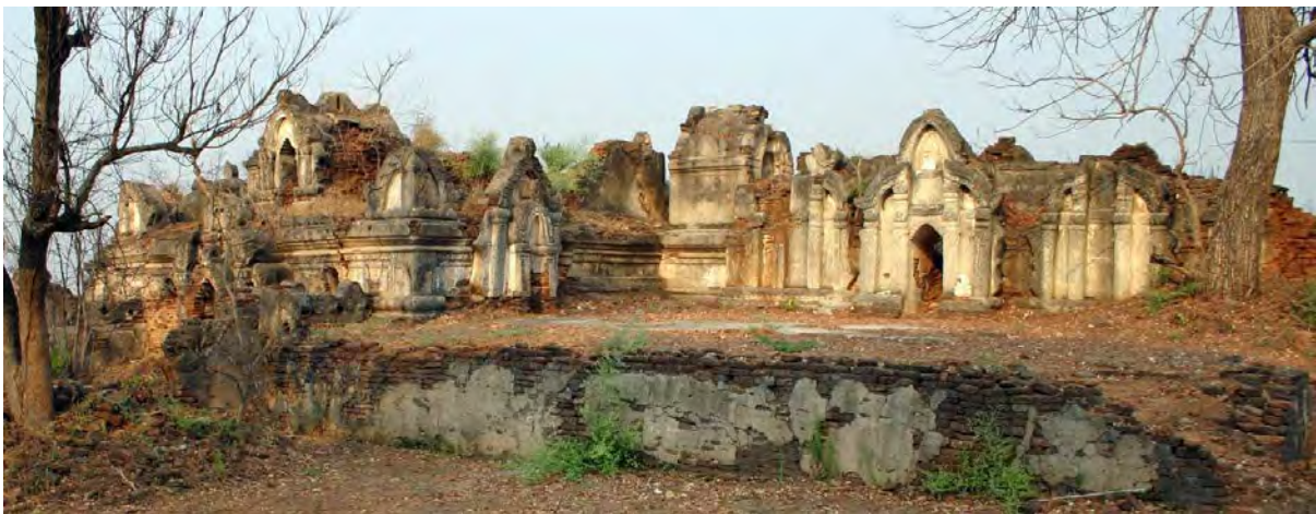
LATE 19TH CENTURY CE MONASTIC STRUCTURE ON HALIN CITY WALL
