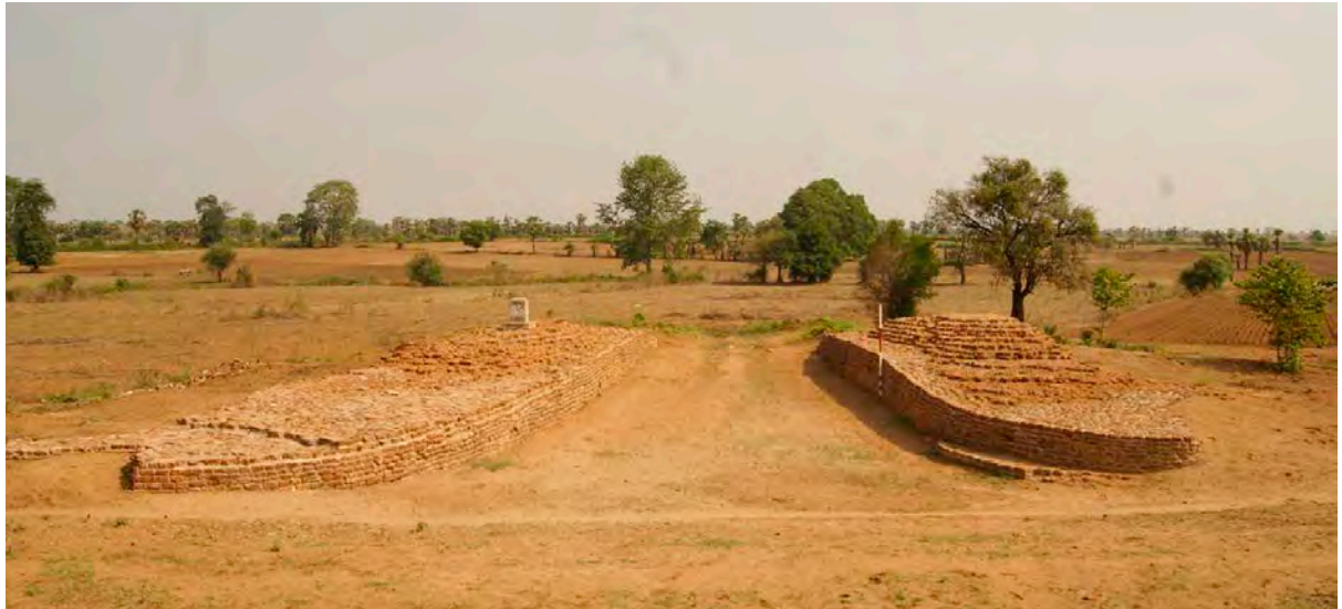
PRESENT STATE OF HL-10 GATE (HALIN)
