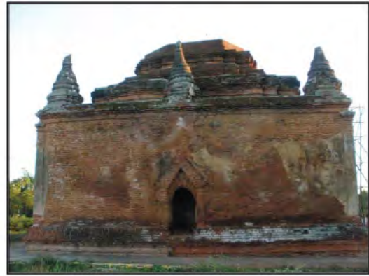
Photo from North side
