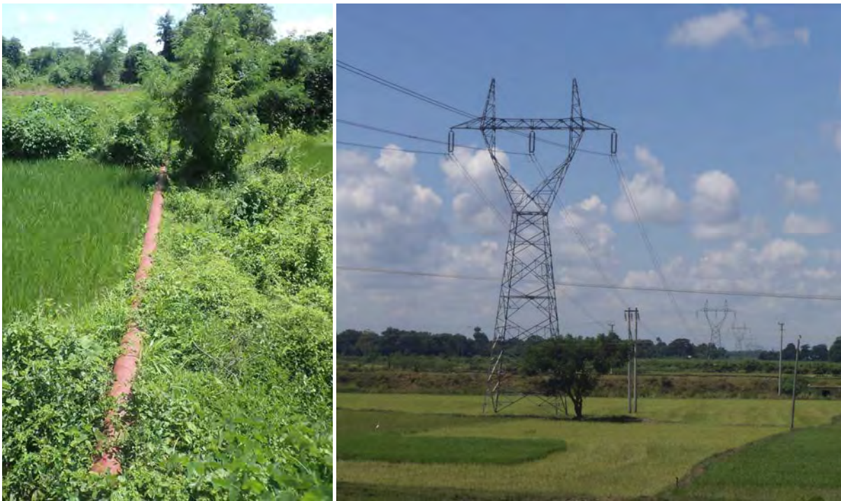
GAS PIPE LINES AND ELECTRICAL PYLONS (SRI KSETRA)
