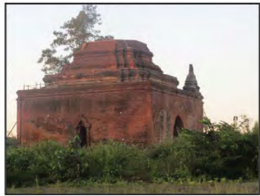
Photo from Southeast corner
