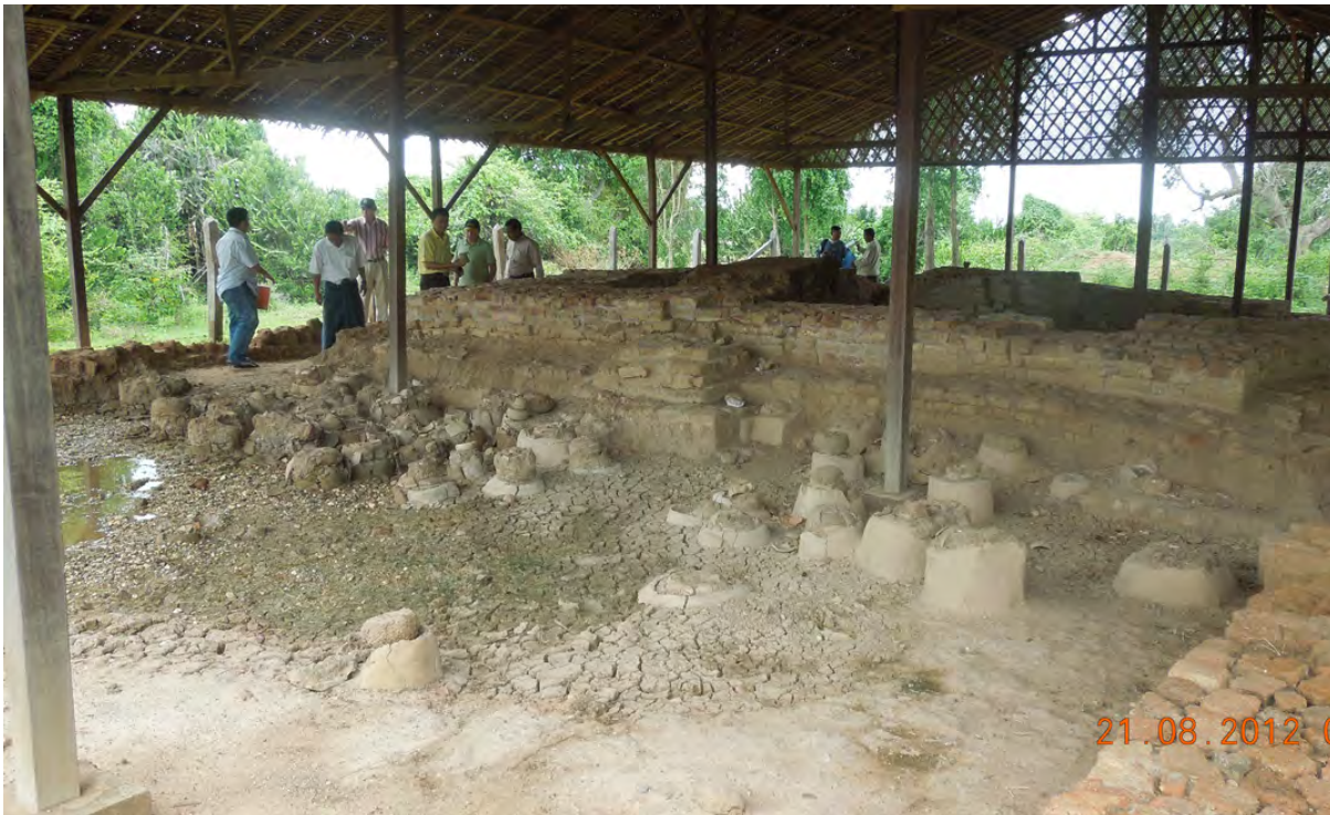
MEMORIAL HALL WITH URNS WHERE SHELTER HAS PROVIDED ONLY PARTIAL PROTECTION (BEIKTHANO)
