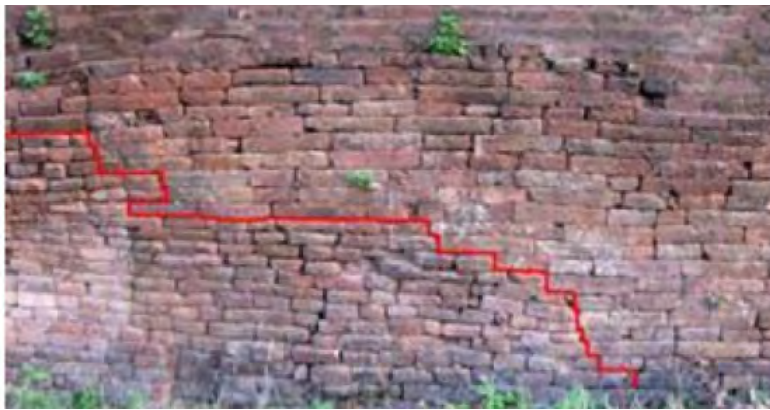
DETAIL OF LULIN-KYAW GATE (RED LINE) SHOWING MODERN RESTORATION OVERLYING ANCIENT PHASES (SRI KSETRA)
