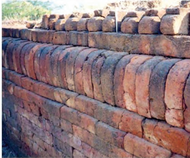
WALL BTO-5 WITH LARGE BRICKS AND SPECIALIZED BRICK MASONRY (BEIKTHANO)
