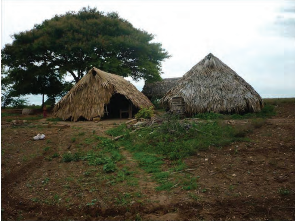
TEMPORARY RESIDENTIAL STRUCTURES WITHIN THE BOUNDARY OF THE PROPERTY (HALIN)
