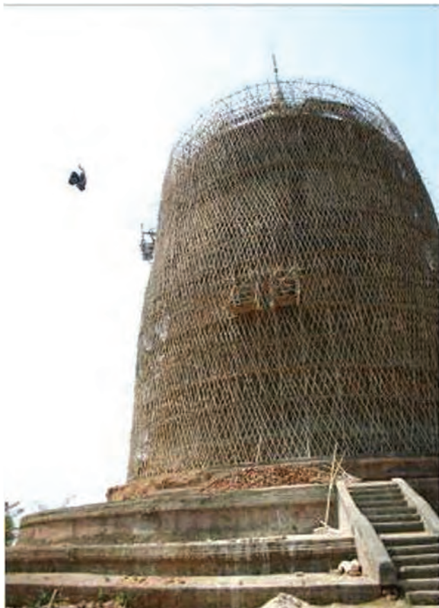
LARGE STUPA COVERED AND READY FOR REPAIR
