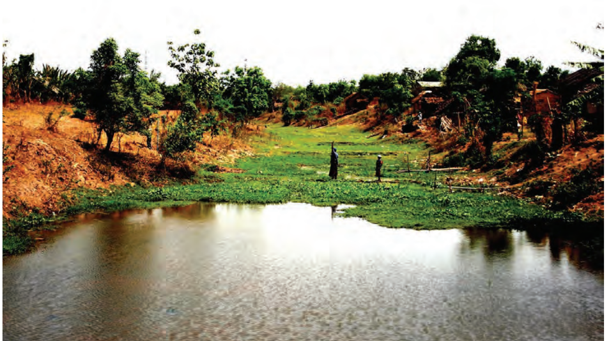
PRESENT CONDITION OF THE MOAT (SRI KSETRA)
