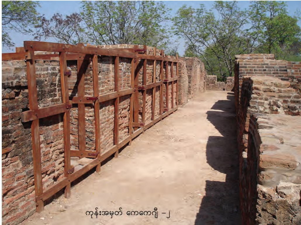
STABILIZATION OF MONASTIC STRUCTURE KKG-2 UNDERTAKEN IN 2009 (BEIKTHANO)
