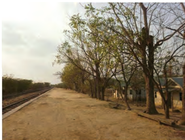
RAILROAD TRACKS (BEIKTHANO)
