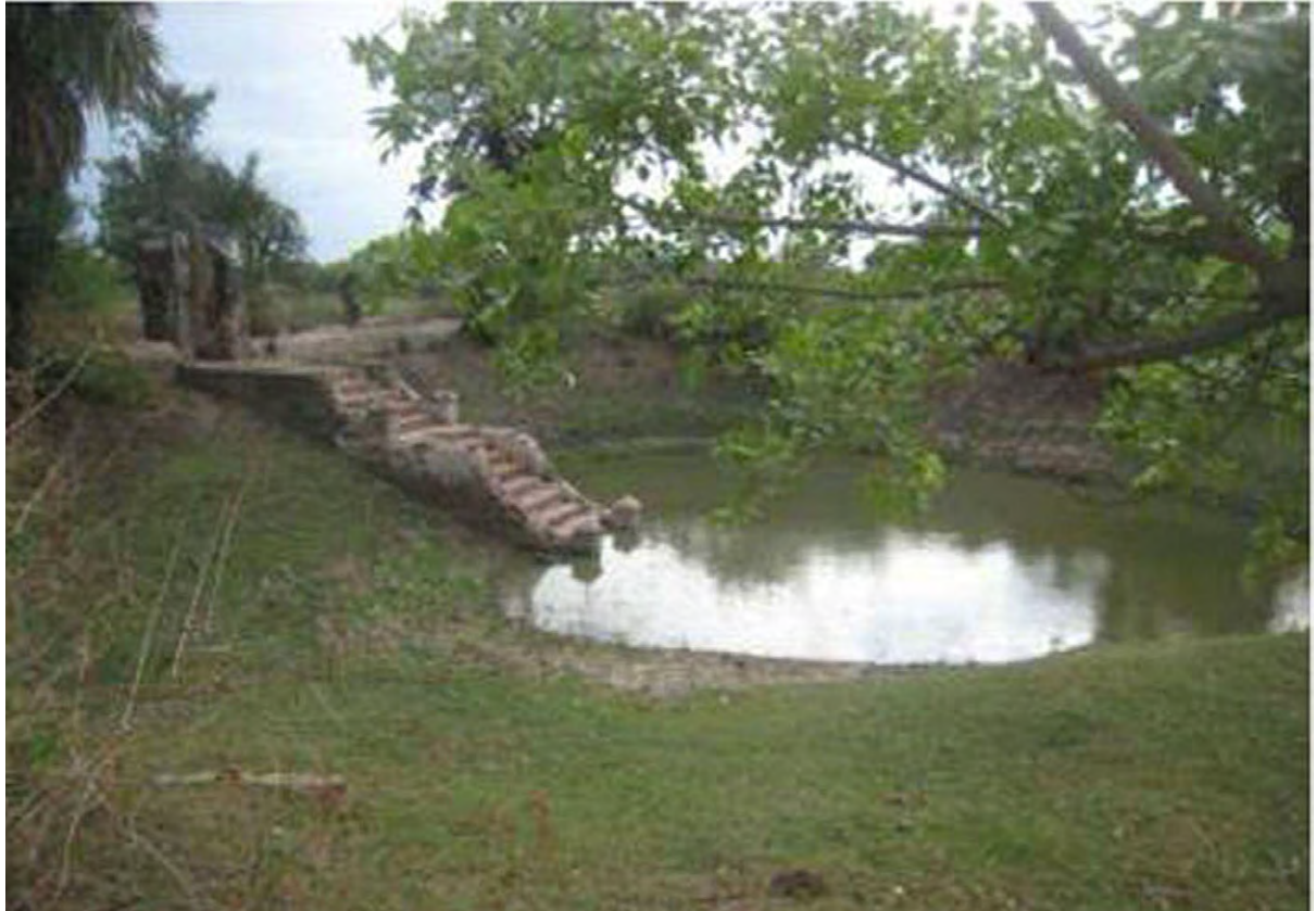
STORAGE OF DRINKING WATER AT HALIN
