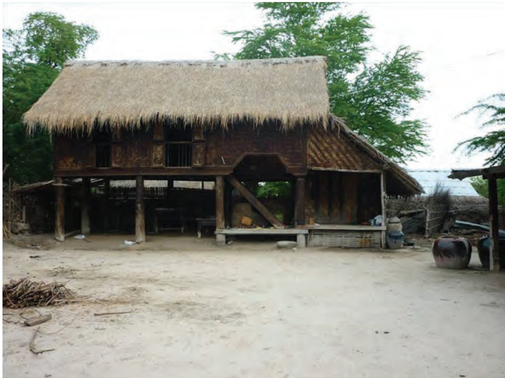
TRADITIONAL VILLAGE HOUSE WITHIN BUFFER ZONE, SHOWING TRADITIONAL CONSTRUCTION WOOD BAMBOO THATCH (HALIN)
