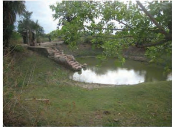
DRINKING WATER STORAGE TANK (HALIN)
