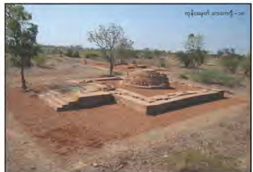
Present condition from Northeast
