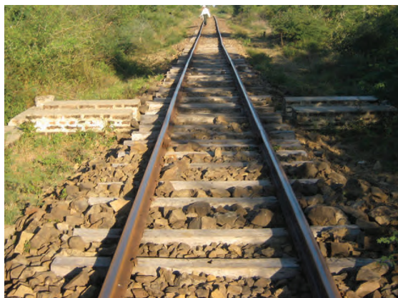
TAUNGDWINGYI-MAGWE RAILWAY LINE PASSING THROUGH BEIKTHANO PROPERTY AND BUFFER ZONE (BEIKTHANO)
