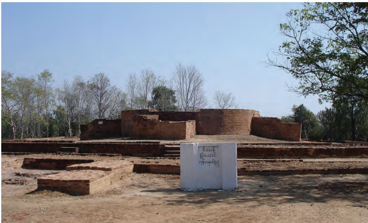
STUPA KKG-3 WITH INADEQUATE CONSERVATION WORK UNDERTAKEN IN THE PAST (BEIKTHANO)
