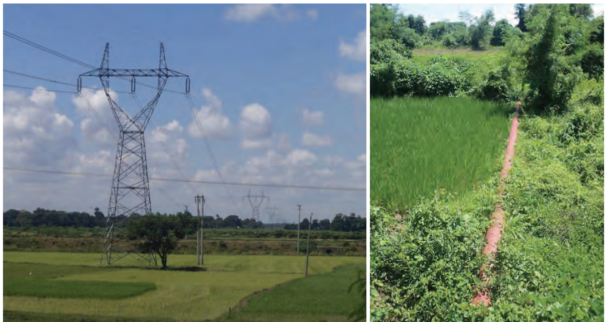
MODERN UTILITIES INFRASTRUCTURE OF POWER AND GAS PIPE LINES WITHIN PROPERTY (SRI KSETRA)
