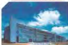
The suspended double glazing façade of the BPO building
