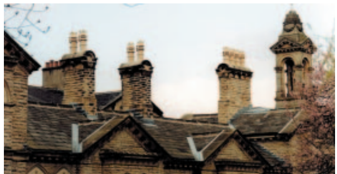
Chimney stacks and roof restorations are some of the works completed as part of a full programme of repairs funded by the City of Bradford Metropolitan District Council, English Heritage and the Heritage Lottery Fund.
