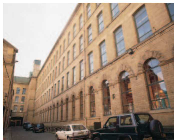
The elevation shows the north face of the main spinning mill from the inner mill yard which retains its stone setted carriageway. Original cast iron window details survive on the mill.
