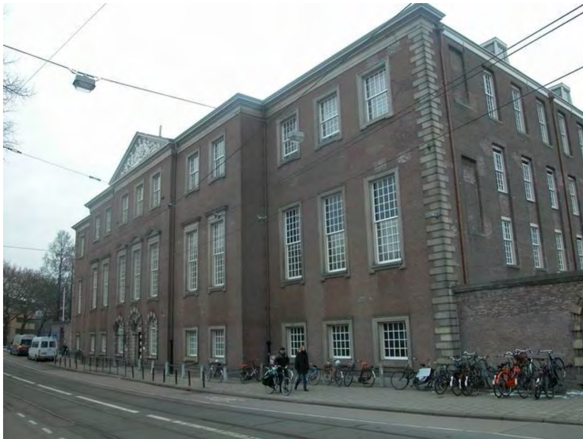
Photo C.23: View of the former Nieuwe Spinhuis en Werkhuis , seen from Roetersstraat
