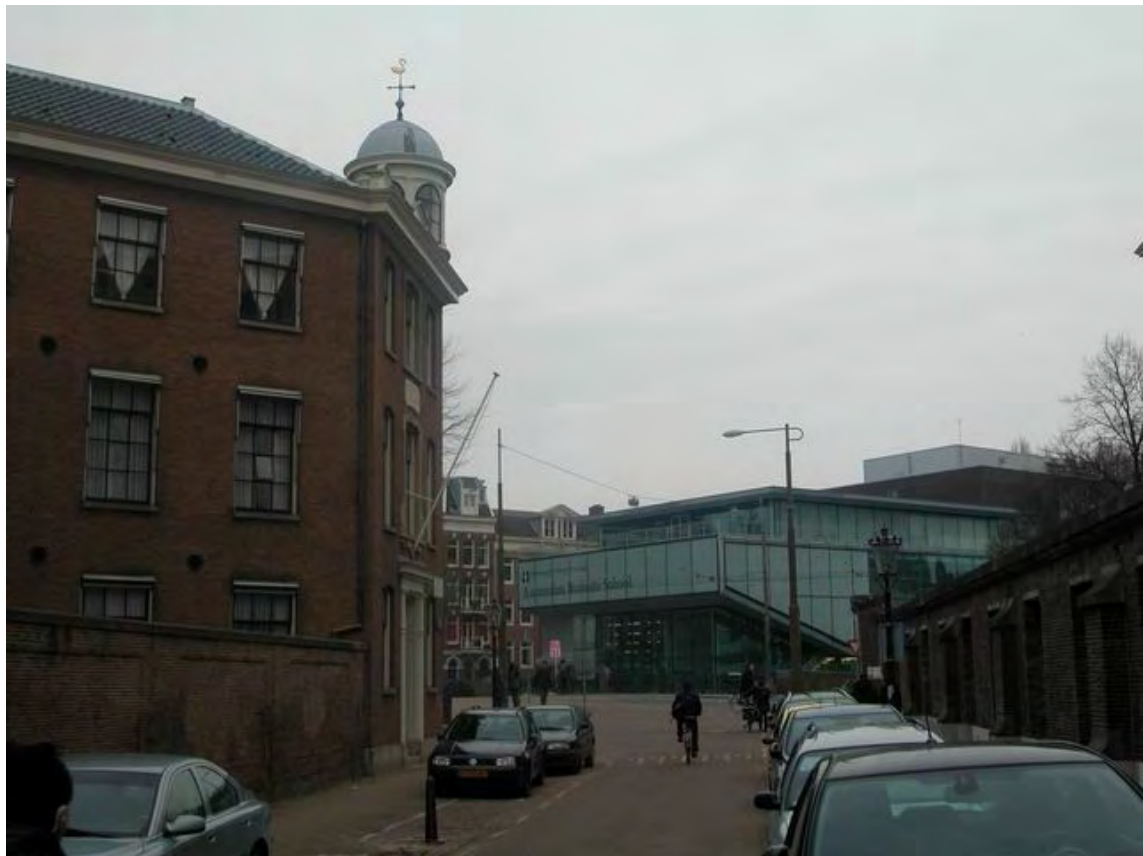
Photo C.28: View from Nieuwe Kerkstraat in direction of Roeterseiland
