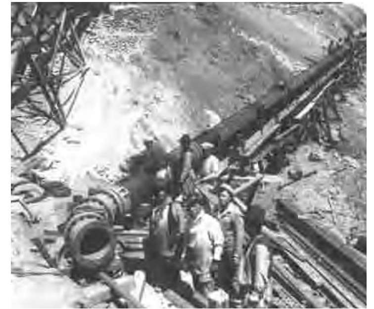
Construction of drinking water system.
