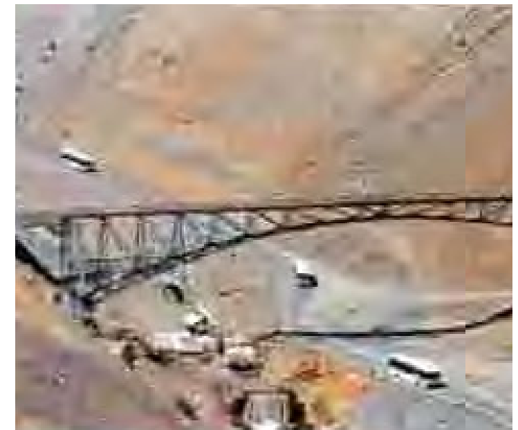
Bridge over River Coya, built in 1942.
