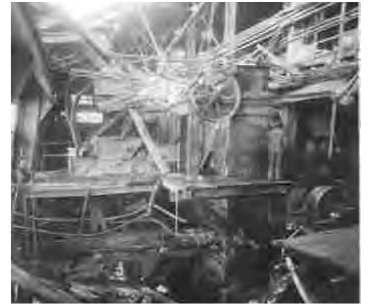
Collapse at Sewell Concentrator.
