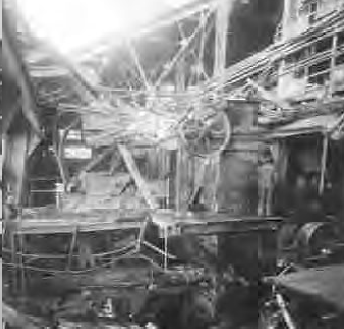
Partial destruction at Sewell Concentrator.
