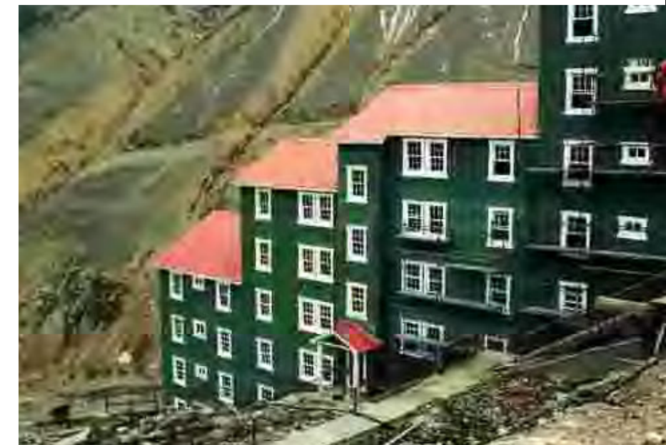
Building N°152 before and after restoration.
