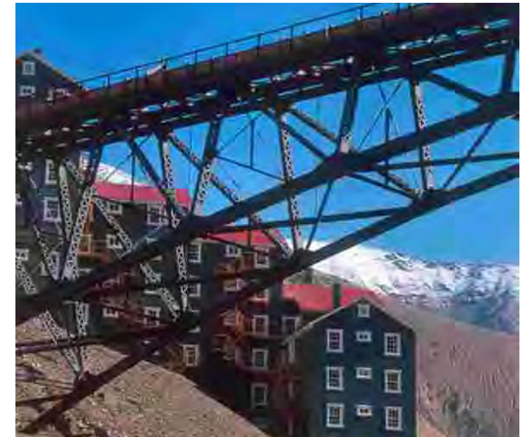
Rebolledo bridge and building N° 152.
