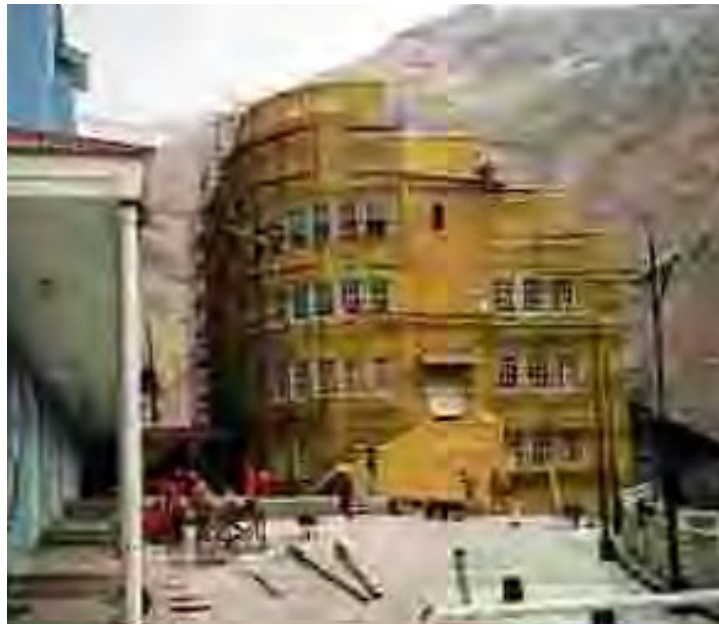
Building N° 129 under restoration.
