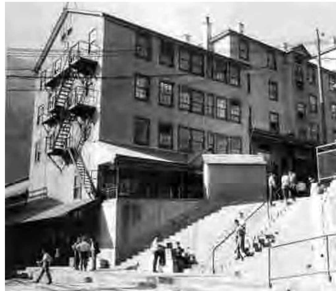
Central staircase, decade 1950.
