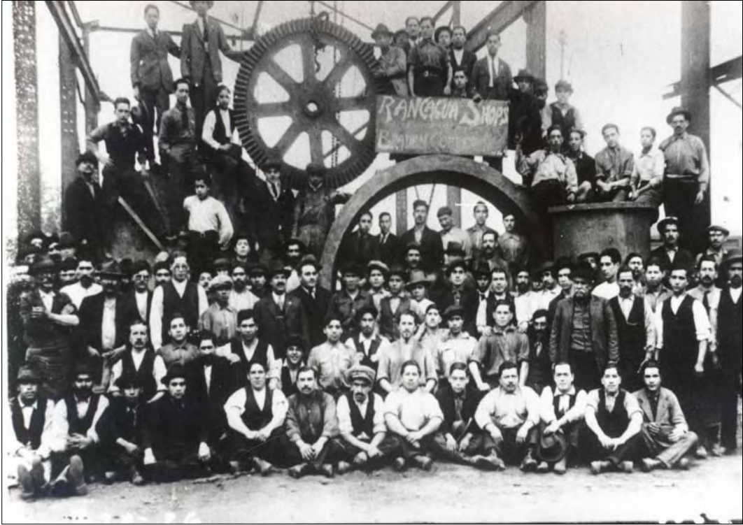
Photo N° Year Description 051 1926 Rancagua Yard workshop workers
