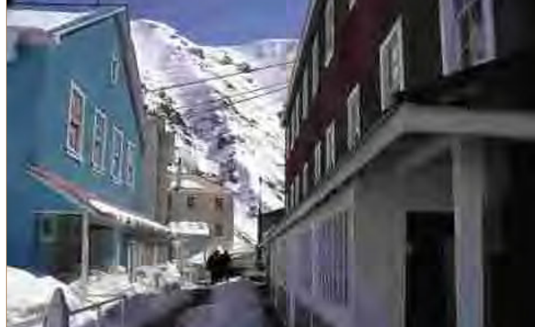
Buildings N° 107 and N° 101.
