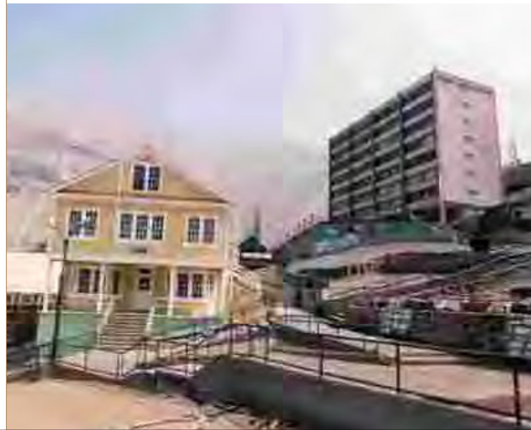
Buildings N° 102 and N° 501.
