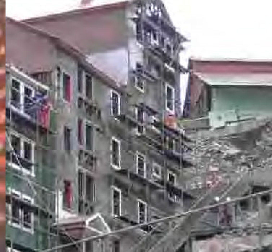
Building N° 152 during restoration.
