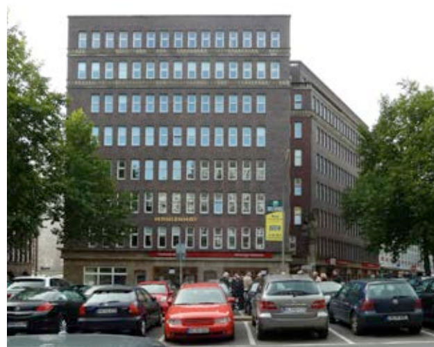
Fig. 74: The Mohlenhof, view from east
