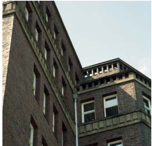
Fig. 77: Mohlenhof, northeaster corner, roof section
