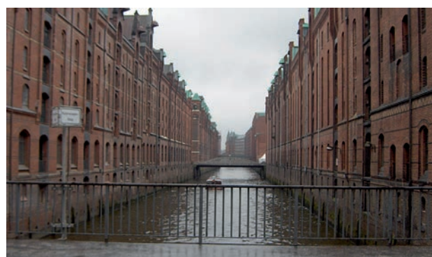
Fig. 48: Historic view of the waterways and view down Brooksfleet as it is today
