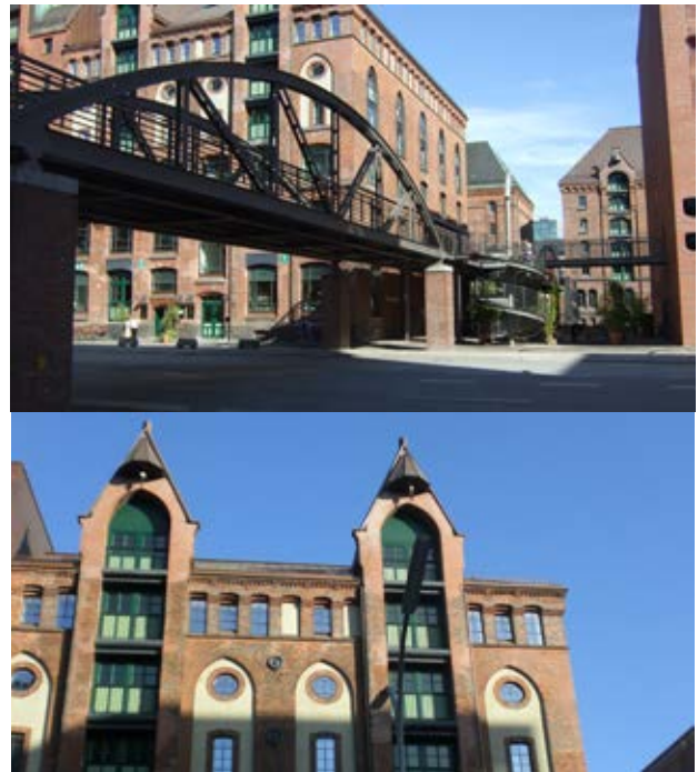
Figure 9: Kibbelstegbrücke and warehouse block N
