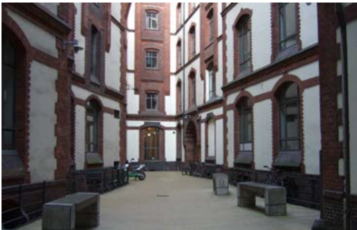
Figure 6: Courtyard of the office building at Sandtorquaihof
