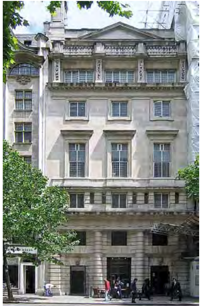
Fig. 17: Dorland House, Kingsway, London WC2, Edwin Lutyens, 1906
