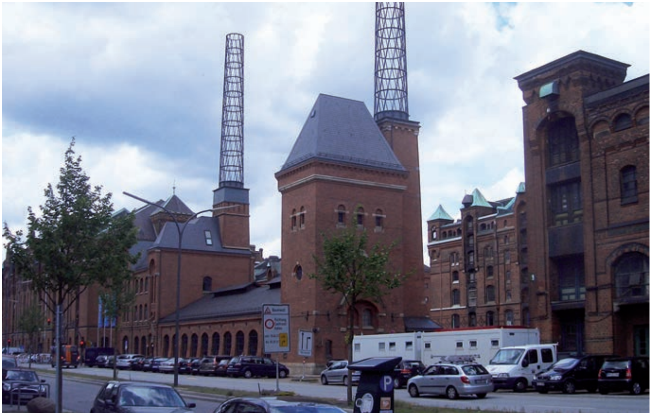
Fig. 180: The Boiler House
