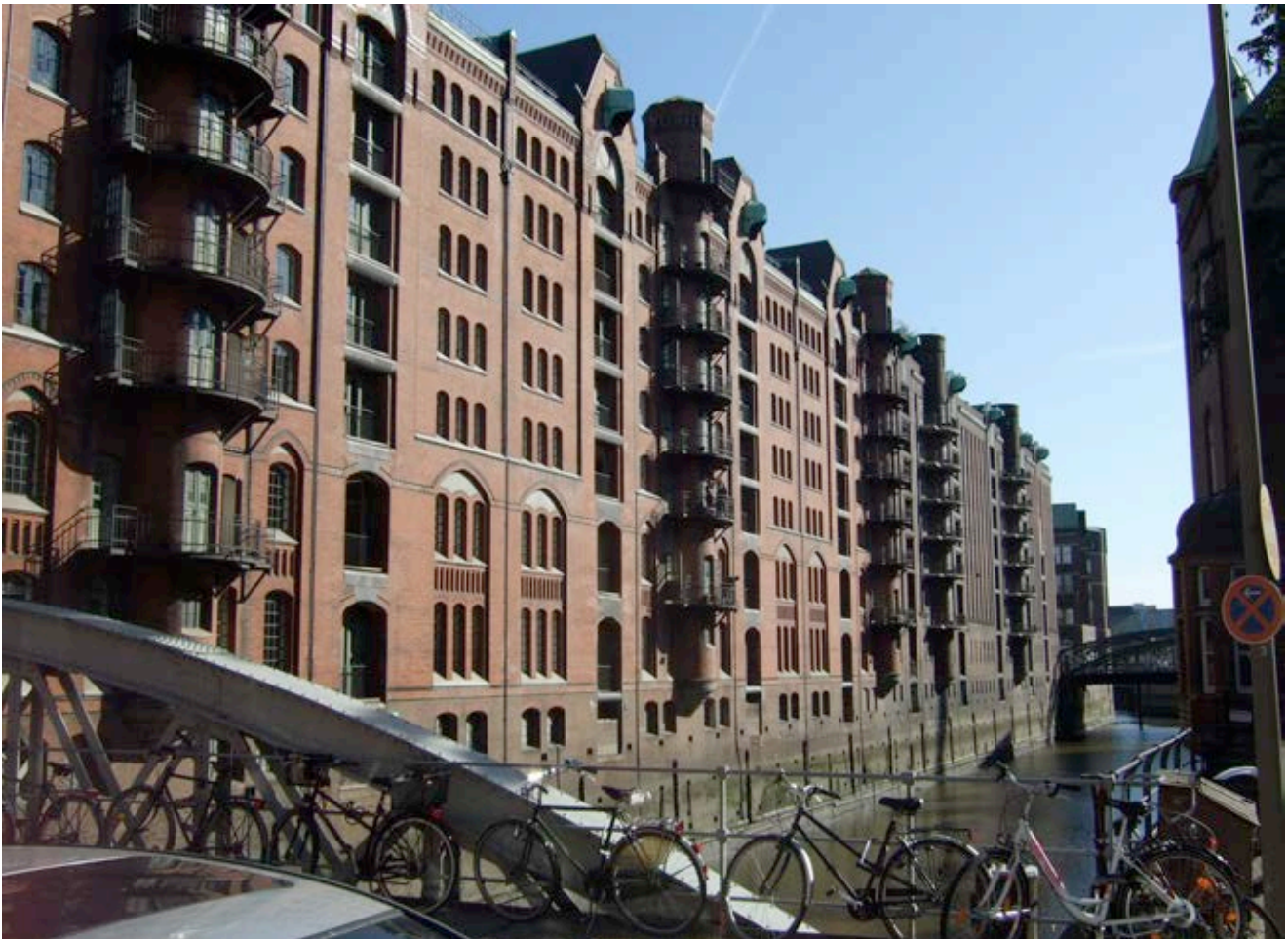
Fig. 46: Block W, view from southwest
