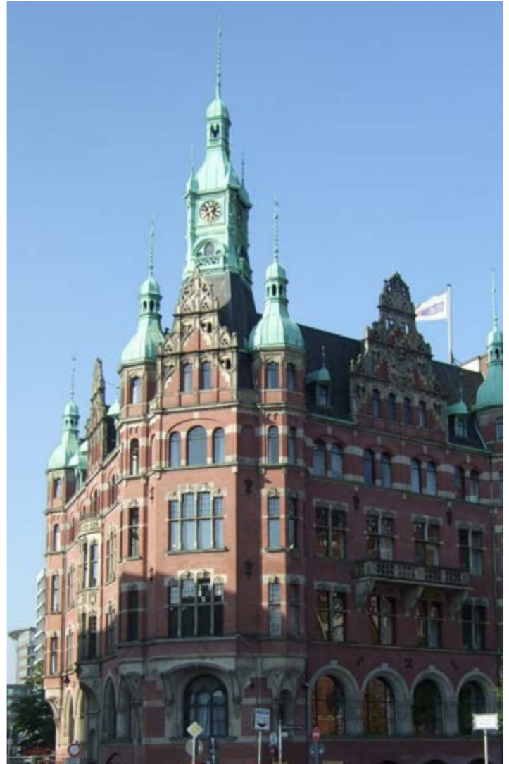
Figure 4: The Speicherstadt's "town hall"; today the headquarters of the HHLA
