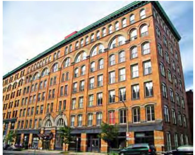
Figure 14: Jeremiah Williams & Co. Building, a fireproof wool warehouse, FPCD, built 1898; it has two more stories on its rear side
