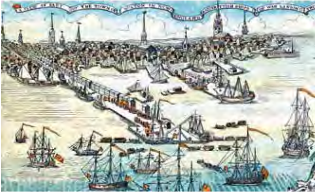
Figure 3: Warehouses on the north side of Long Wharf (center) in Boston Harbor and along other wharves
