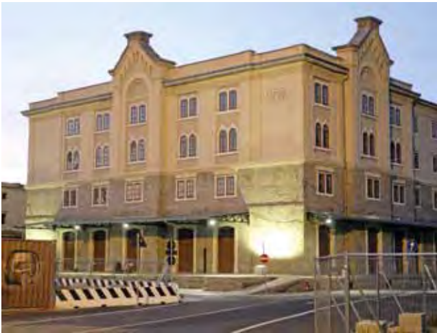
Figure 17: Trieste, Old Port, old warehouse no. 26 after restoration (2011)
