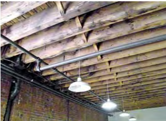
Figure 12: “Ordinary” floors of closely-spaced joists and bridging
