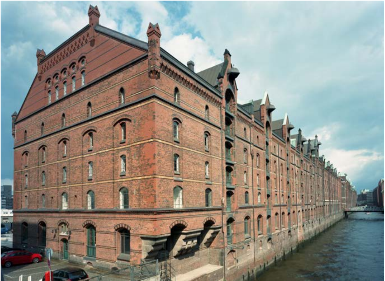
Fig. 23: Block D, view from southwest
