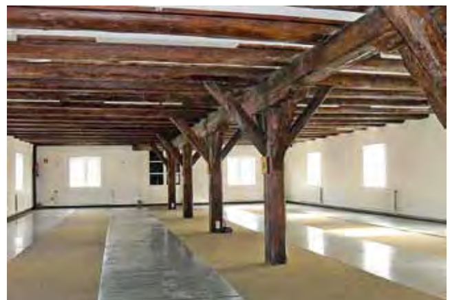
Abb. 5: Bremen, Vegesack, Thiele-Speicher um 1800, innen
