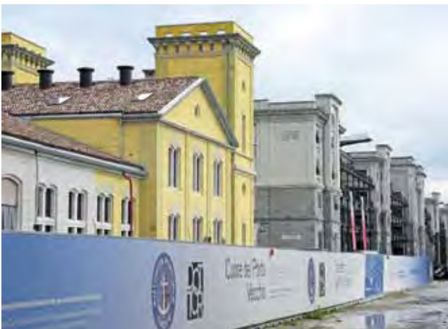
Figure 18: Trieste, Old Port, hydraulic power plant, works for restoration (2011)
