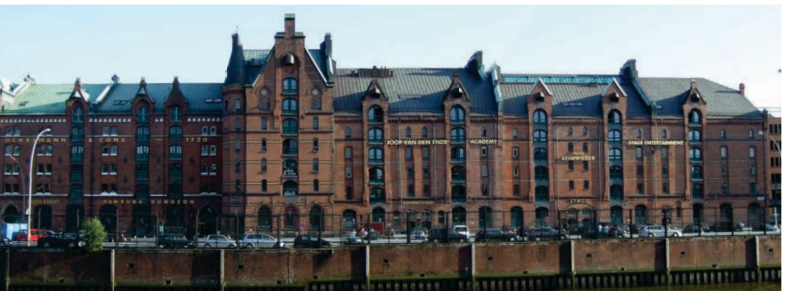
Figure 72: View of warehouse block D from the north
