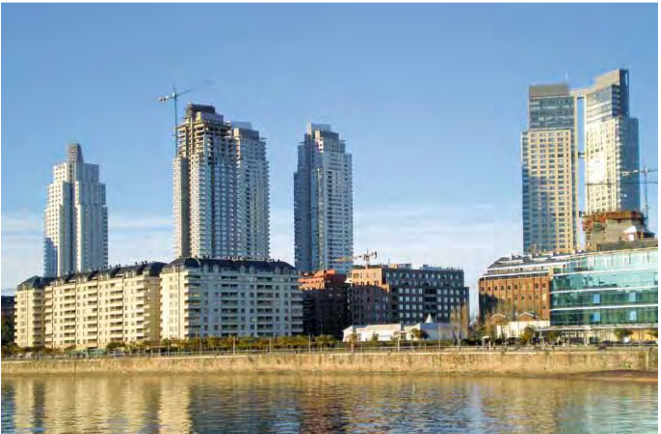
Figure 11: Contrast between first and second stages of construction of new buildings on the eastern bank
