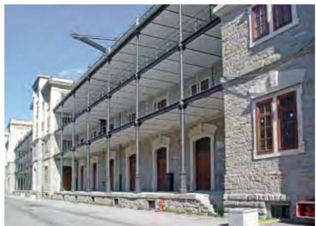
Figure 16: Trieste, Old Port, old warehouse no. 26 after restoration (2011)
