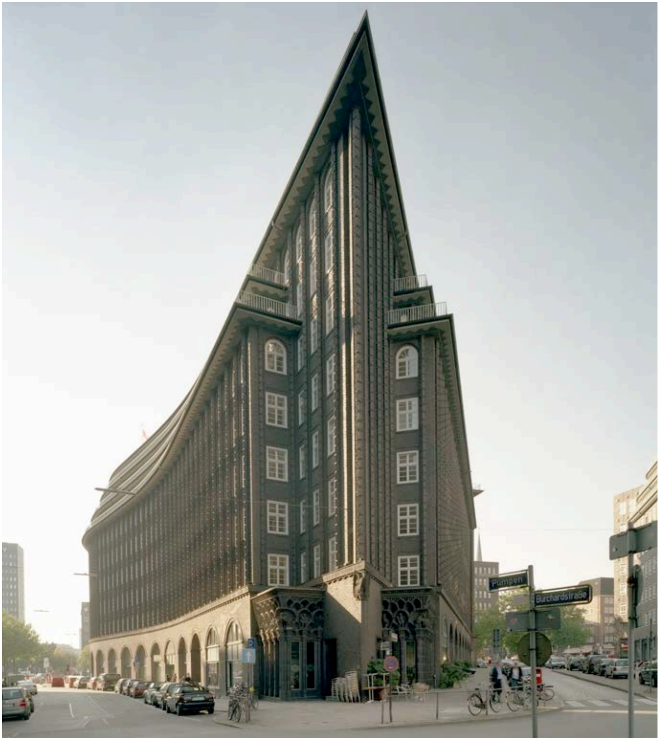
Fig. 52: The Chilehaus, view from east
