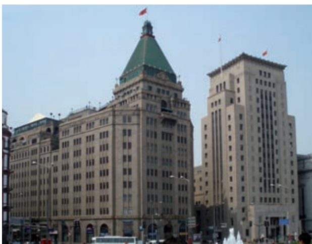
Fig. 158: Shanghai, Sassoon House (left, today "Peace Hotel") and Bank of China Building (Design: Tsuyee Pei, 1934), 2002
