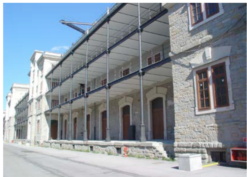
Fig. 146: Trieste, Porto Vecchio, warehouse district, warehouse 26 after the redevelopment, 2011
