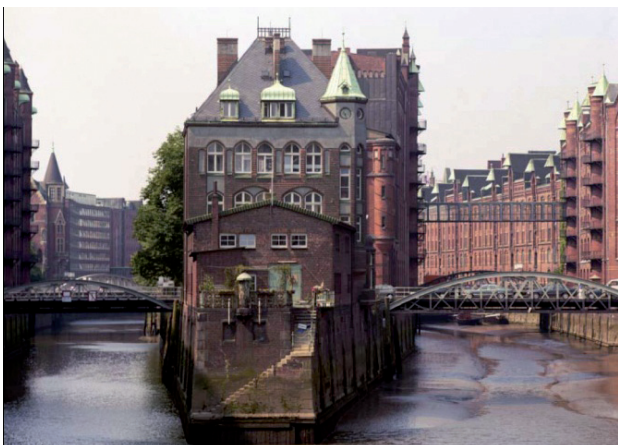
Fig. 64: View of the "Wasserschlosschen" (Little Water Castle)
