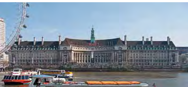
Fig. 8: ex County Hall 1911–22 and 1931–33, Ralph Knott, Westminster Bridge SE1 Built as headquarters of London County Council, now hotel. Island site with frontage to Thames; six storeys plus two in huge roof, planned round multiple light-wells. Steel frame, Portland stone cladding
