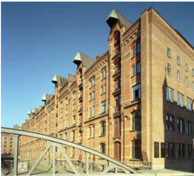
Fig. 102: Repaired block P with new eastern gable, around 2010
