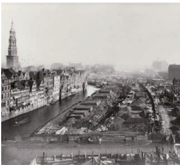
Fig. 83: Demolition works on the Brookinseln around 1884
