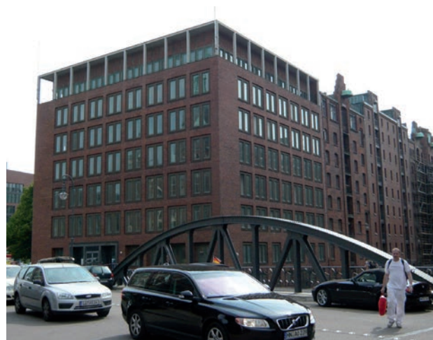
Fig. 24: Speicherstadt, new eastern section block R
