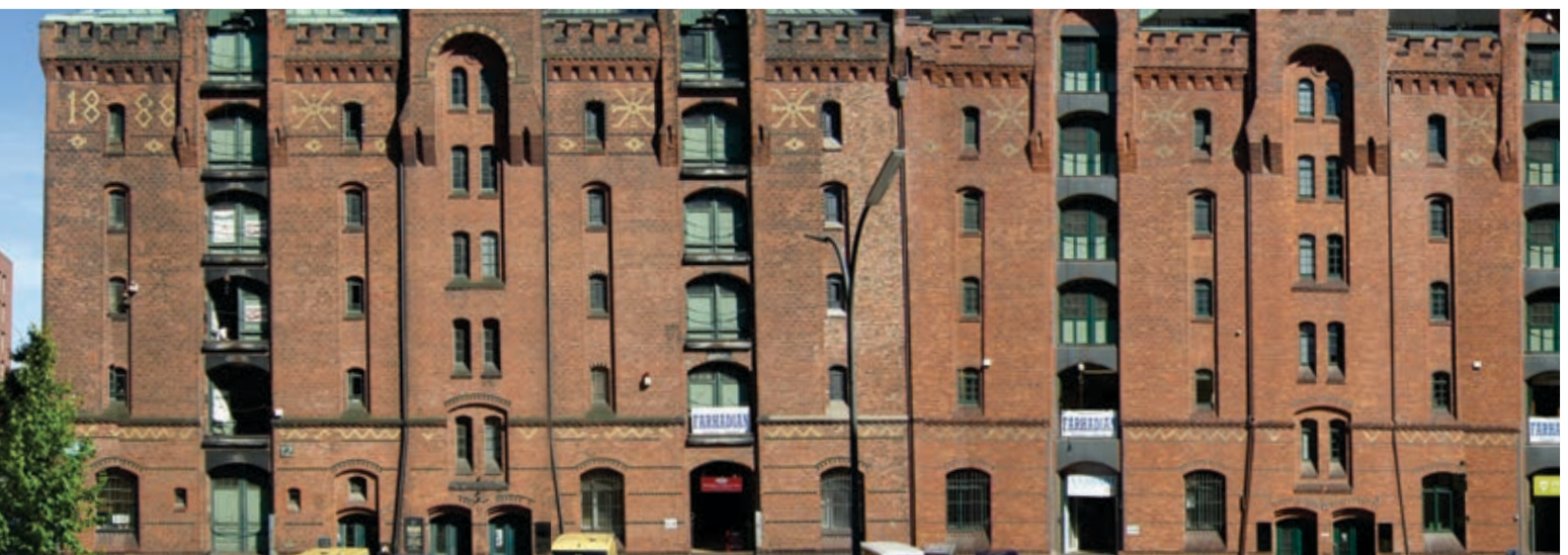
Figure 81: View of warehouse block L from the south
