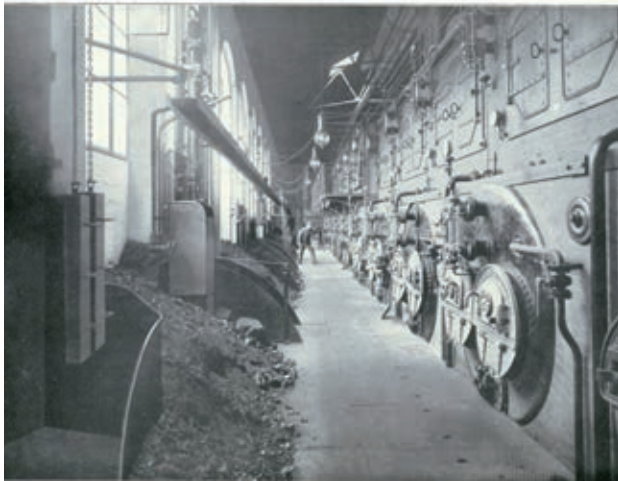
Fig. 92: Steam Boiler Complex in the Central Power House, around 1890
