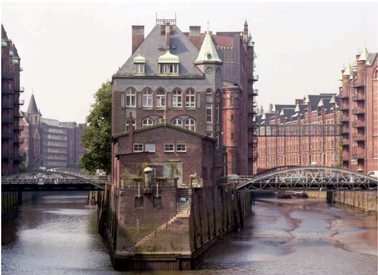
Fig. 176: View of the "Wasserschlosschen" (Little Water Castle)
