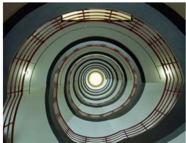
Fig. 73: Sprinkenhof, staircases of section one at the Burchardstrasse
