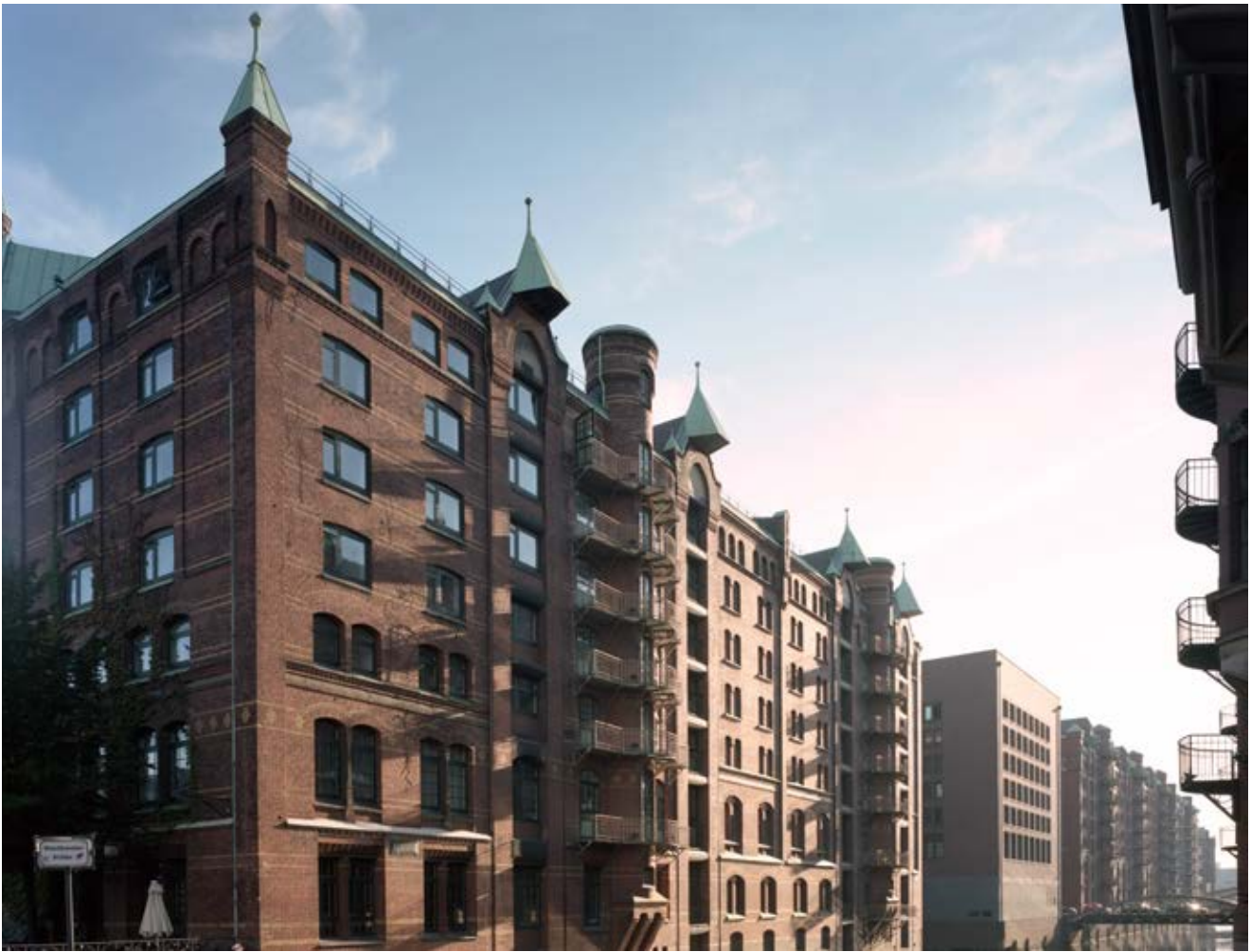
Fig. 39: Block S, view from southwest
