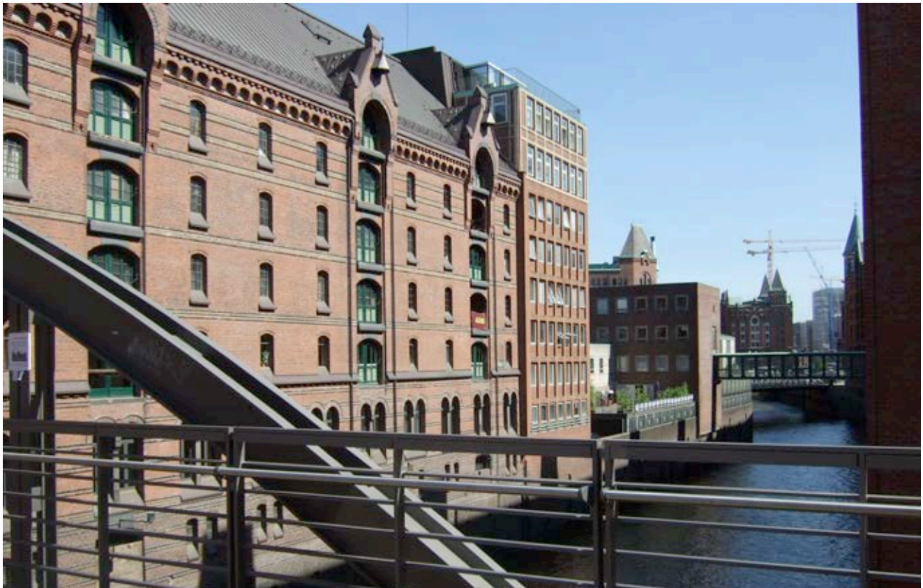
Fig. 29: Block G, view from southwest
