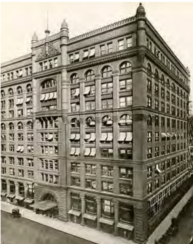
Figure 5: Exterior, The Rookery (1885–1888), Chicago, Burnham & Root
