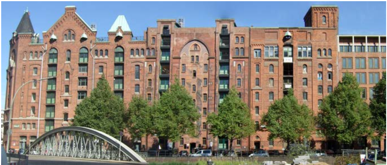
Fig. 37: Block Q/R, view from south
