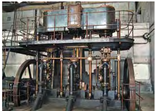
Figure 9: Trieste, Old Port, hydraulic power plant, (1890) machine Breitfeld & Danek – Karolinental – Prag
