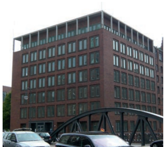
Fig. 38: Block R, view from east
