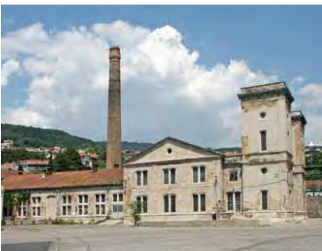
Figure 7: Trieste, Old Port, hydraulic power plant
