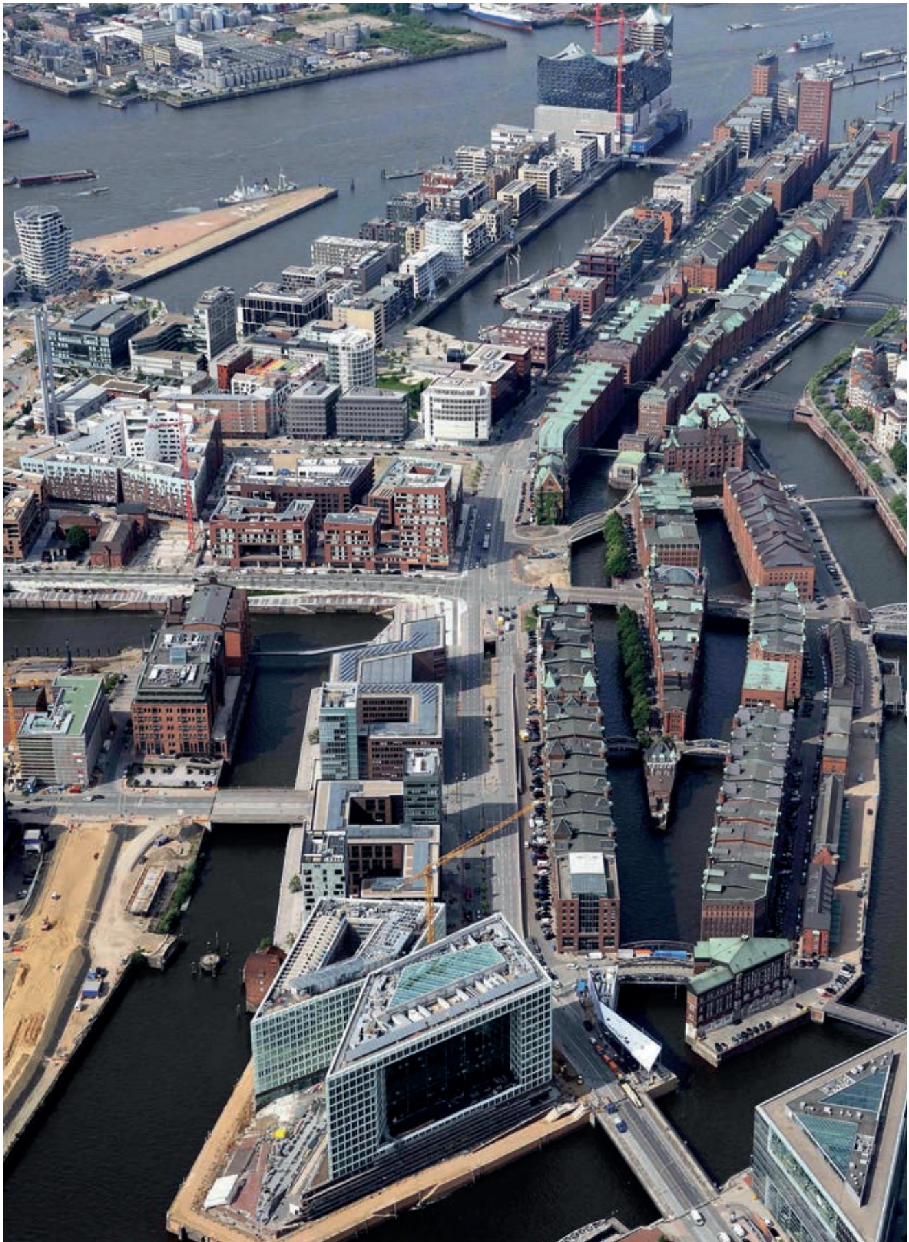
A: Aerial view of the Speicherstadt from east
