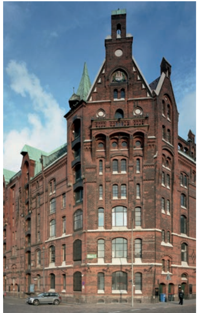
Fig. 25: Block E, view from Northwest
