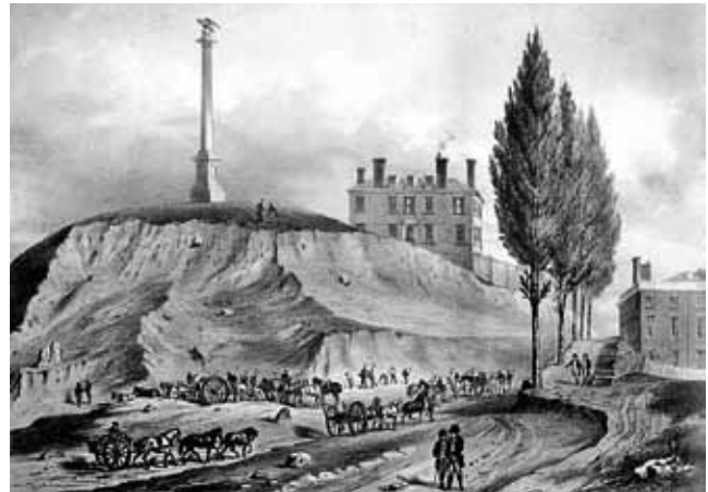
Figure 5: Cutting down Boston's Beacon Hill ca 1811 to fill the Mill Pond
