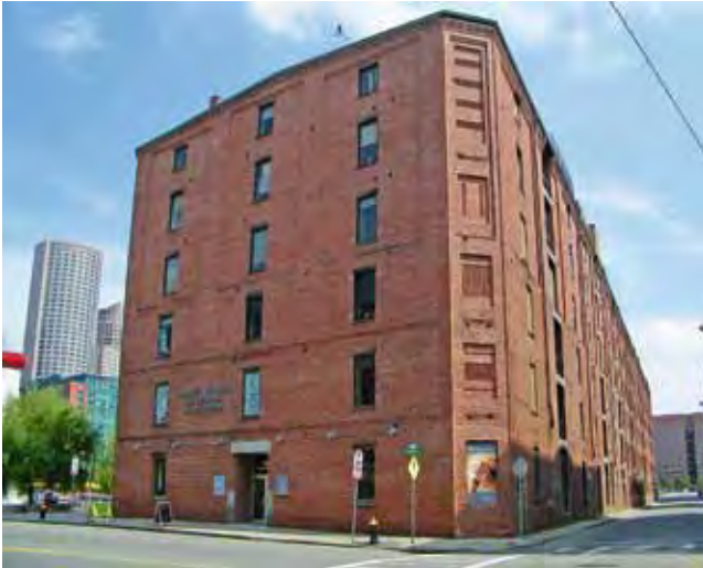
Figure 11: Patterned brick at the corner does little to relieve the plainness of the Atlas Stores, FPCD, the first part of which was built in 1890 by BWCo
