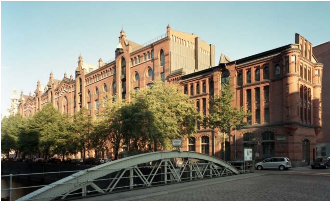
Fig. 42: Block U from southeast with electric substation
