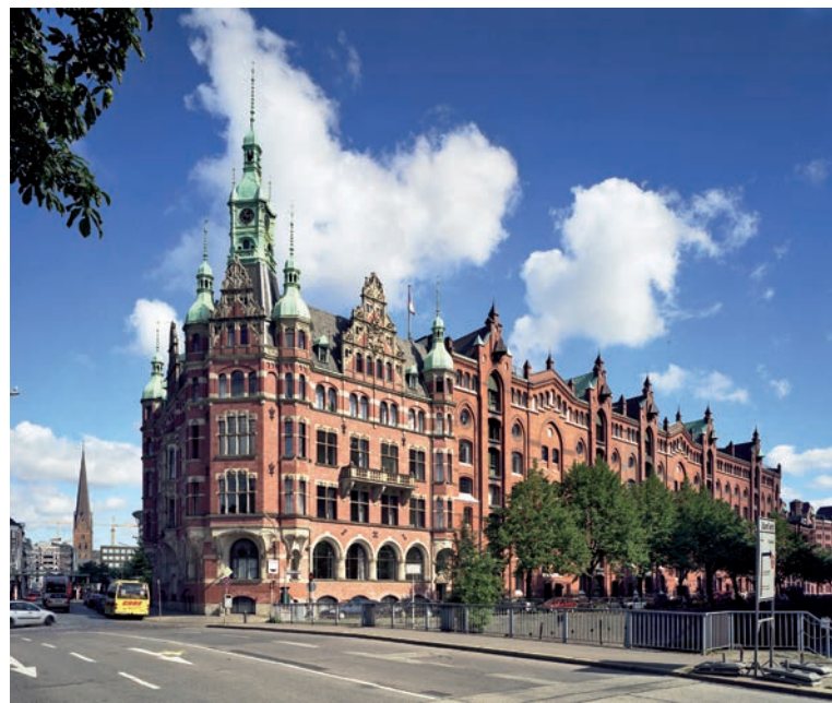
Fig. 43: View from the „Town Hall“ of the Speicherstadt on the Domplatz to the St. Petri Church
