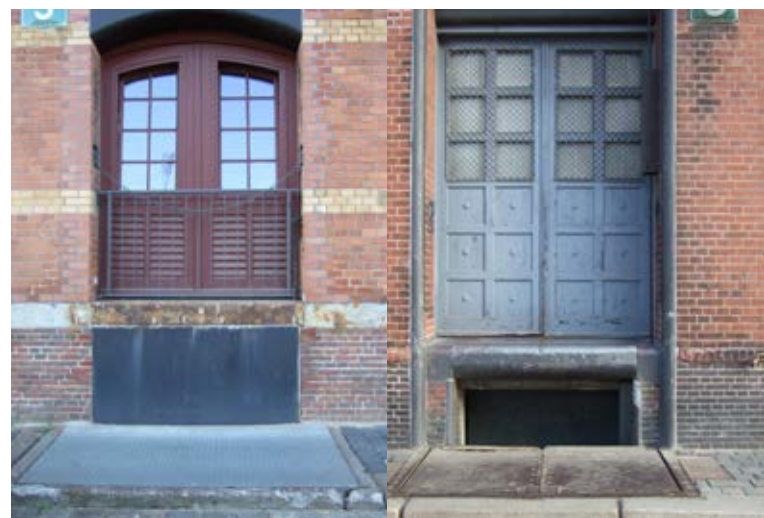
Figure 30: Sealing of a basement hatch with concrete
