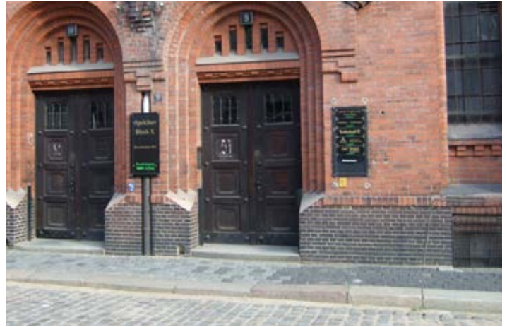
Figure 27: Strip of cobble setts in front of the warehouse buildings
