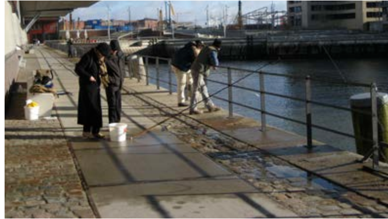
Figure 57: New railing at Sandtorhafen
