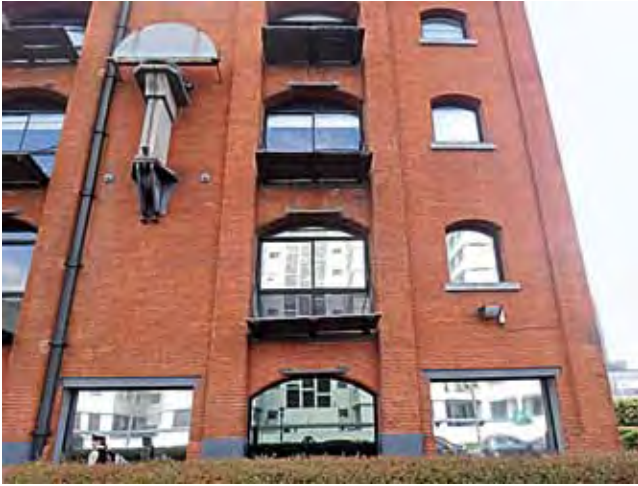
Figure 9: Detail of restored façade
