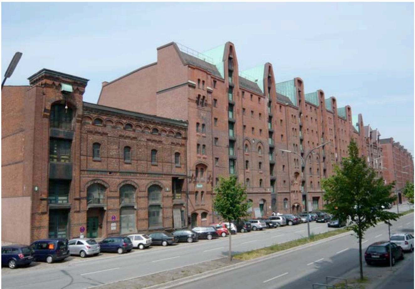
Fig. 27: Block M/N with Central Power House, view from southwest
