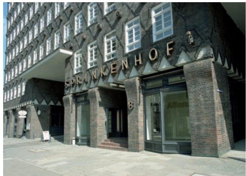
Fig. 67: Sprinkenhof, first section, detail
