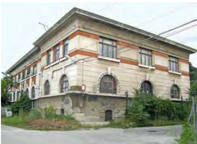
Figure 13: Trieste, Old Port, power plant
