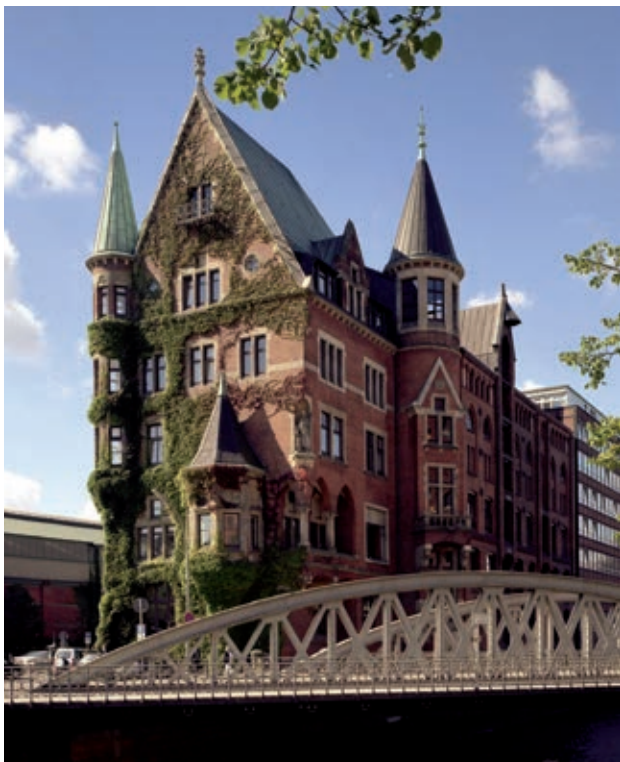
Fig. 34: Block O with the first administration building of the HFLG (Hamburg Free Port Warehouse Association)
