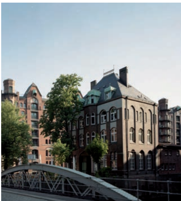
Fig. 48: "Little Water Castle", view from southwest
