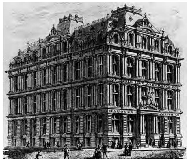
Figure 2: Equitable Building, New York City, by Gilman & Kendall with George B. Post, 1870
