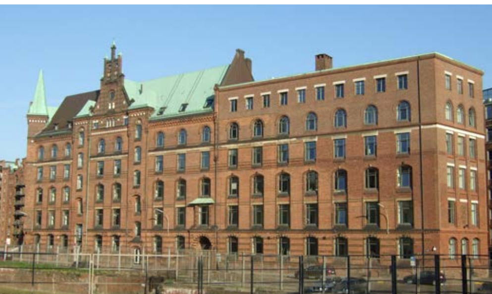
Figure 79: View of warehouse block H from the north
