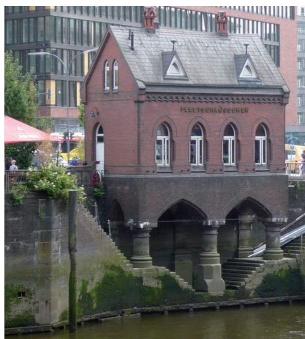
Fig. 17: Manned Fire Alarm Station (Fleetschlosschen)
