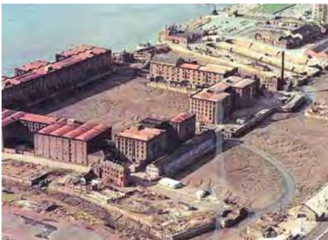
Figure 4: Albert Dock circa 1980, prior to comprehensive restoration
