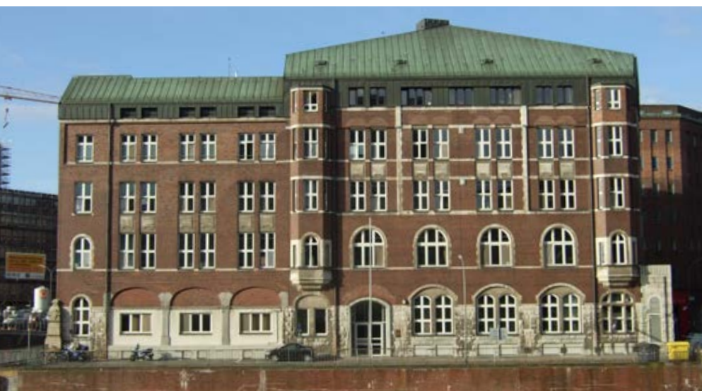
Figure 106: View of the Customs Head Office from the north-east
