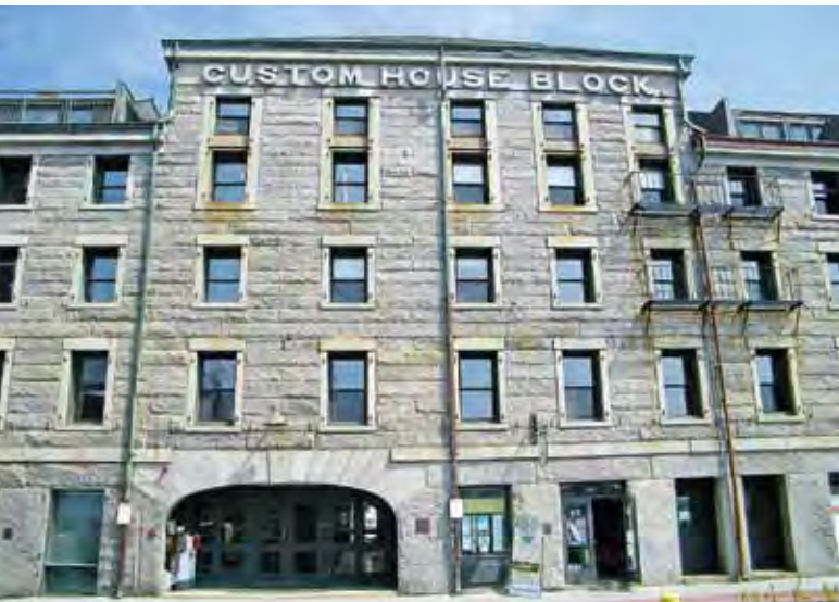
Figure 7: Granite walls, and monolithic piers and lintels, of the Custom House Block on Long Wharf, completed 1848
