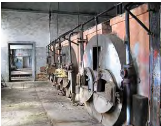
Figure 12: Trieste, Old Port, the boiler room
