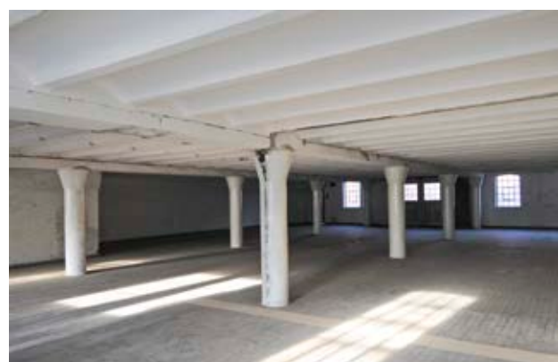
Fig. 19: Construction forms at the Speicherstadt: a.) Iron construction from the first construction phase; b.) Wood Construction from the second and third construction phase; c.) Cast iron pillars with metal sheathing from the third construction phase
