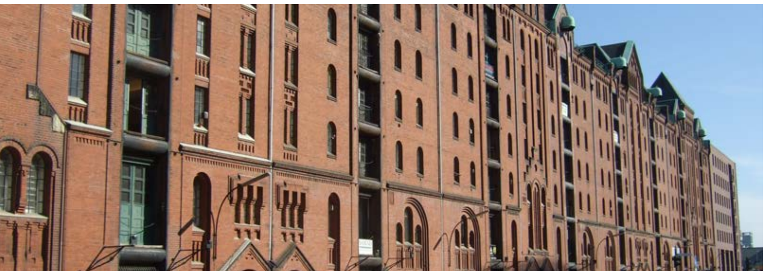
Figure 104: View of warehouse block X from the south
