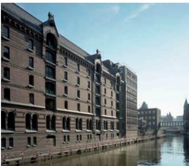
Fig. 104: Block G with new building at the eastern fire section, 2012
