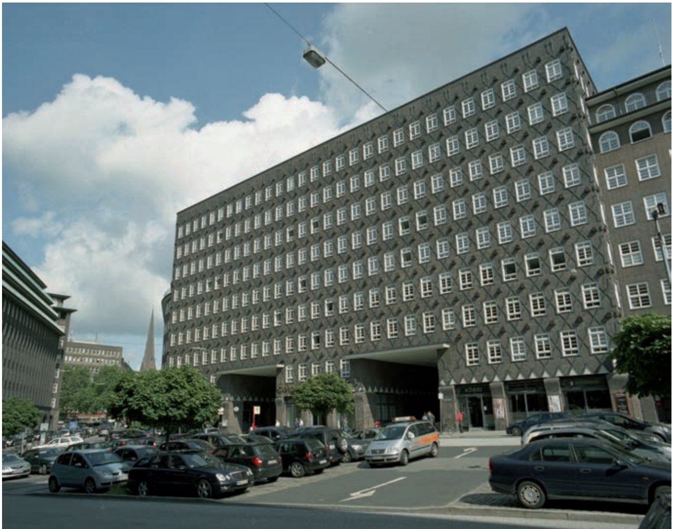
Fig. 66: Sprinkenhof, first section, view from southeast
