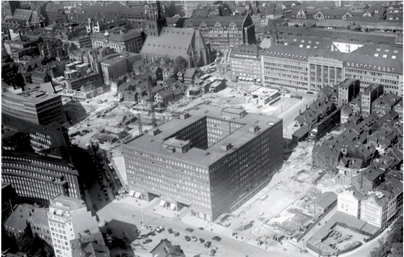
Fig. 123: Aerial view with Sprinkenhof, around 1930
