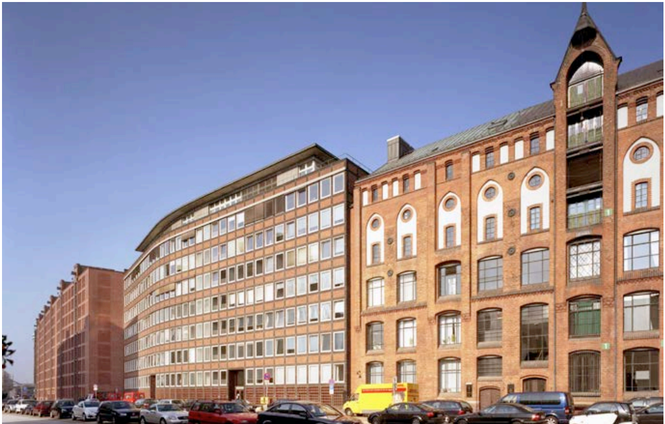
Fig. 33: Block O, view from southeast
