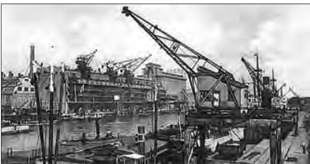
Figure 10: Warehouse Jobsveem, constructed in 1912
