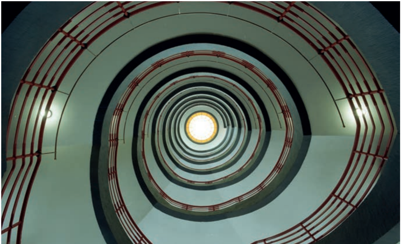
L: The Sprinkenhof, staircase of section one
