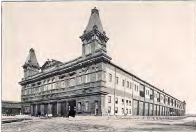
Figure 8: New Municipal Pier at Vine Street, Shore Front
