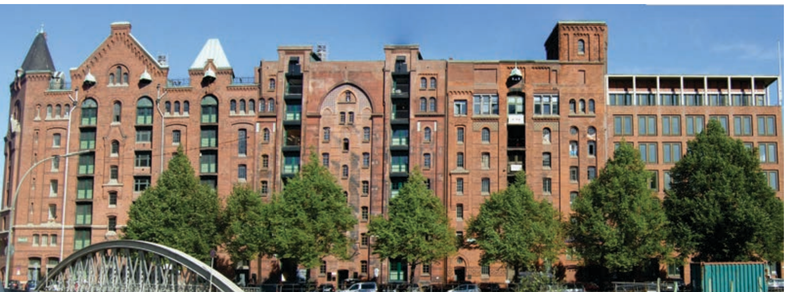
Figure 90: View of warehouse blocks Q and R from the south
