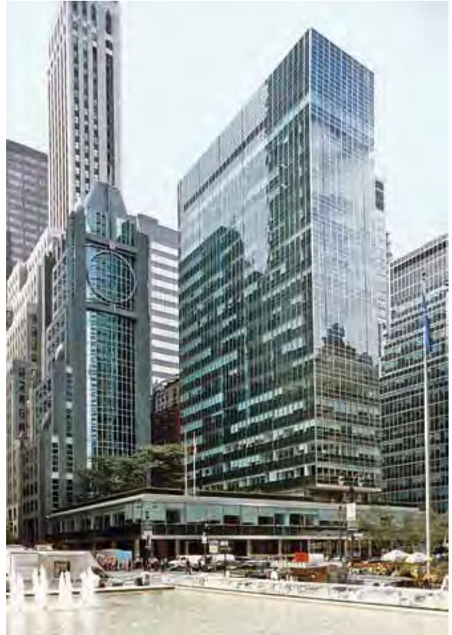
Figure 11: Lever House, New York City, Gordon Bunshaft for Skidmore Owings & Merrill, 1949–52
