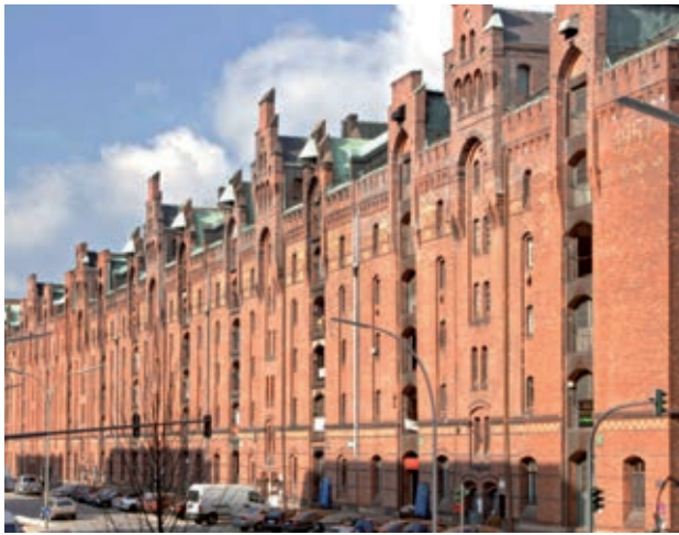
Fig. 101: Repaired block L, 2007
