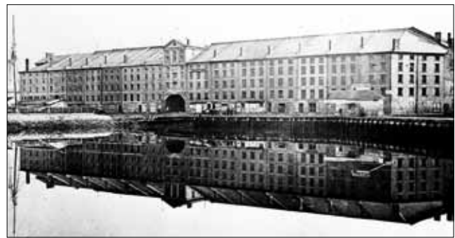
Figure 6: India Wharf warehouses, built 1805–ca 1807: although consisting of many separate stores, the stores were grouped and treated as one building
