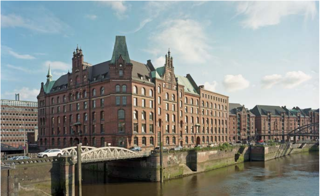
Fig. 35: Block H, view from northeast
