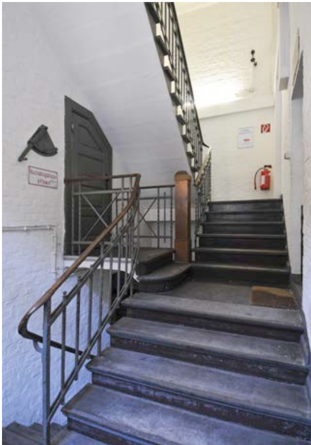
Fig. 21: Staircase, block V, third construction phase
