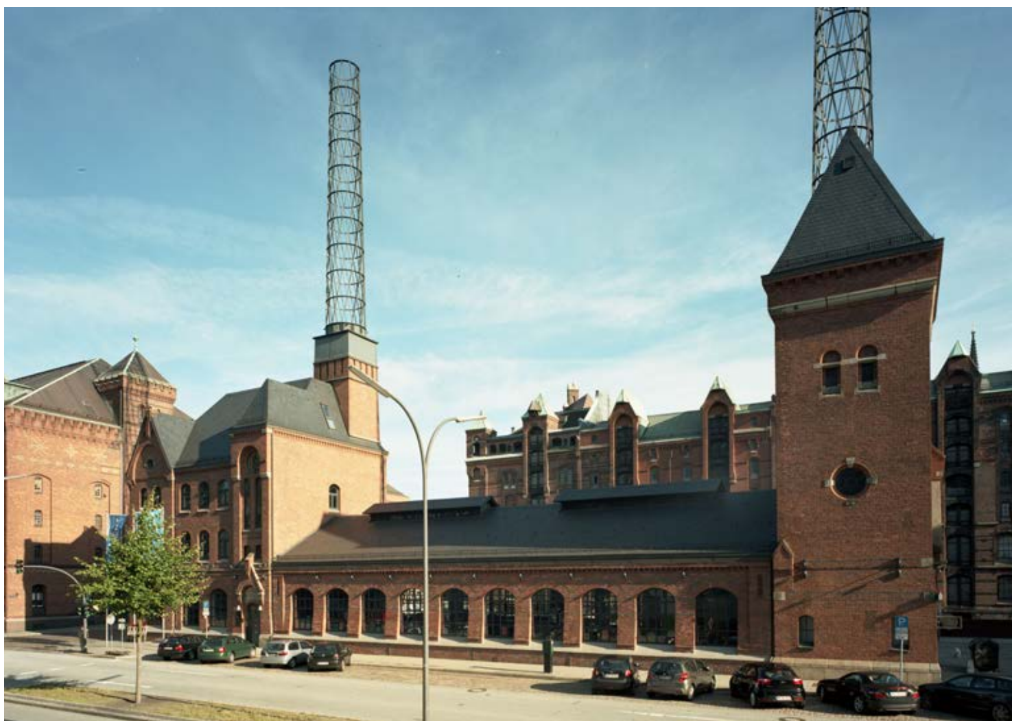
Fig. 26: Boiler House, view from south
