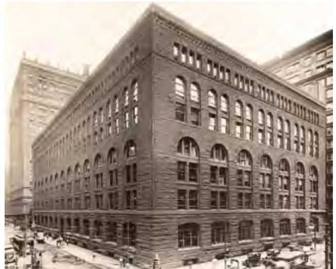
Figure 2: Exterior, Marshall Fields Wholesale Store (1885–87), Chicago, H. H. Richardson (demolished)
