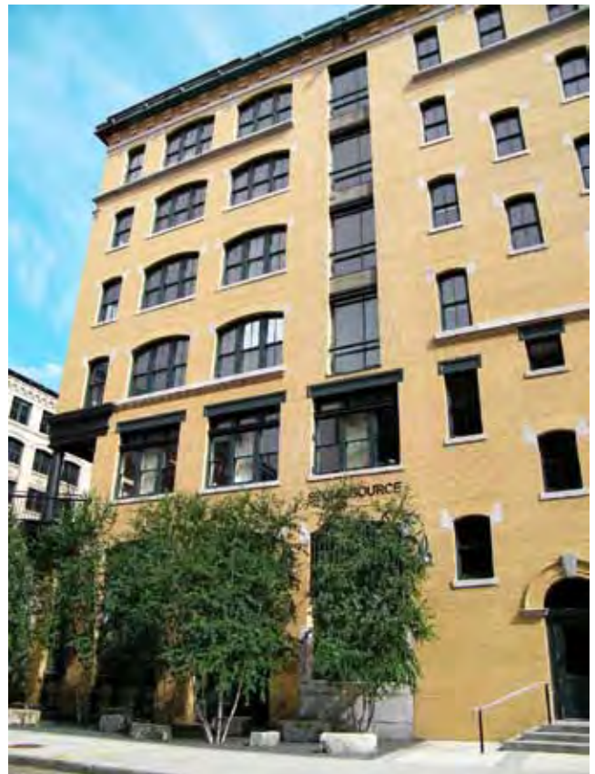
Figure 15: A tier of loading doors that has been changed to windows after renovation; Dwinell-Wright Co. Building, FPCD, built 1904
