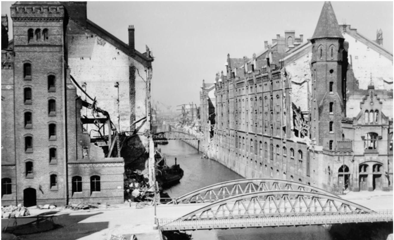
Fig. 100: Damage at block L (left) and at block D (right), 1944
