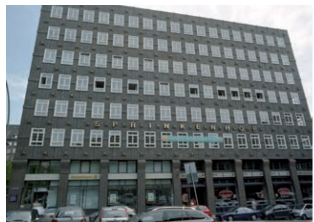
Fig. 70: Sprinkenhof, second section, view from west
