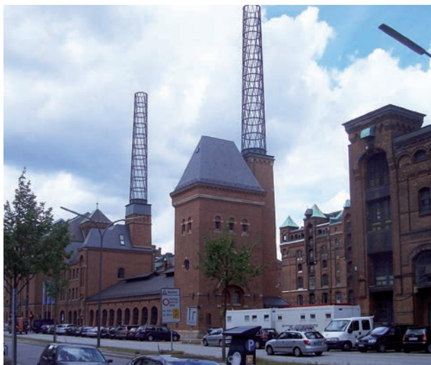
Fig. 68: The Boiler House
