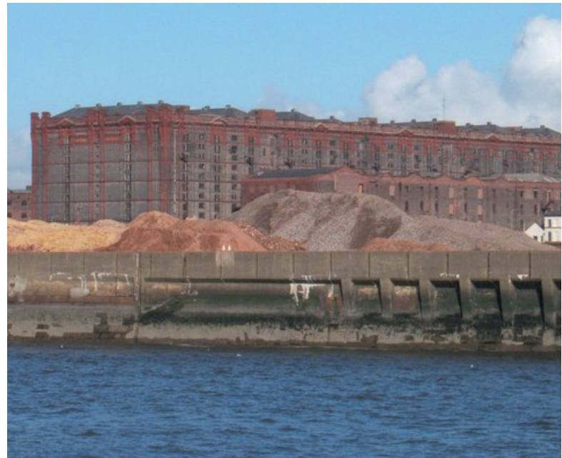
Fig. 139: Liverpool, Stanley Dock Tobacco Warehouse, 2008
