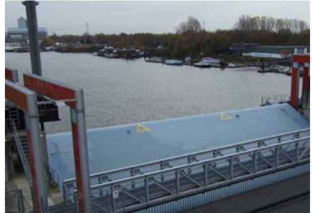
Figure 16: Barrage at Billwerder Bucht
