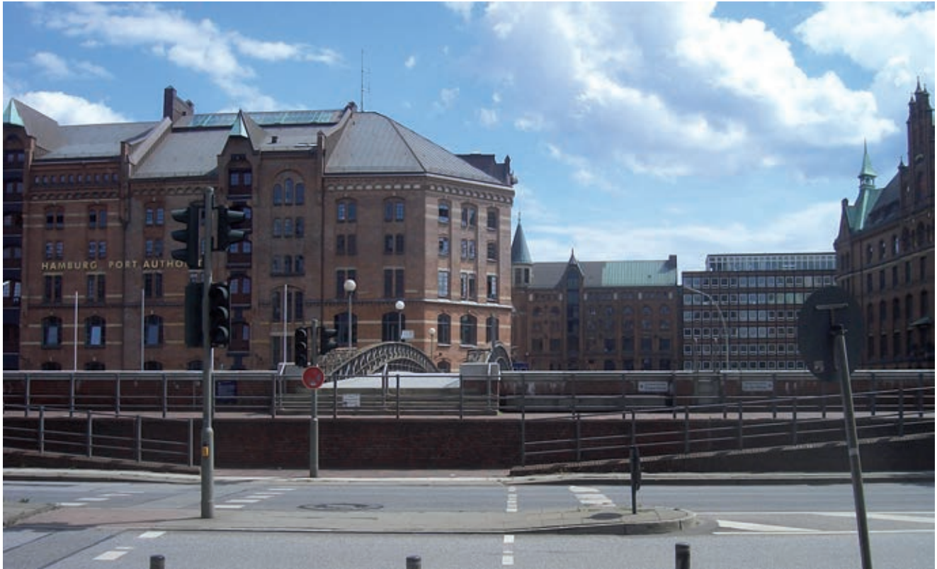
Fig. 164: Existing flood defences along the Customs Canal and their utilisation as viewing points
