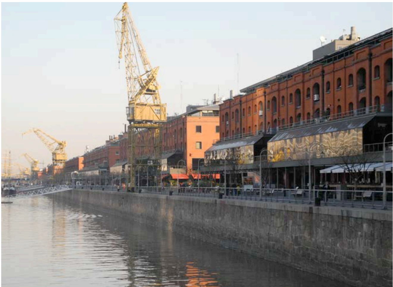
Fig. 149: Buenos Aires, Puerto Madero, modified warehouses, 2012
