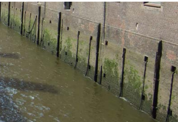
Figure 19: Quay walls underneath warehouse blocks D and L
