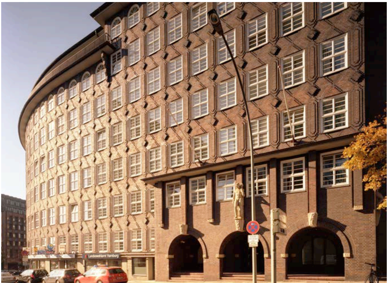
Fig. 71: Sprinkenhof, third section, view from northeast with the entrance at the Johanniswall
