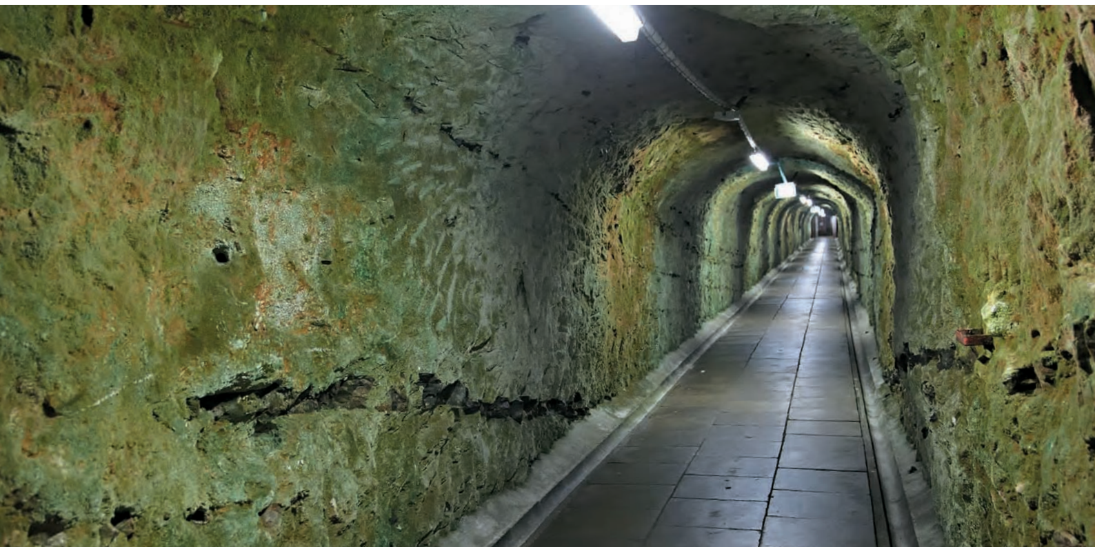
Figure 39. The subterranean Cold War fortress Stevnsfort with 1.6 km of tunnels excavated into the limestone.
