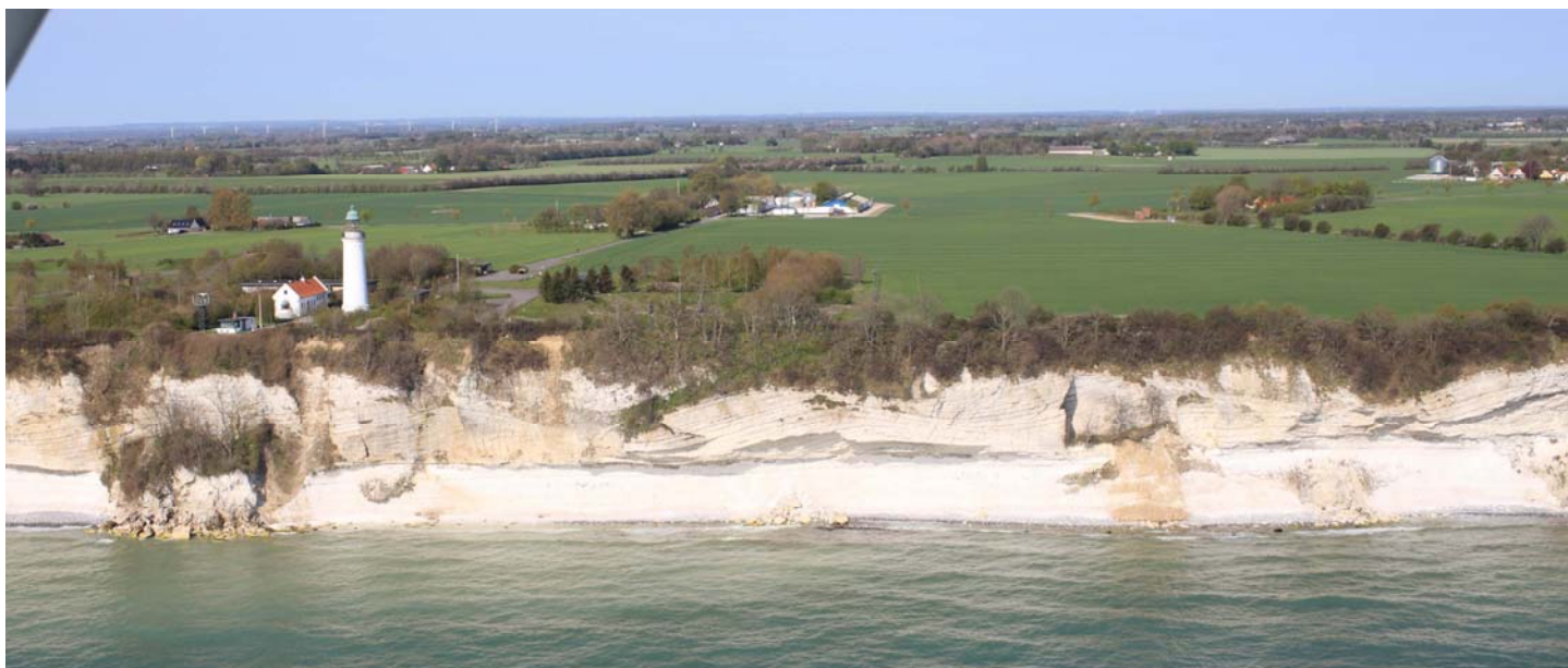
Figure 12. Photo of the cliff-fall and the large overhang at Stevns Fyr. The lighthouse is located at the highest point along Stevns Klint, 41.5 m a.s.l. Below and north of the lighthouse the rectangular shaped small limestone quarries can be seen. Note that under the substantial overhang a small pile of blocks indicate a rock-bedding exfoliation of the roof below the overhang. This type of erosion contributes to the decrease in the thickness of the overhang, which decreases its strength and thus increases its tendency of a cliff-fall (or cliff-slide).
