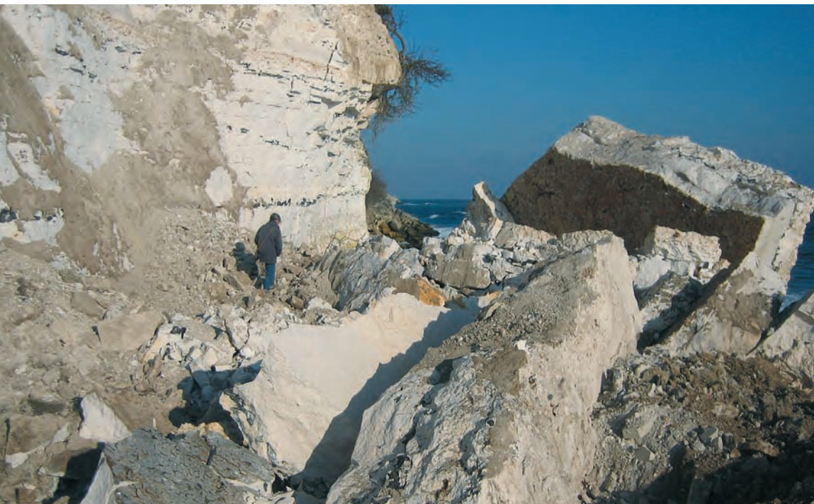
Blocks from rock fall, November 2011.
