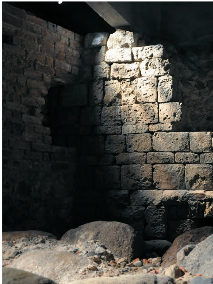
Figure 33. Building stones from Stevns Klint in the ring walls of the castle built in 1167 by the founder of Copenhagen, Bishop Absalon.
