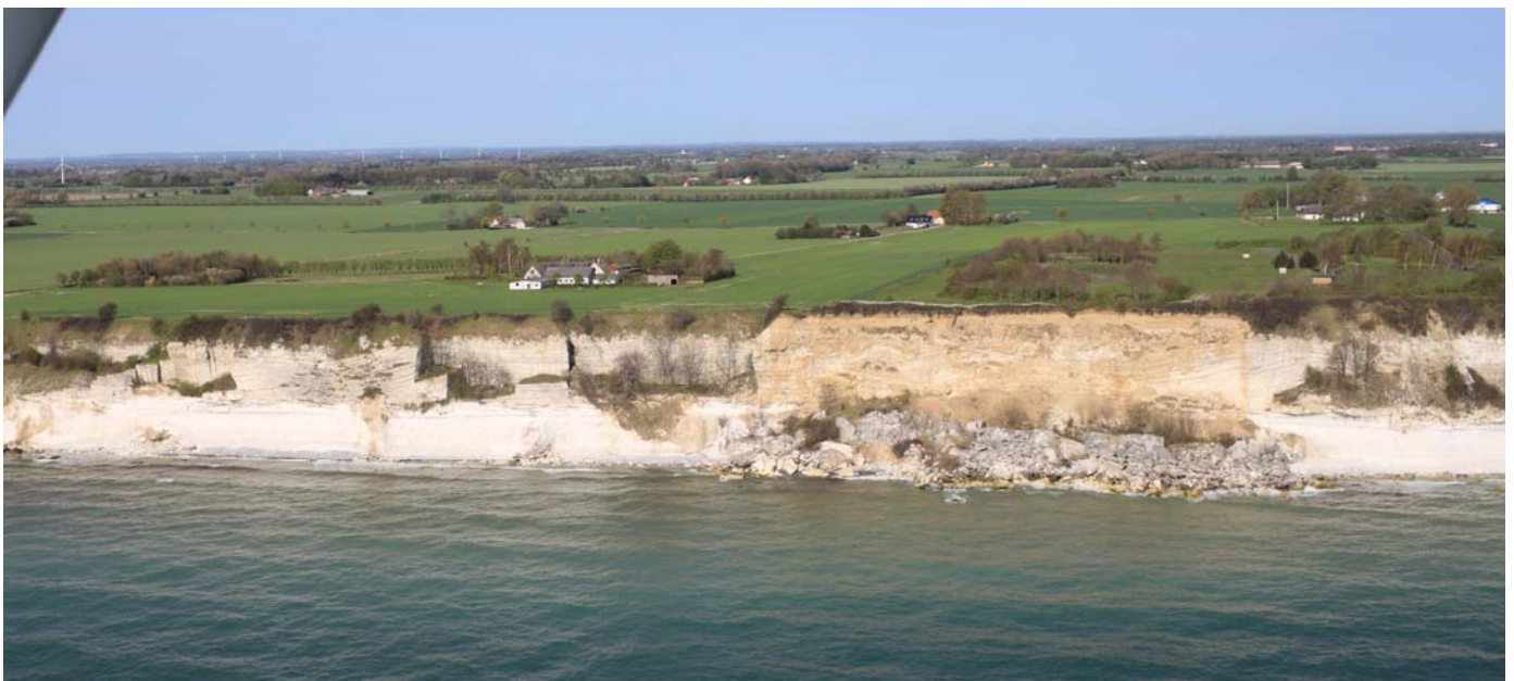
Figure 15. The large rockfall c. 200 km south of Stevns Fyr. Note the 3–4 m thick till unit at the top of the cliff. The clay content in the till contributed to a mixed rockfall development.
