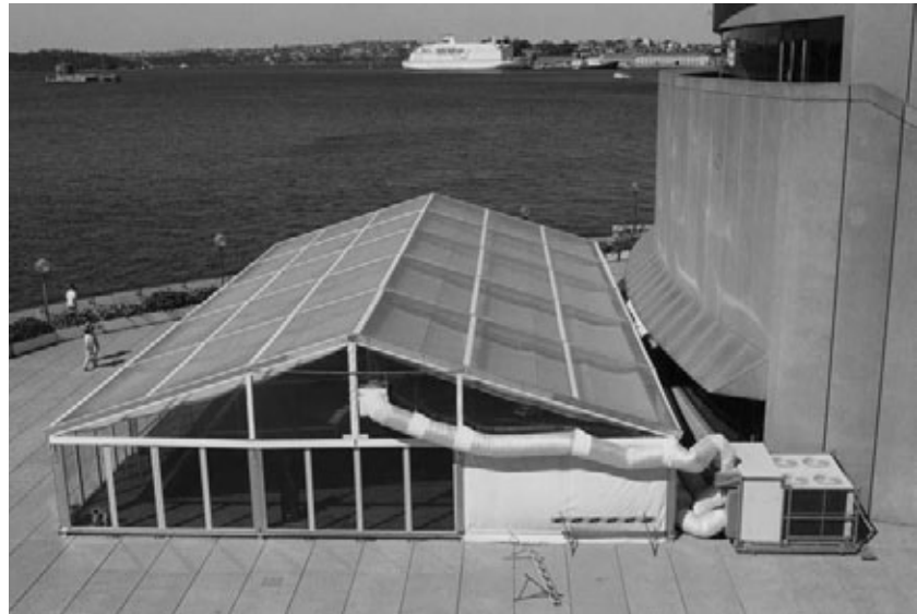
32. Unacceptable 'temporary' (i.e. long stay) venue for hire located against the north wall of the podium. The air conditioning plant is on the right and the servicing trucks are out of the picture on the left. The structure remained in place from September 2002 to April 2003. JSK photograph 19.9.2002.
