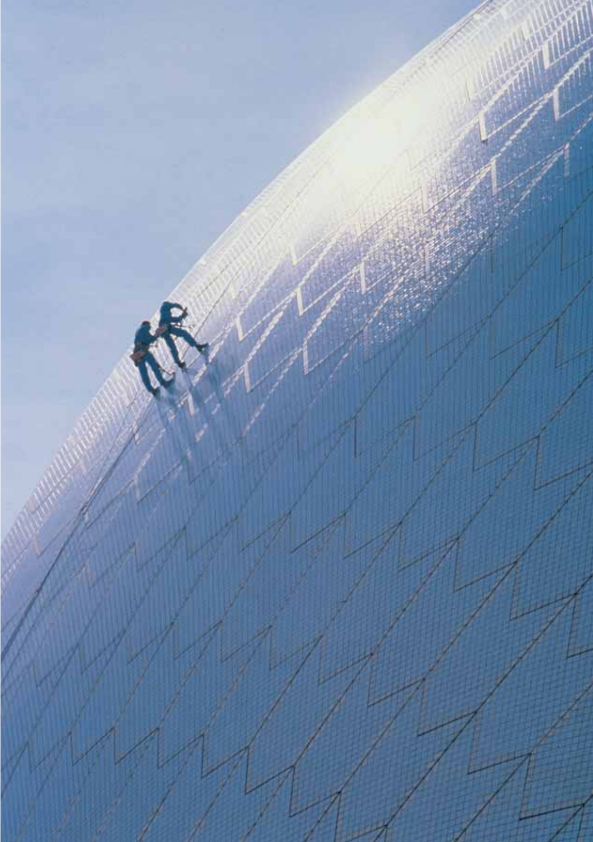
Figure 6.2 Monitoring the sealants to the tiling
