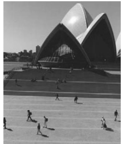
30a Clear forecourt. JSK photograph 2002.5.14A.
