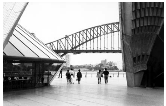
36. The podium deck and bronze railing showing the canted glass walls at eye level which ensure that reflections do not mar the view from the interior, 1993. JSK photograph 93.8.10.
