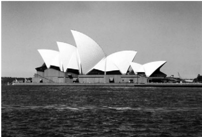
39. West elevation showing: on the left, the original podium cladding and broadwalk skirting; and, on the right, the 1988 sea wall of the lower forecourt. JSK photograph 93.7.0.
