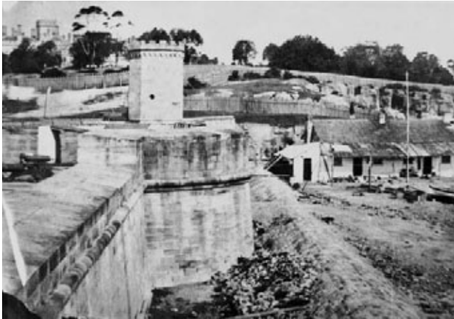
70. Detail of Matthew Fortescue Moresby's late 1850s photograph showing the main sewer on the western side of Fort Macquarie. Provided by the Department of Public Works in 1993.
