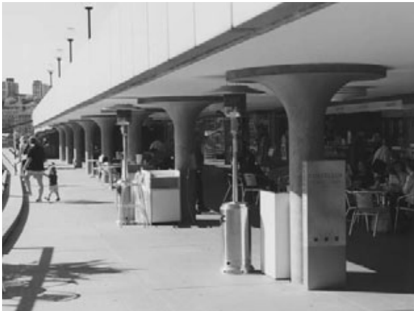
44. Lower forecourt showing column bases obscured by furniture. JSK photograph September 2002.
