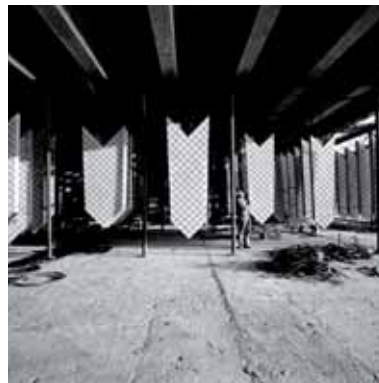
Figure 3.30 The precast tile lids awaiting placement
