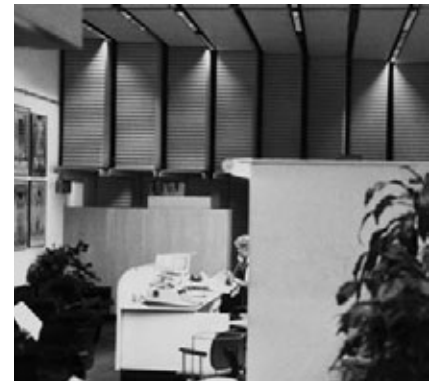
54a. Former administration foyer showing progressive degradation by partial removal of strip lighting and intrusion of makeshift partitions, 1993. JSK photograph 93.8.23.
