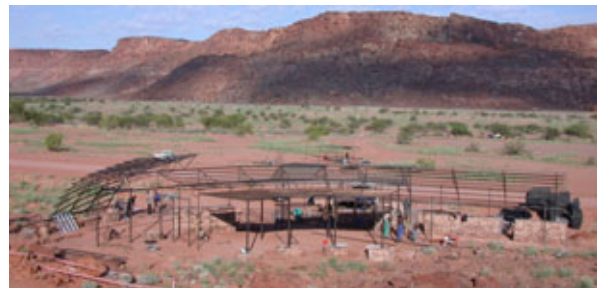
Fig. 11: Progress on 15 April 2005
