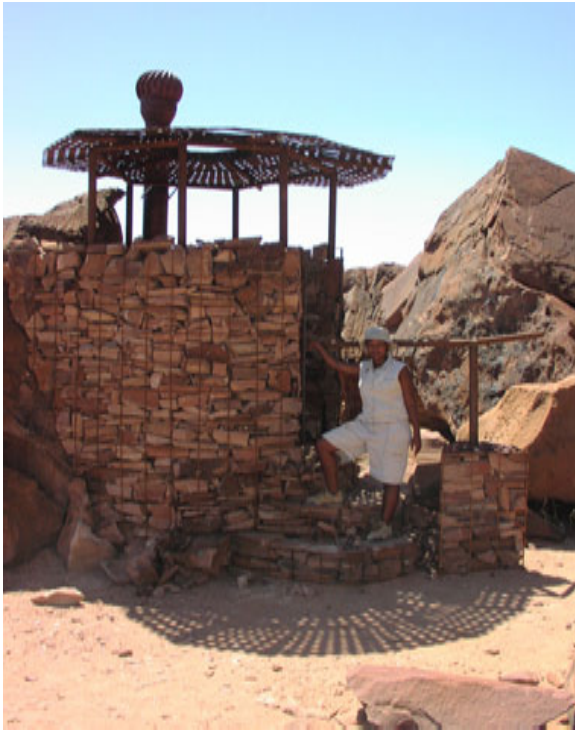
Dry compost toilet erected during site restoration work in 2005
