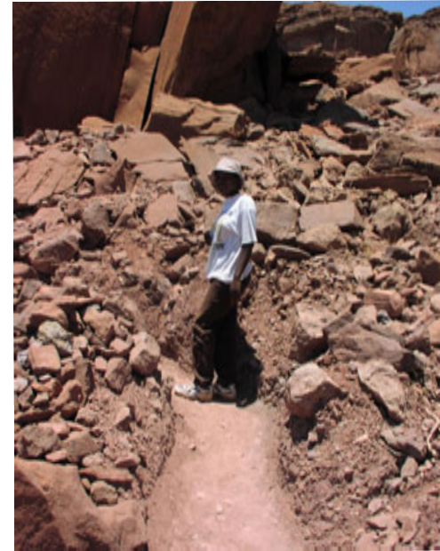
Severely eroded pathway showing depth of gulleying prior to restoration work in 2005
