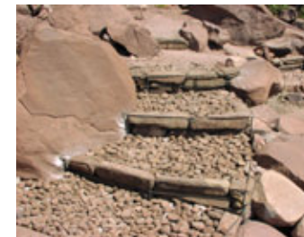
Steel gabion and gravel steps
