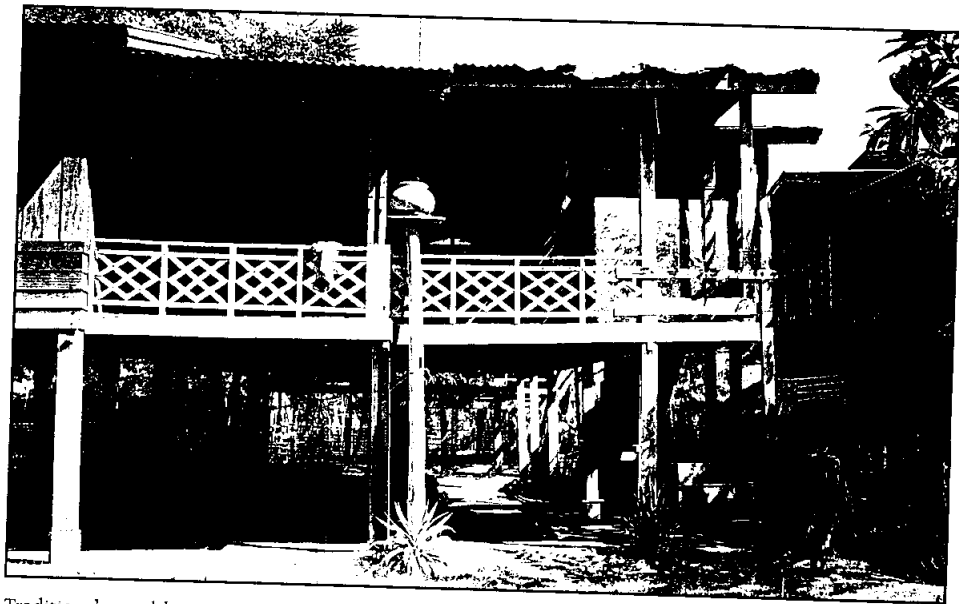
Traditional wood housing construction has had minimal impact on the subterranean archaeological resources and contributes to the character of the cultural landscape
