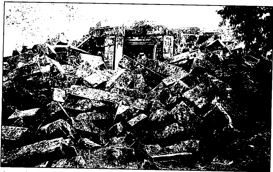
The temple at Hong Nang Sida illustrates the extent of the conservation work needed in the Champasak Heritage and Cultural Landscape Protection Zone
