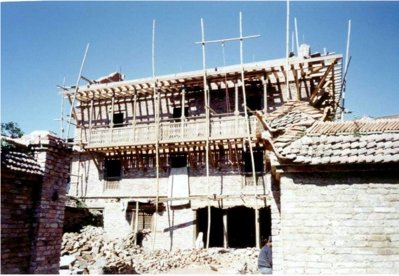
Restoration of a typical Kathmandu house using traditional materials and methods
