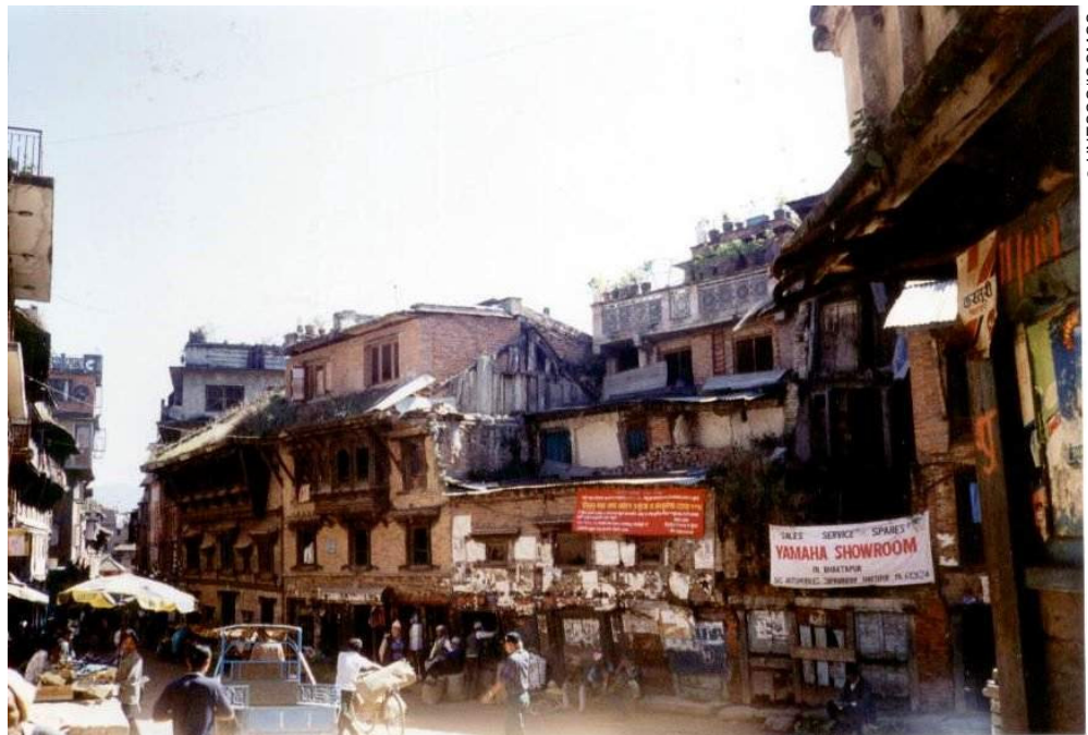
Chaotic and unregulated urban development marring the visual impact of the Kathmandu Valley
