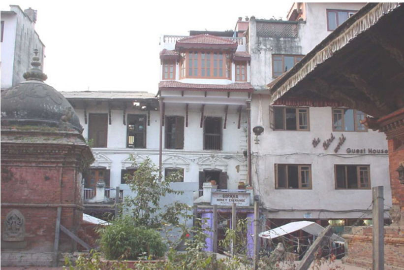
Illegal elevation on a traditional building within Patan Monument Zone
