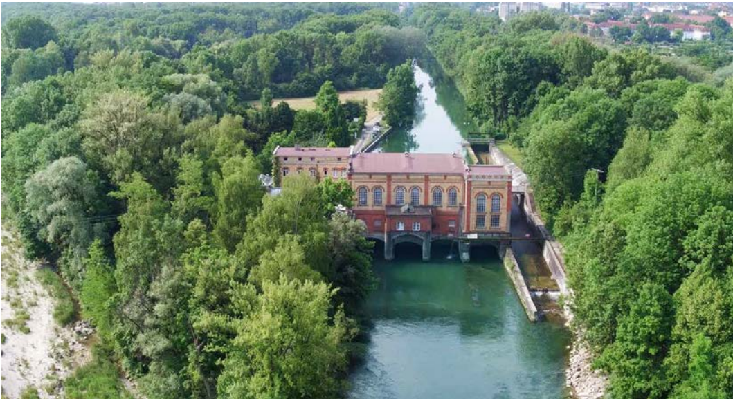
Wolfzahan power plant
