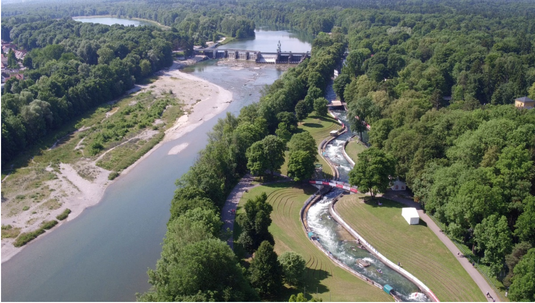
Aerial view of Hochablass Waterworks
