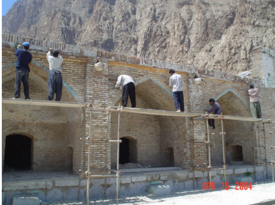
Picture 51. Shâh-Abbâsi Caravanserai under restoration
