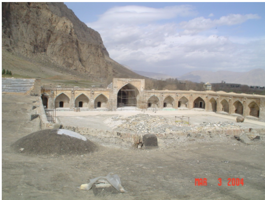
Picture 52. Shâh-Abbâsi Caravanserai under restoration
