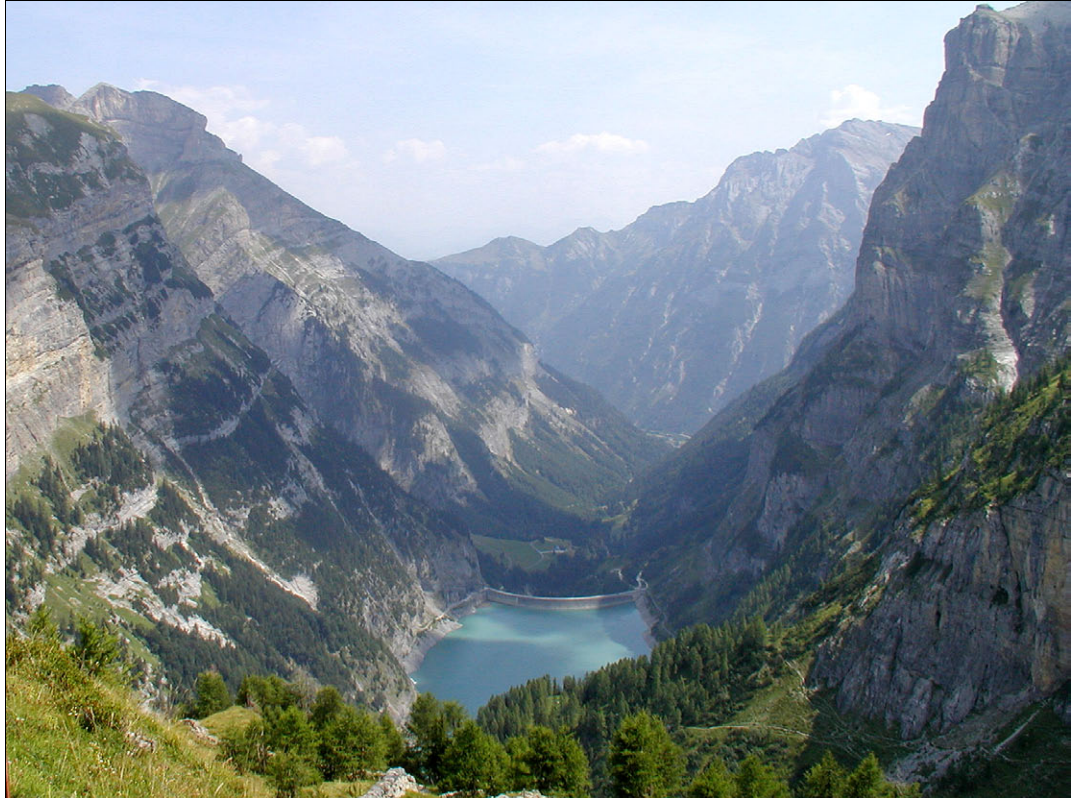
Fig. 02-33: The Gigerwald reservoir is used to produce renewable energy. Photograph: D. Imper, Heiligkreuz.
