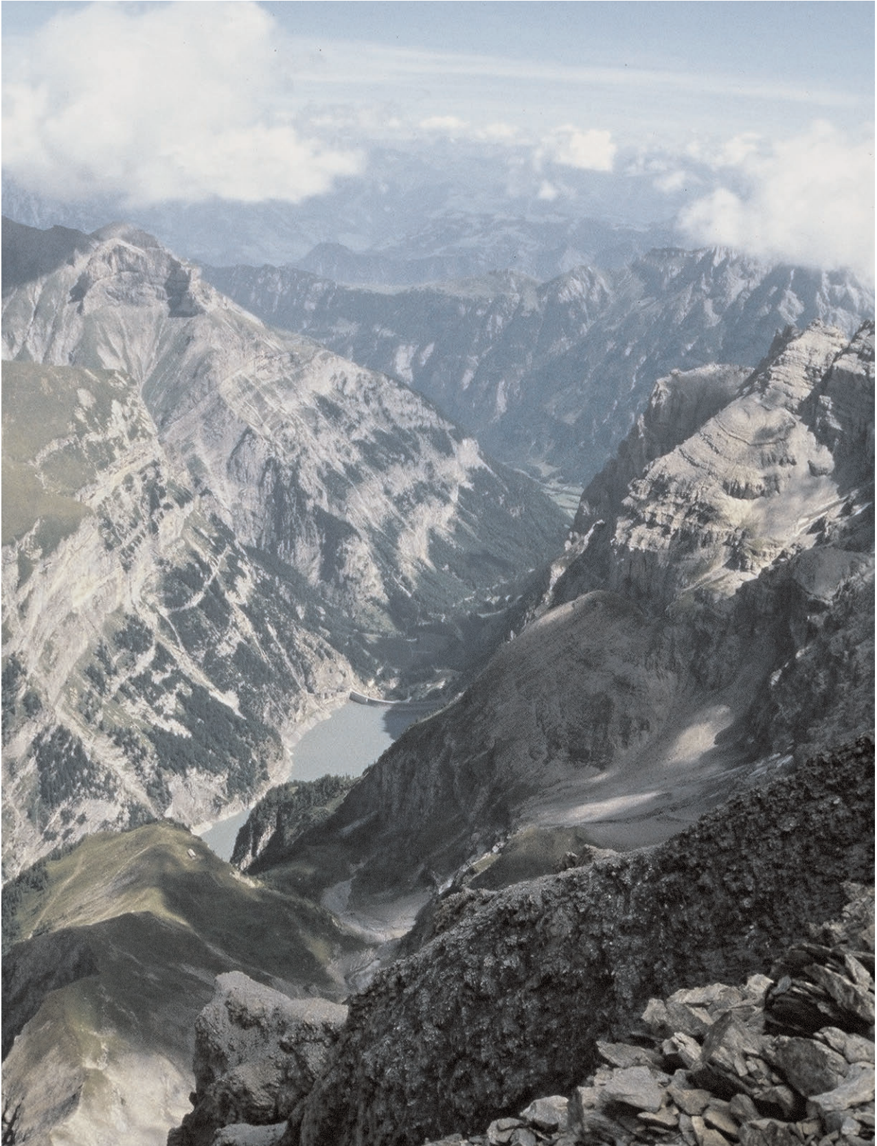
Fig. 02-11: The Gigerwald reservoir produce renewable energy. Photograph: D. Imper, Heiligkreuz.
