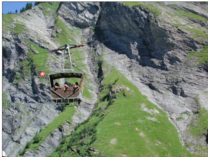
Fig. 04-01: The Niedererbahn is the only mountain railway within the boundary of the proposed World Heritage site. Photograph: H. Brühwiler, Elm.
