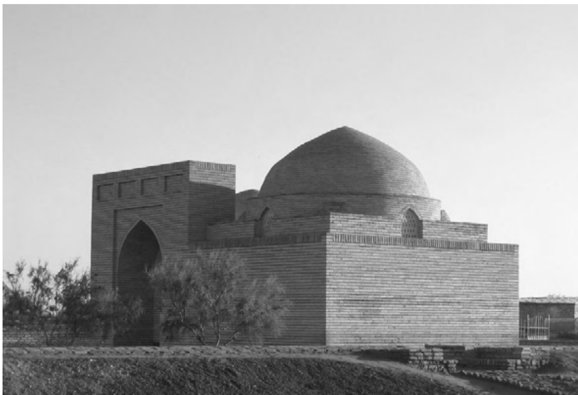
rebuilt on the ancient foundation, after it collapsed in 1993
