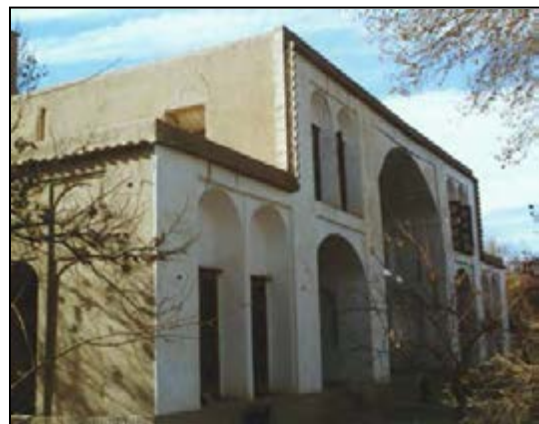
Fig .6-299.c. (Base of nominated gardens of Yazd)
