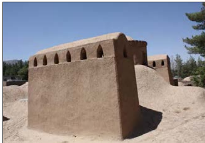
Fig .3-188. Usage of mud brick and Kahgel in the building
