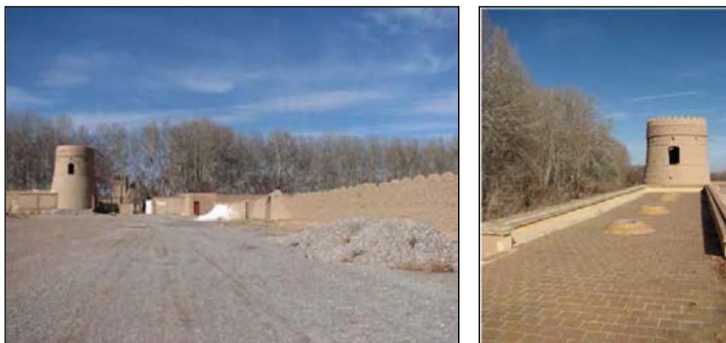
Fig.4-45. The tower after done repairs (The Base of Persian Garden, Yazd)
