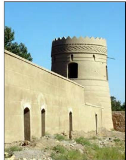
Fig .2-253. Surrounding Wall Tower.
