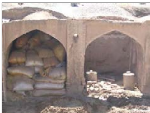
Fig.4-56.Stall before restoration (Base Of Bagh-e Akbariyeh )
