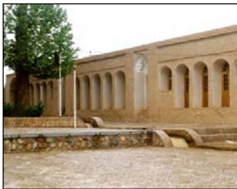
Fig. 2-217. The rooms around yard
