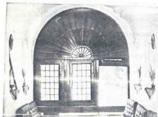
Fig.4-34.Restoring doors and plasters inside the Shahneshin 1987- 1995 (Base of Bagh-e Shahzadeh )
