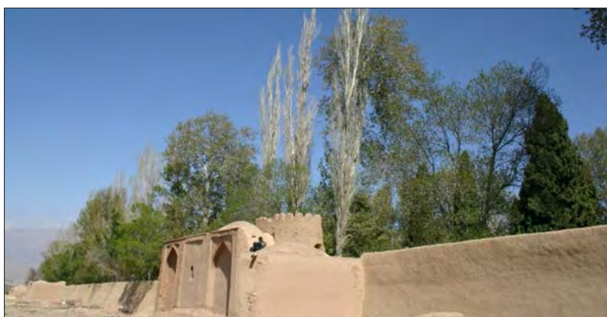
Fig .3-150. Western wall & tower of garden (Base of Bagh-e Shazadeh -2009)
