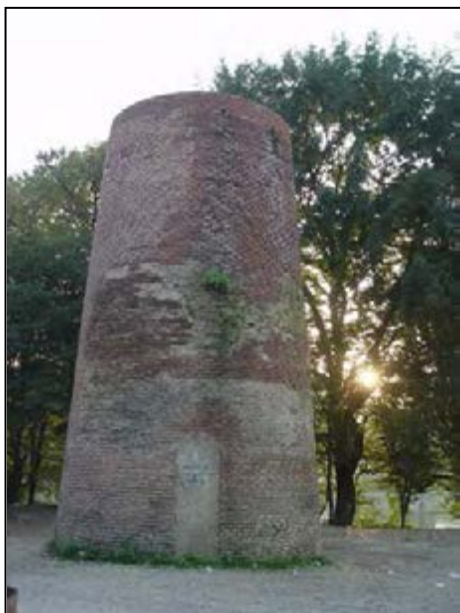
Fig.4-90.Environmental affects on the tower of the garden (the Base of Bagh-e Abas Abad )
