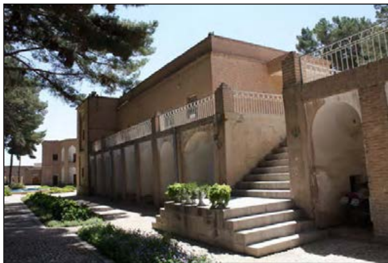
Fig . 2-299.Connecting stairways in subsidiary structure
