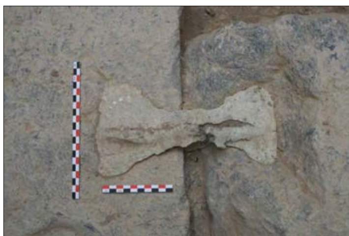
Fig. 6. Detail of a dovetail-clamp in situ
