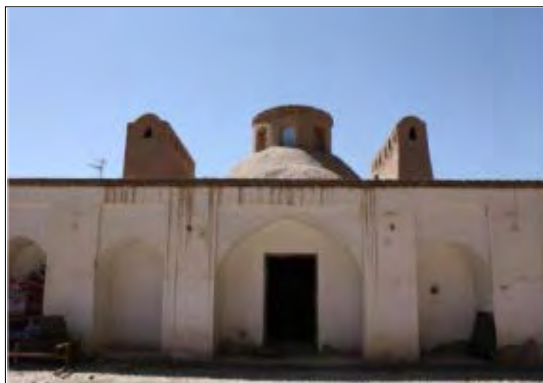
Fig. 3-202. Badgirs of the service section in the back Miansara
