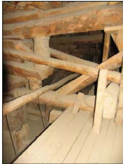
Fig .-105. The wooden roof truss and ceiling apparatus maintained in their authentic condition (Fazeli-Nezhad, 2009)
