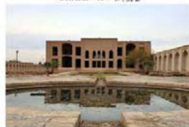
General View (6).jpg
