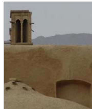
Fig. 3-132. Usage of traditional materials (Kahgel) for covering the roof (Khoshnood)
