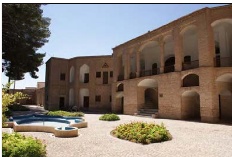
Fig . 2-289 . View of the main pavilion
