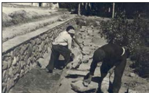
Fig.4-31.Installing the water course stones (Base of Bagh-e Shahzadeh )
