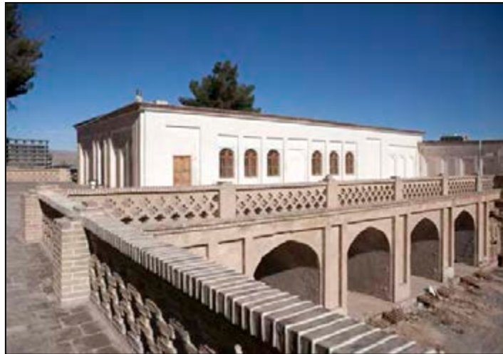
Fig . 2-295. Internal view of Stable
