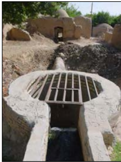
Fig .2-249. Mirza Nasrollah water mill
