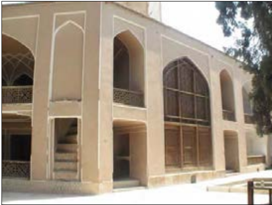
Fig. 3-170. East facade of Wind tower building
