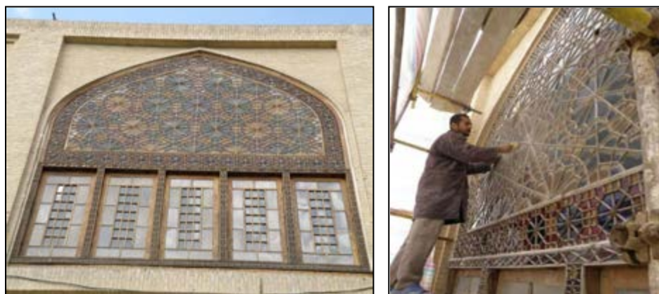
Fig.4-20.Restoring the Orsi window (The Base of Persian Garden, Isfahan)
