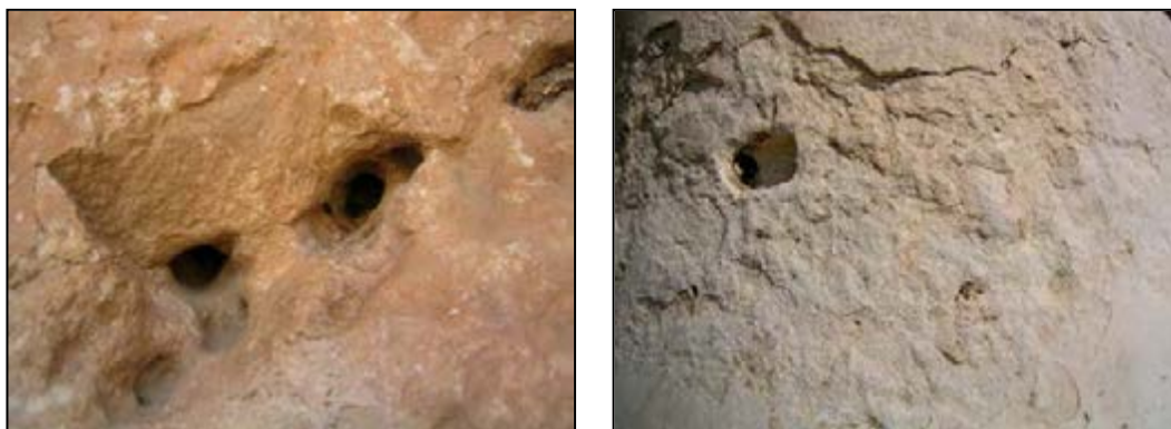
Fig.4-63. Sample of column slips erosion by wind and holes formed inside stones due to their aeration, Palace P( Parse-Pasargadae Research Foundation Archives)
