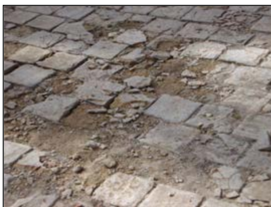
Fig.4-93. Brick pavements destroyed in the floor (Gholamnejad)
