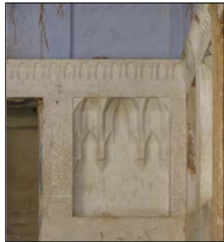
Fig.3-137. Karimkhani private chamber portico (Khoshnood) chamber rooms (2007)
