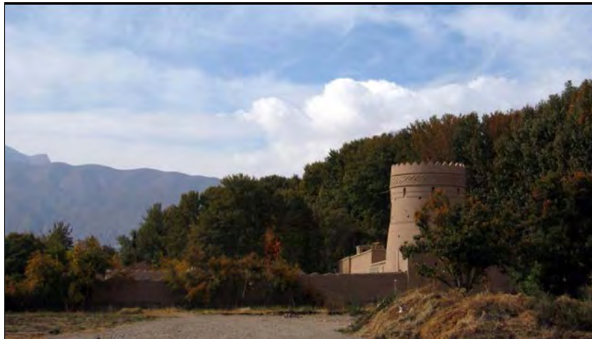
Fig .3-187. Photo showing the wall and entrance tower of the garden
