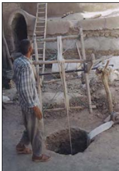
Fig.4-23. The shallow well that serves drainage system. (The Base of Persian Garden, Isfahan)
