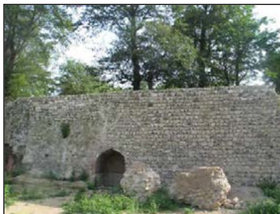
Fig.4-28.Stone wall after restoration (Base of Bagh-e Abbas Abad )
