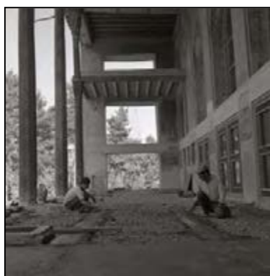
Fig.6-95.1958, During the restorations (ICHHTO of Isfahan)
