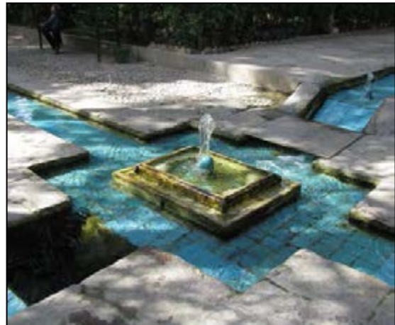
Fig .2-153. The water division point in front of Safavid Shotor Galu (Khoshnood, 2009)
