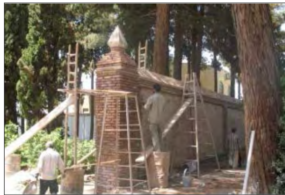
Fig. 3-201. Pier-laying of the inner space using uniform materials
