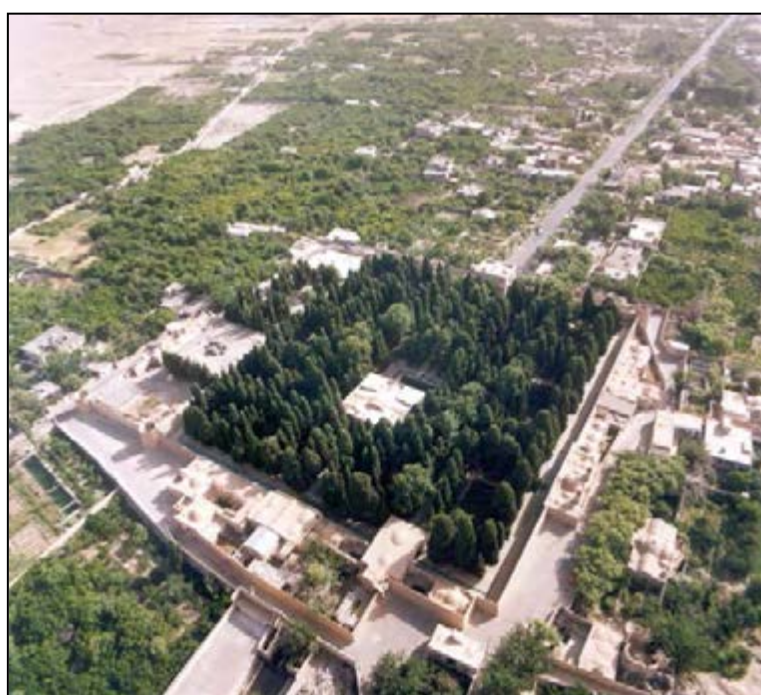
Fig. 2-127. General view of Bagh-e Shahzadeh Mahan
