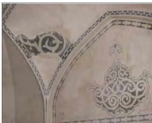
Fig . 3-112. Stucco decorations inside the bath house of the garden
