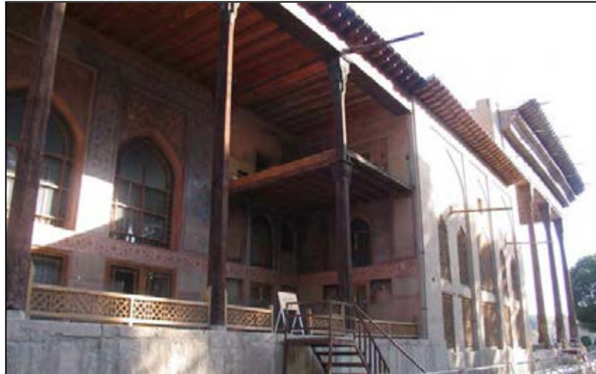
Fig . 2-111. The south façade (Fazelinejad, 2009)
