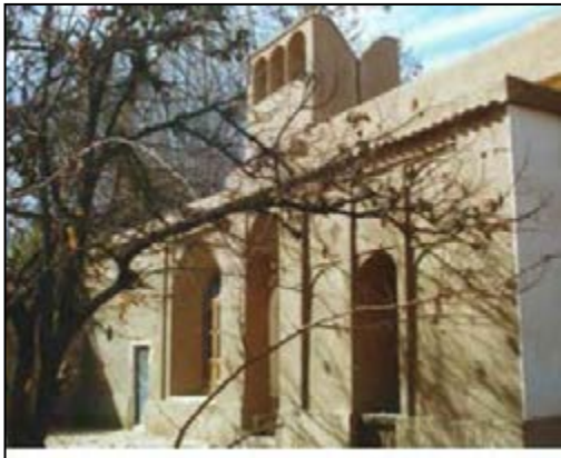
Fig.4-46.The pavilion after performing Kahgel coat (The Base of Persian Garden, Yazd)
