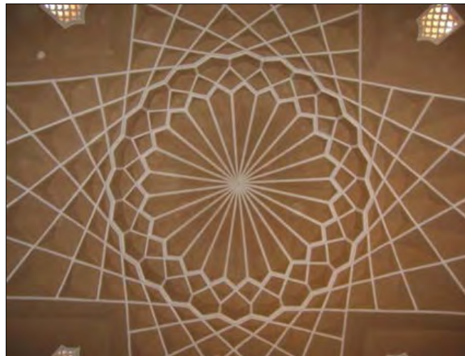
Fig .3-189. Photo showing Karbandi of the main pavilion
