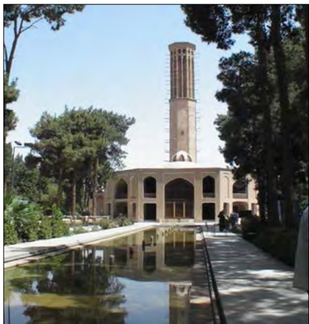
Fig. 3-159. Badgir building (summer palace), 2008
