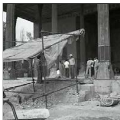
Fig.6-96.1958, During the restorations (ICHHTO of Isfahan)
