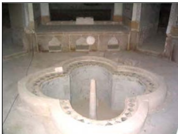
Fig.4-10. Restoring hamam's pond (The Base of Persian Garden, Fars)
