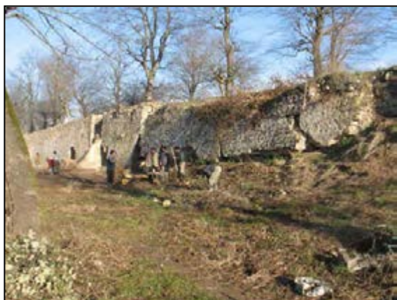
Fig.4-27.Stone wall before restoration (Base of Bagh-e Abbas Abad )
