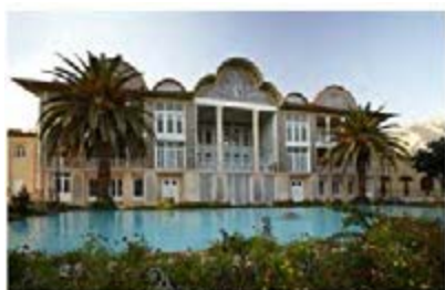
General View (7).idm
