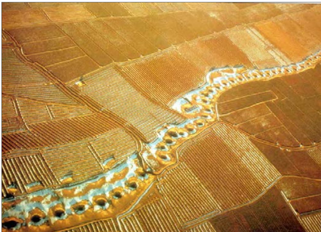
Fig .40. Aerial view of a Qanat passing under the grounds located near Yazd Source: Persian Garden a Reflection of Paradise, 2004
