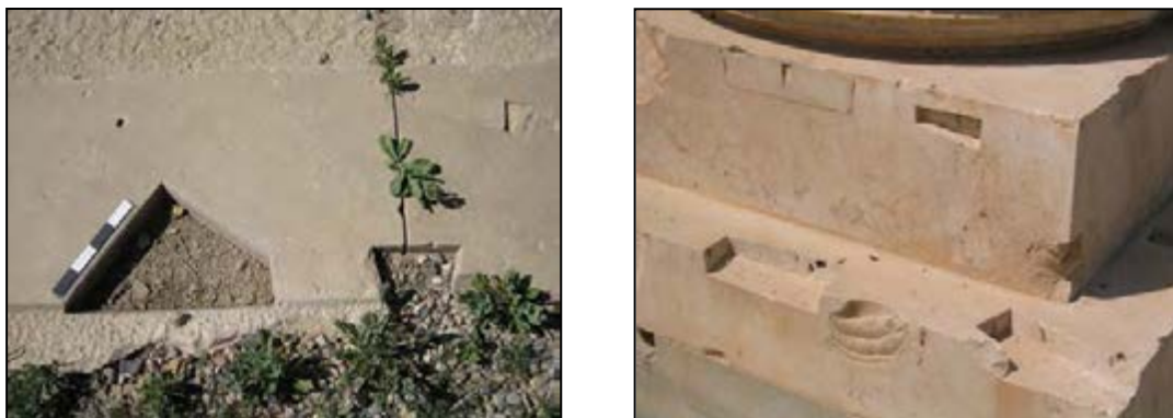
Fig.4-1.Repairs in the Achaemenids Era (Archives of Research Foundation of Parse-Pasargadae)
