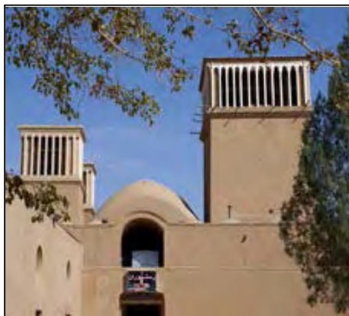
Fig . 2-233. Andarooni building, 2009
