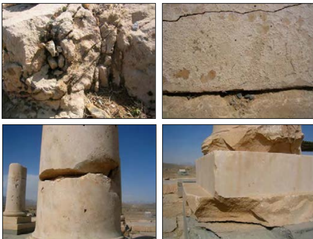
Fig.4-62. Stones breaking and crushing due to temperature oscillations and fall of building materials in Palace P (Parse-Pasargadae Research Foundation Archives)
