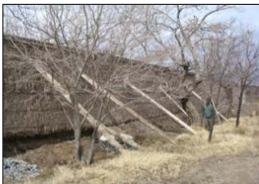
Fig.4-54. Walls of the Bagh before Restoring (Base of Bagh-e Akbariyeh )
