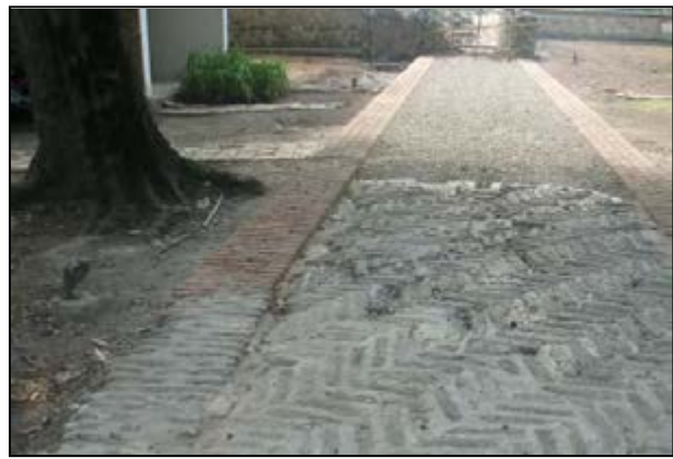
Fig.4-30.Restoration of pavements (Base of Bagh-e Abas Abad )
