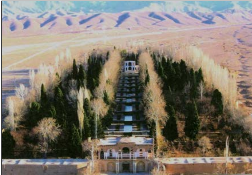
Fig .2-196 . General view
