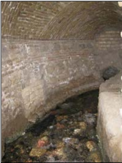
Fig. 2-150. The aqueduct that conduct the water of the Fin Spring (Khoshnood, 2009)
