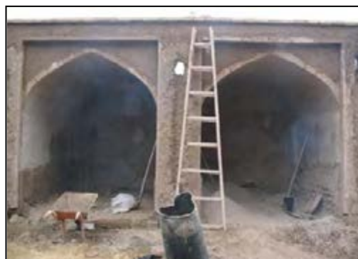
Fig.4-57.Stall after restoration (Base Of Bagh-e Akbariyeh )
