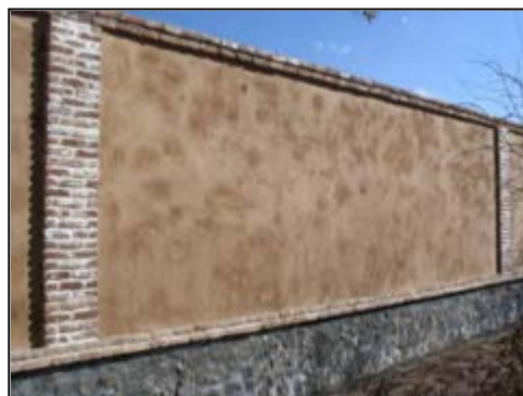
Fig.4-55. Restoring and repairing the walls (Base of Bagh-e Akbariyeh )
