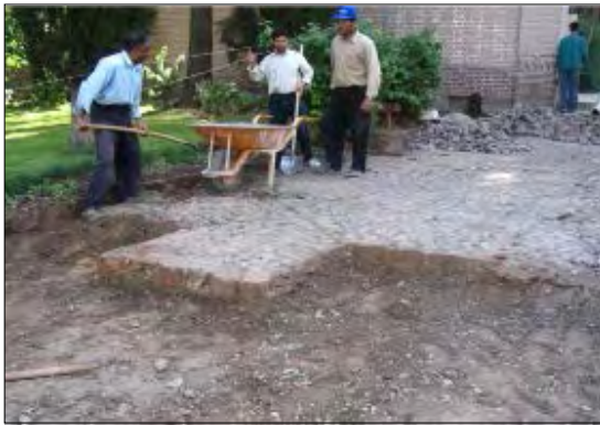
Fig. 3-200. Restoration of floor paving with uniform materials
