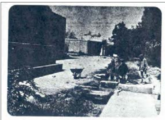
Fig.4-36.Restoring partitions of water course (Base of Bagh-e Shahzadeh )
