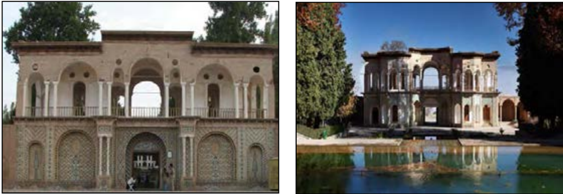
Fig .2-209. Sardar khaneh (Entrance house) exterior view of Bagh- e Shahzadeh, 2003
