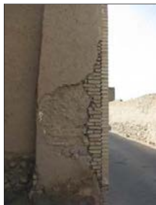
Fig. 3-131. The restoration of the Khalvat-e-Karimkhani entrance wall)(Khoshnood)
