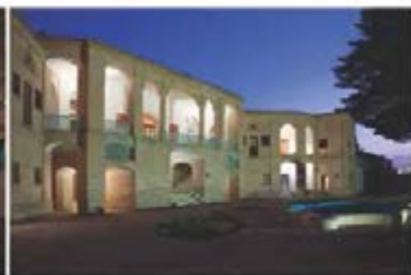
General View (6).jpg
