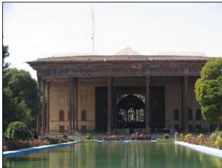
Fig .2-94. The pool in front of the palace (Fazelinejad, 2009)
