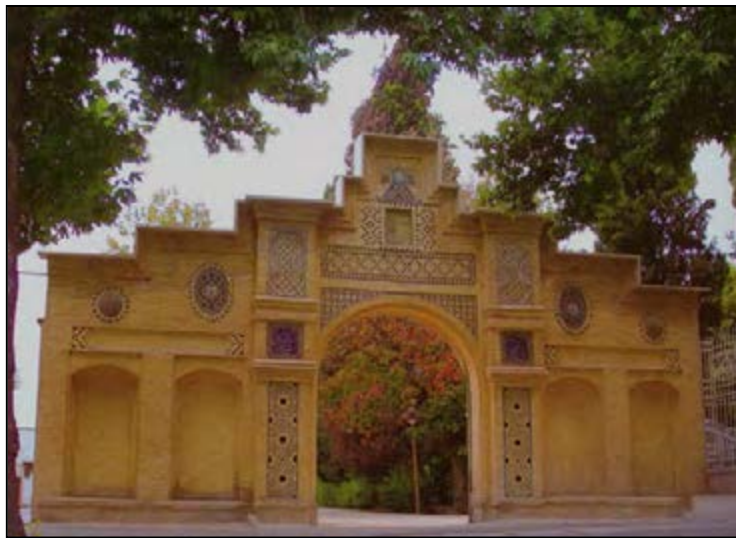
Fig. 2-77. North eastern entrance (M.R.Sharif, Bagh-e Eram )
