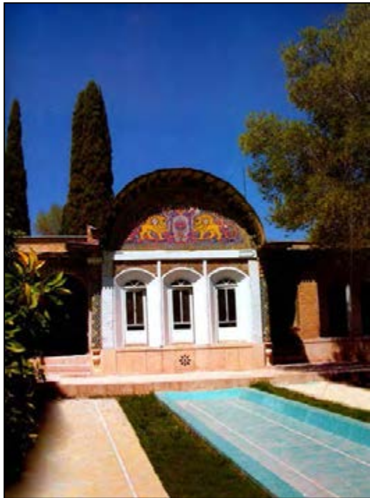
Fig. 2-75. At the front part of the andaroon (the seraglio), there is a quadrilateral structure, known as the Gholam-Neshin (lit. slave room).
