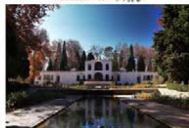
General View (6).jpg
