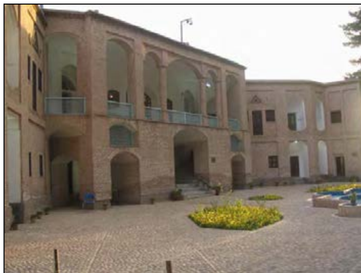
Fig. 2-365. View of main building (rear court)
