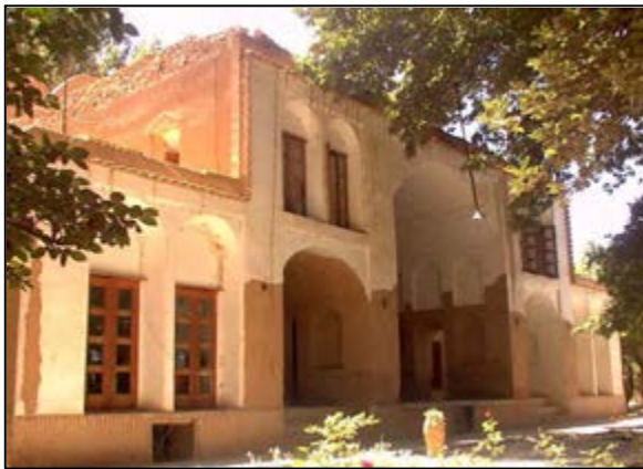
Fig .6-298.c. (Base of nominated gardens of Yazd)
