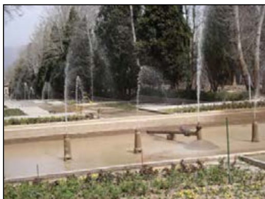
Fig.4-42. Restoring the fountains (Base of Bagh-e Shahzadeh )
