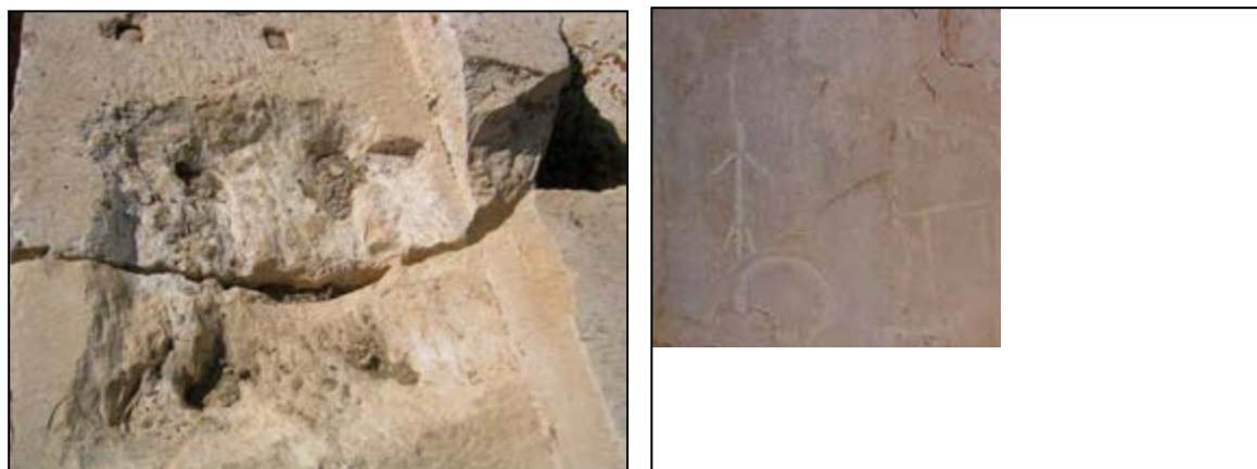
Fig.4-66.Removal of dove-tailed clamps and patches as well as engraving impressions on monuments (Parse-Pasargadae Research Foundation Archives)
