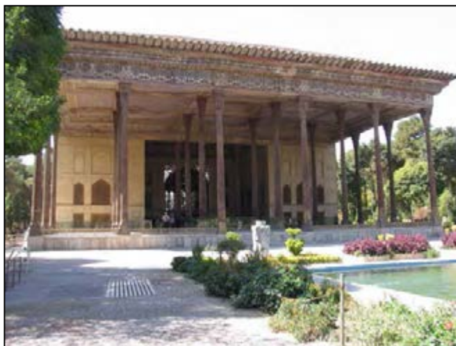
Fig .2-102. The east facade of Chehel Sotun Palace (Fazelinejad, 2009)
