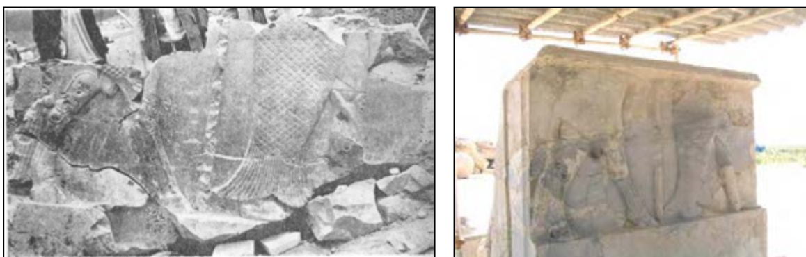
Fig.4-2.Pattern of the left side pier of the doorway threshold standing southeast of the Audience Hall Palace before and after restorations of Ali Sami. (Archives of Research Foundation of Parse-Pasargadae)
