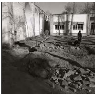
Fig .6-94.1975, During the restorations (ICHHTO of Isfahan)
