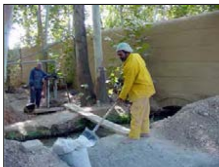
Fig.4-52. Restoring water ways and Karts (The Base of Persian Garden, Yazd)
