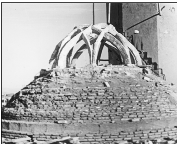
Fig.3-172. Restoration of wind tower building's ceiling,1970
