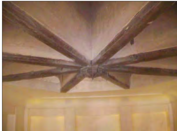
Fig. 3-174. View of under the wind tower
