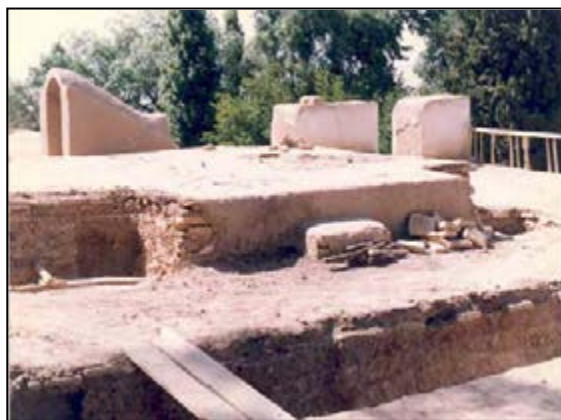
Fig.4-38. Restoring the second floor of Shahneshin (Base of Bagh-e Shahzadeh )
