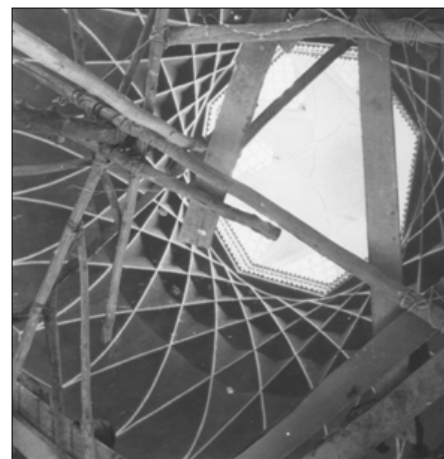
Fig.3-173. Restoration of Karbandi of Wind tower building,1970
