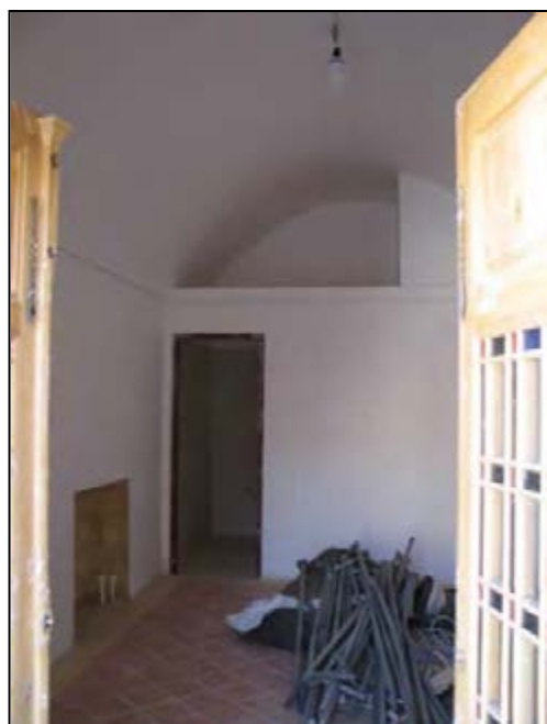
Fig.4-100.Using some spaces as stock room (Base of the Persian Garden, Yazd)
