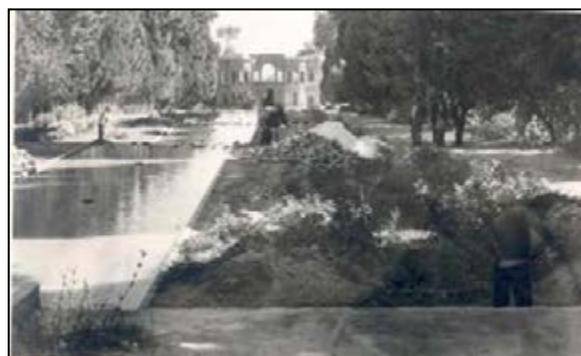
Fig.4-32.Soil removing around the pond (Base of Bagh-e Shahzadeh )
