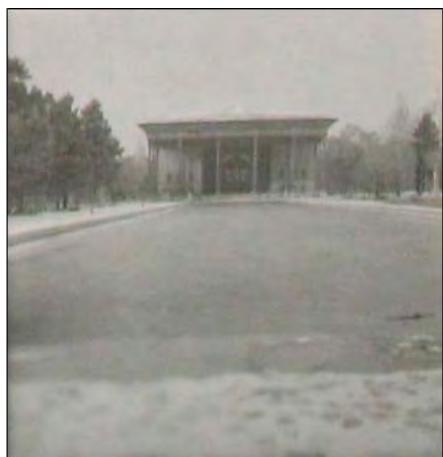
Fig .3-95. Bagh-e Chehel Sotun pavilion in 1959 (NHBI Base)
