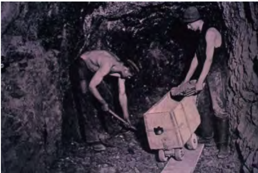
002 070 FILLING THE MINE CART (TRUGCA) WITH THE ORE
