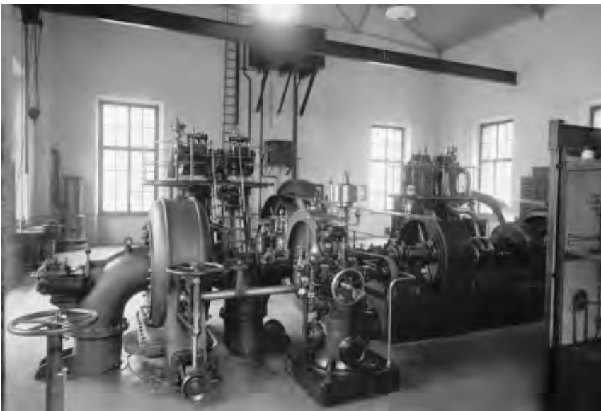
002 143 THE MINE'S POWER PLANT WITH ITS DIESEL ENGINE AND WATER TURBINE IN 1915
