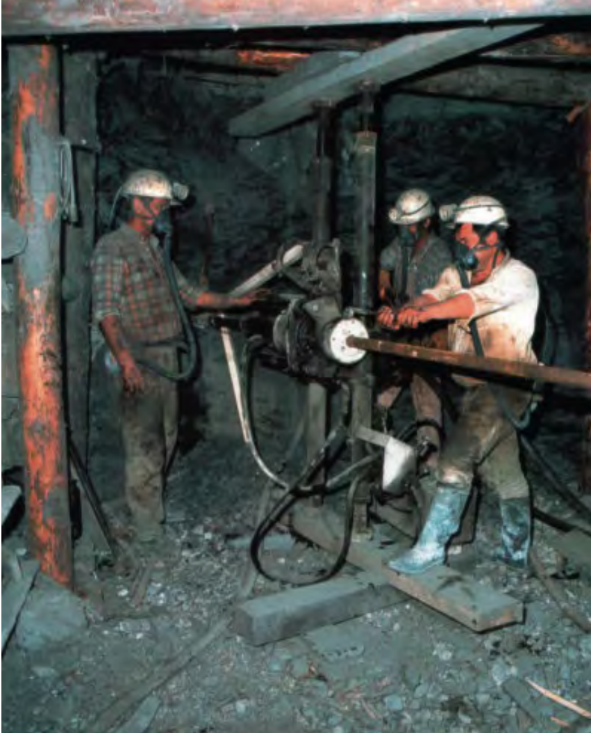
002 115 CLOSURE WORKS – DRILLING OF INJECTING BORES.
