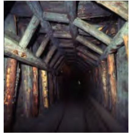
002 014 THE MAJORITY OF THE TUNNELS IN THE MINE ARE SUPPORTED BY WOODEN BEAMS.
