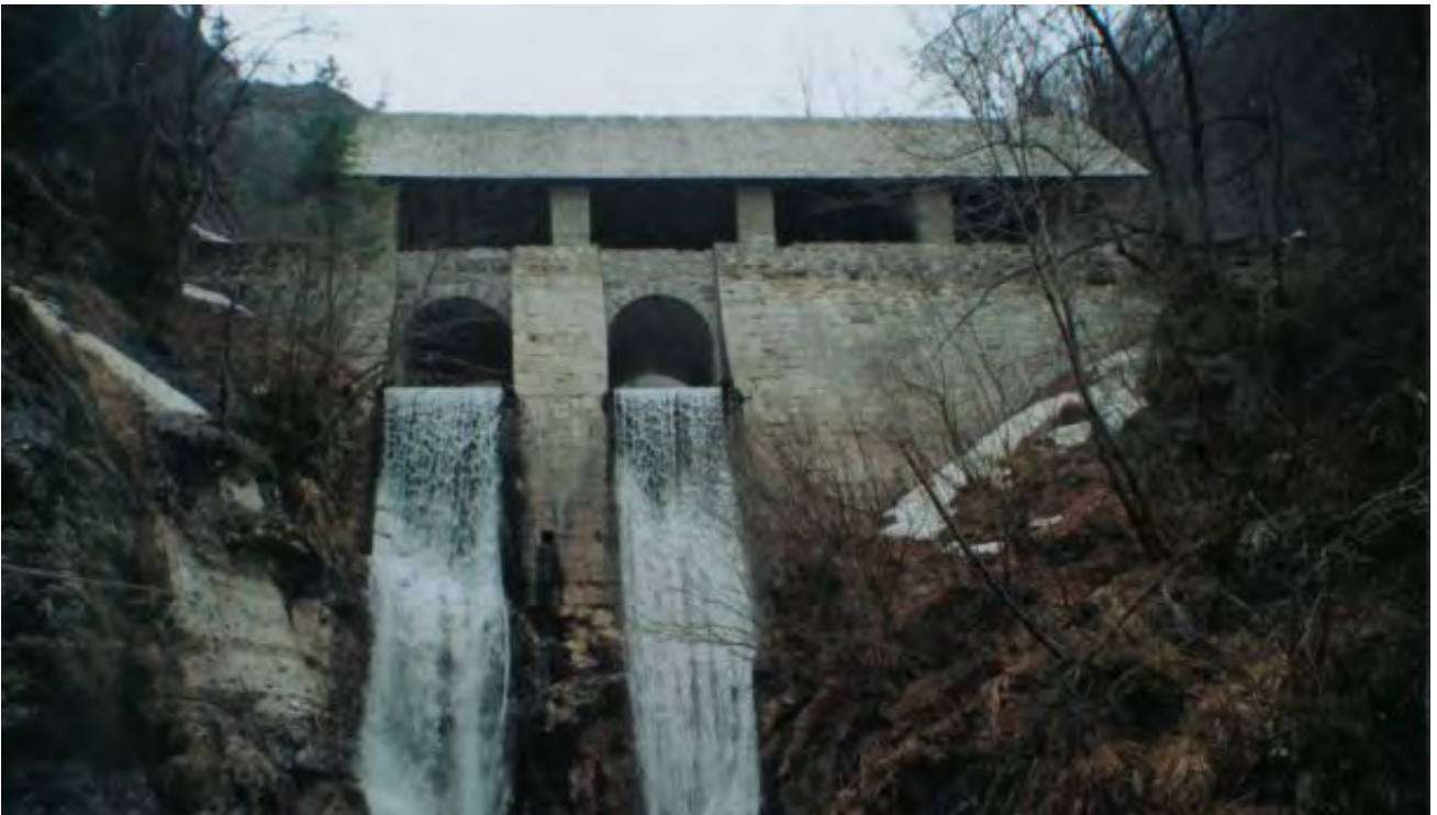
002 027 THE PUTRIH'S KLAVŽE WATER BARRIER, 2004
