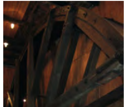
002 126 THE WOODEN WATER WHEEL OF THE IDRİJA KAMŠT WATER PUMP IS THE LARGEST OF THE KIND IN EUROPE.
