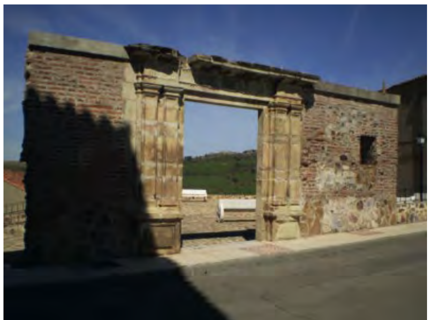
001 031 HOUSE OF THE MINE SUPERINTENDENT
