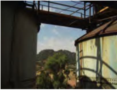
001 040 VIEW OF THE BUFFER ZONE FROM THE MINE
