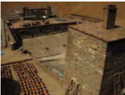
001 078 BUSTAMANTE FURNACES DURING REHABILITATION
