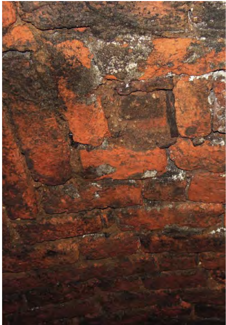
001 019 ENTRANCEWAY TO THE MINA DEL CASTILLO. BRICK BARREL VAULT
