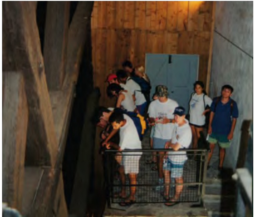
002 140 A VISIT TO THE DRIVE WHEEL OF THE KAMŠT WATER PUMP.
