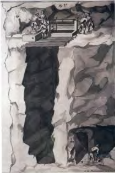
001 062 DRAIN WITH HAND WINCHES AND LEATHER CONTAINERS MADE BY ENFORCED LABOUR PRISONERS. (GENERAL ARCHIVE OF SIMANCAS)
