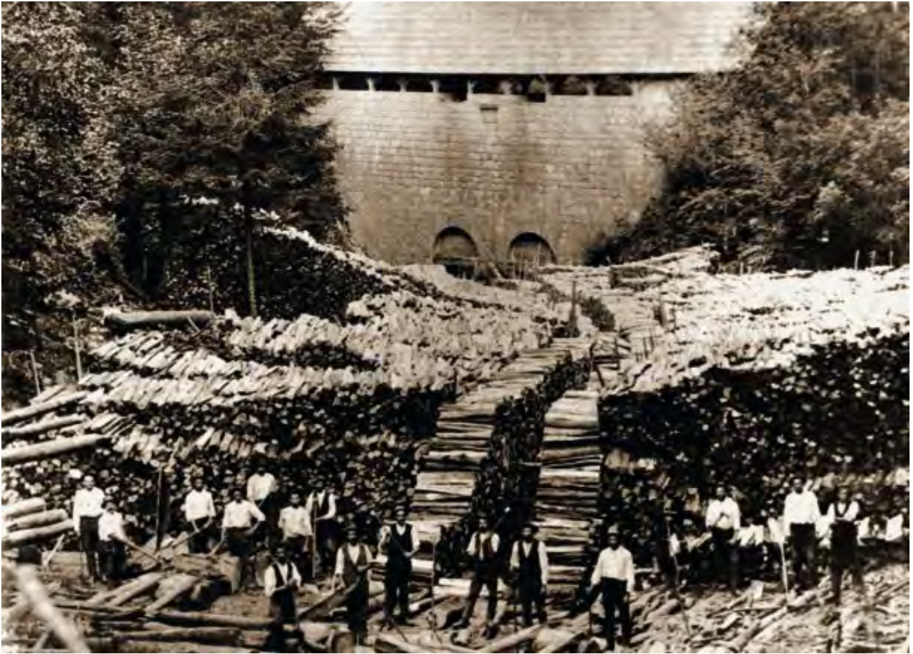
002 025 WOOD STACKS BEHIND THE KANOMLJA KLAVŽE WATER BARRIER, READY TO BE FLOATED – AROUND 1900
