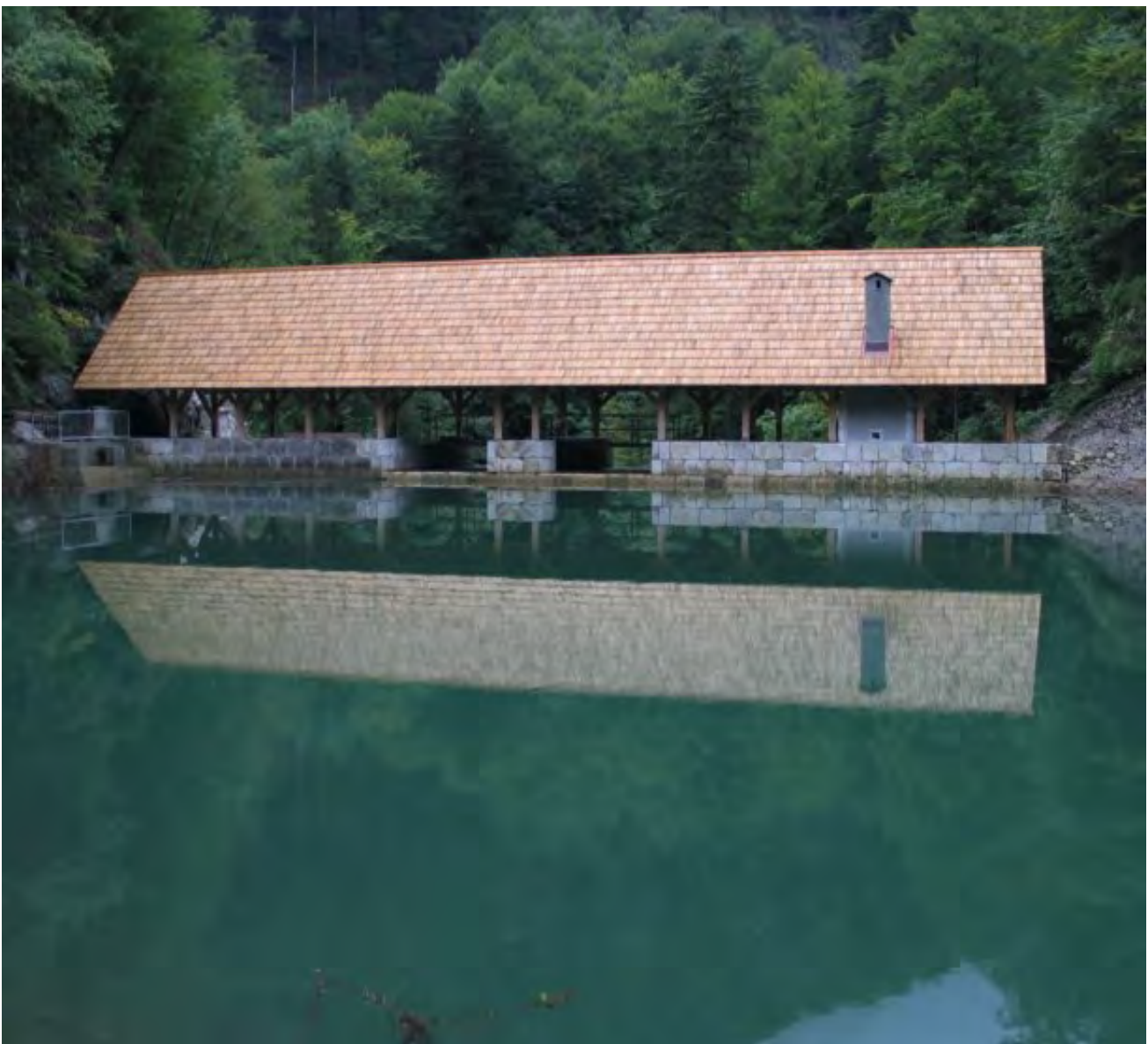
002 124 THE RESTORED KANOMLJA KLAVŽE WATER BARRIER ARE USED AS A DAM FOR A SMALL HYDROELECTRIC POWER PLANT, 2005.
