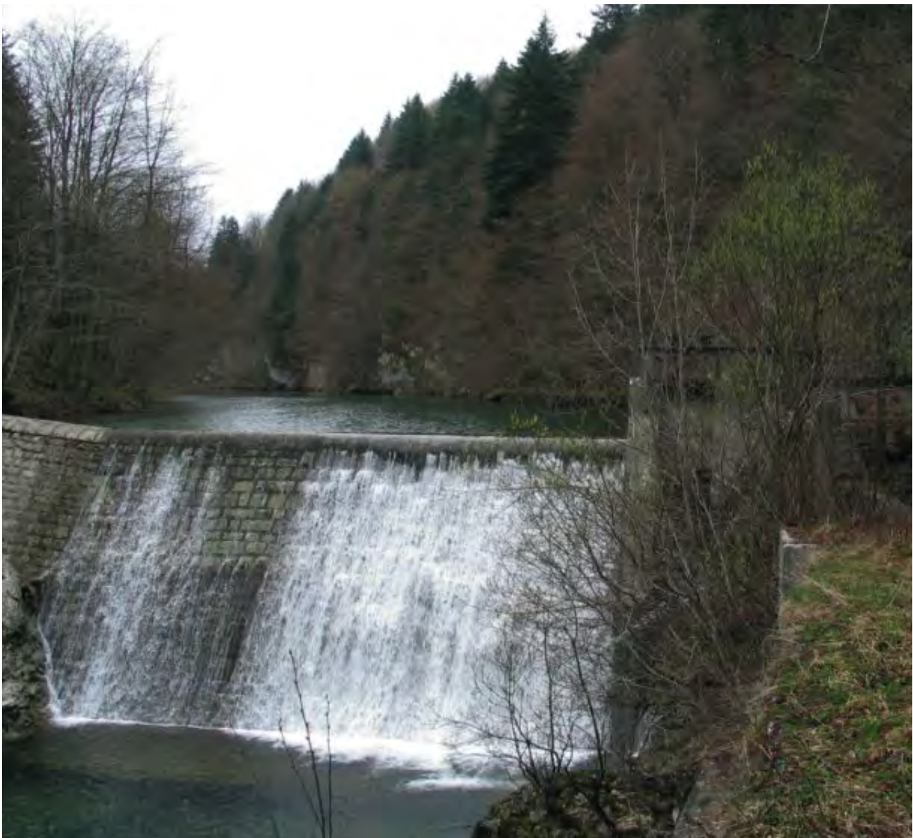
002 125 THE KOBILA DAM WITH THE RAKE WATER CHANNEL.
