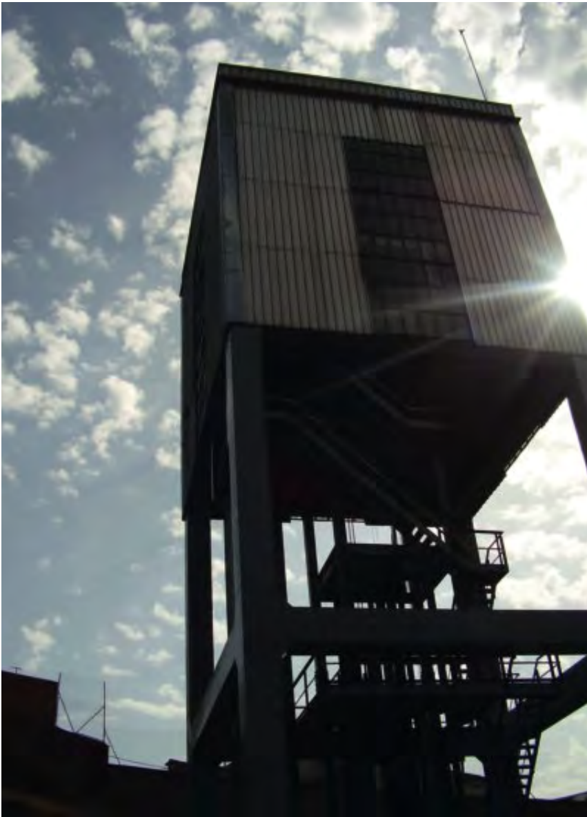
001 013 TOWER ABOVE THE SAN TEODORO SHAFT
