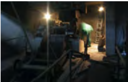
002 158 MACHINERY RESTORATION WORKS IN CRUSHING PLANT.
