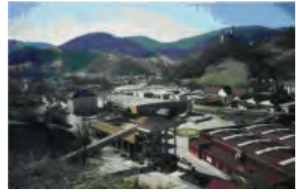
002 137 DEVELOPMENT OF MODERN INDUSTRY IN THE SMELTING PLANT AREA.
