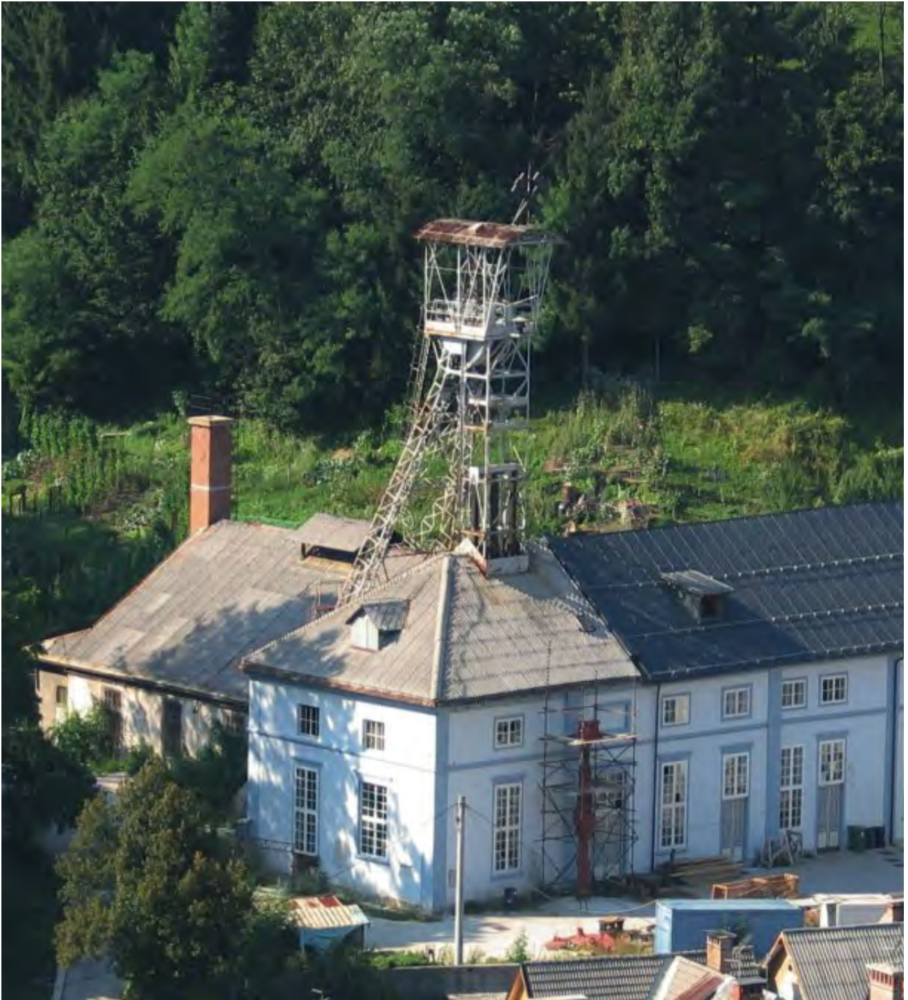
002 119 PARTIALLY RESTORED HEADFRAME OF FRANCIS'S SHAFT, 2005.
