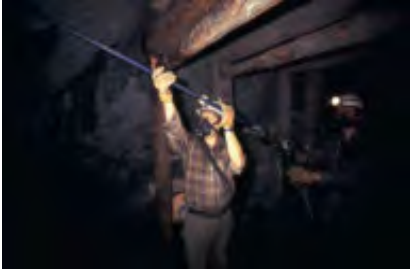
002 071 DRILLING MINE BOREHOLES WITH THE AID OF A PNEUMATIC DRILL
