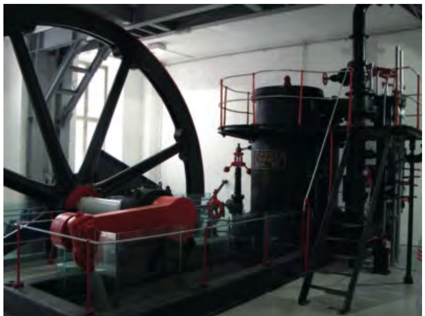
002 141 KLEY'S WATER PUMP IN THE HEADFRAME OF FRANCIS'S SHAFT WAS DRIVEN BY STEAM.
