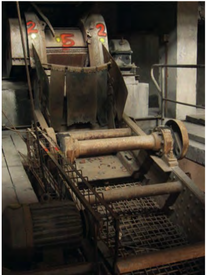
002 159 MACHINERY RESTORATION WORKS IN CRUSHING PLANT.
