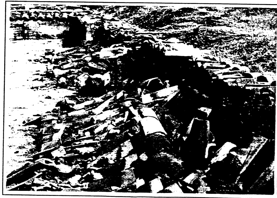
ANOTHER COLLAPSED WALL IN "LAS ESPAÑOLAS" RUIN.
