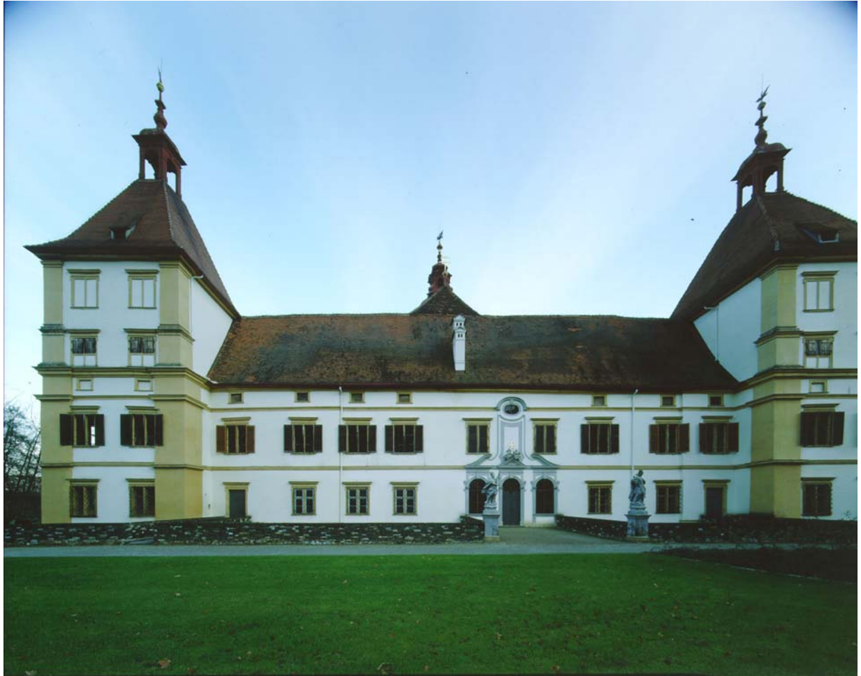
74. West front of the house. Church façade and entrance.
