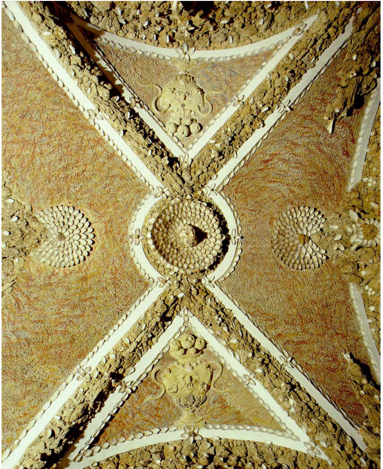
25. Shell ornamentation of the grotto vaulting
