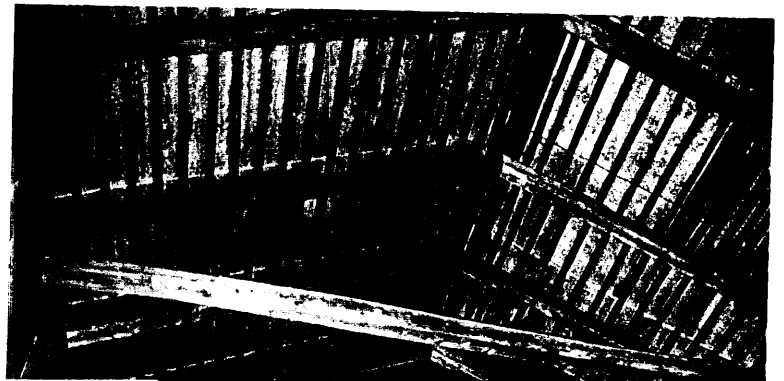
The attic of the structure
