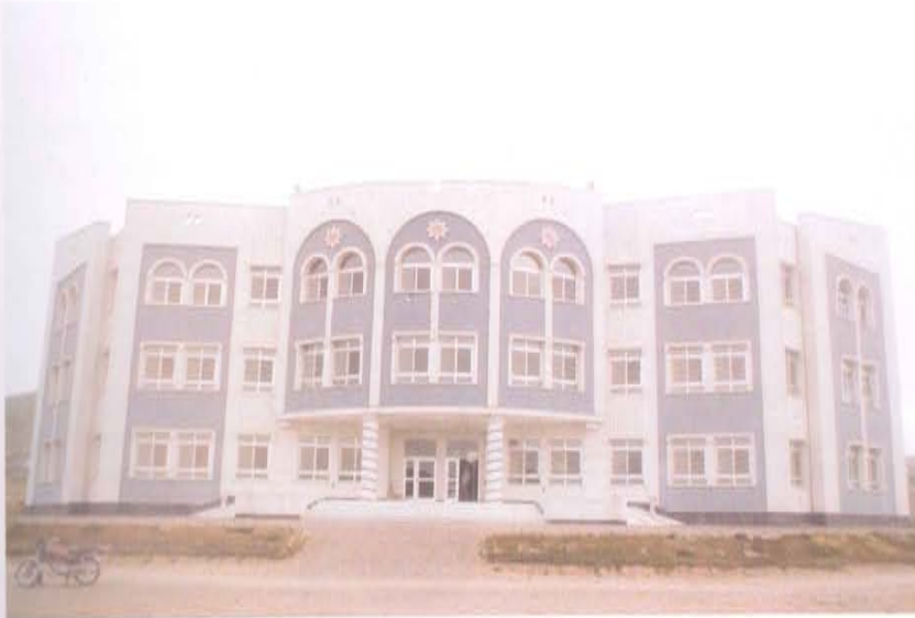
New Construction at Herat University
