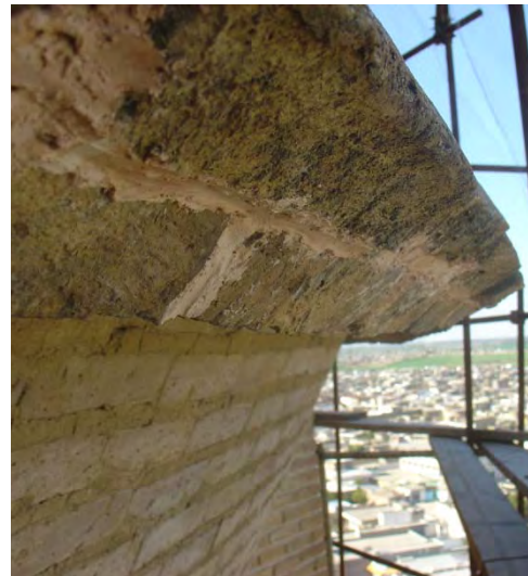
Figure 57 - The edge of the gutter of the conical roof
