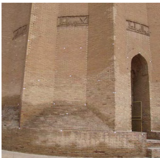
Figure 48 - South side of Gonbad-e Qābus (Lower Body)
