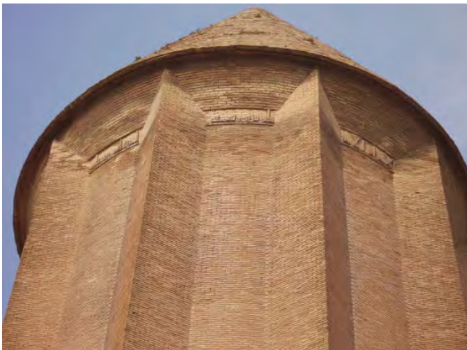
Figure 83 - location of conical roof joining the body
