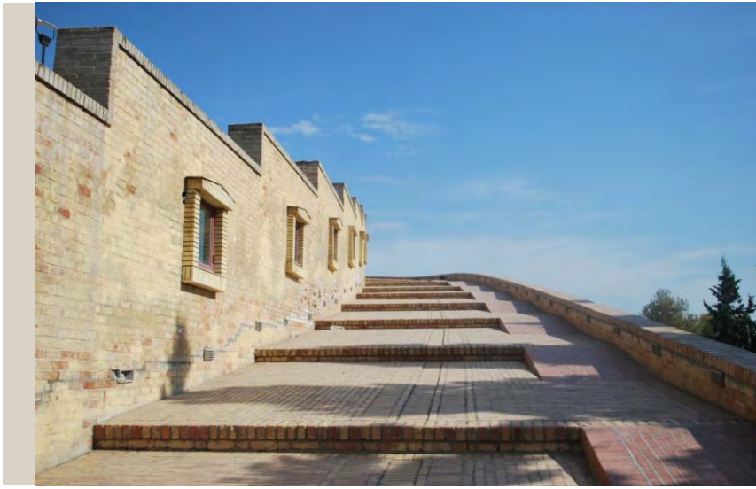
13 Passage way to the site
