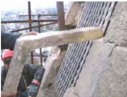
Figure 87 - The Typical fringed bricks used in the conical roof
