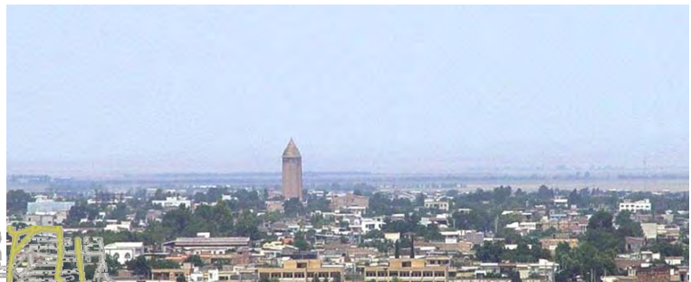
Figure 34 - . Gonbad-e Qābus, View from Azad Shahr area
