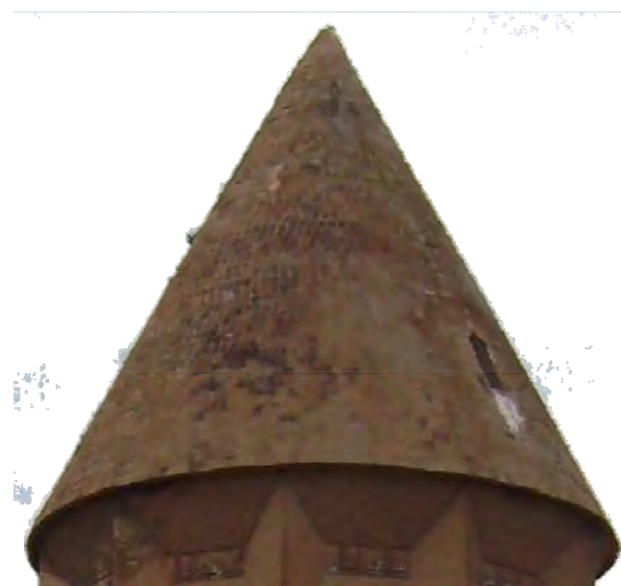
Figure 55 - View of Conical Roof
