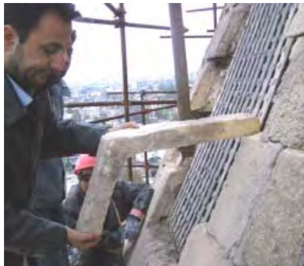
Figure 61 - The typical brick fringed used in the conical roof
