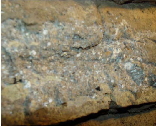
Figure 85 - Inseparable Mortar used in the foundation.
