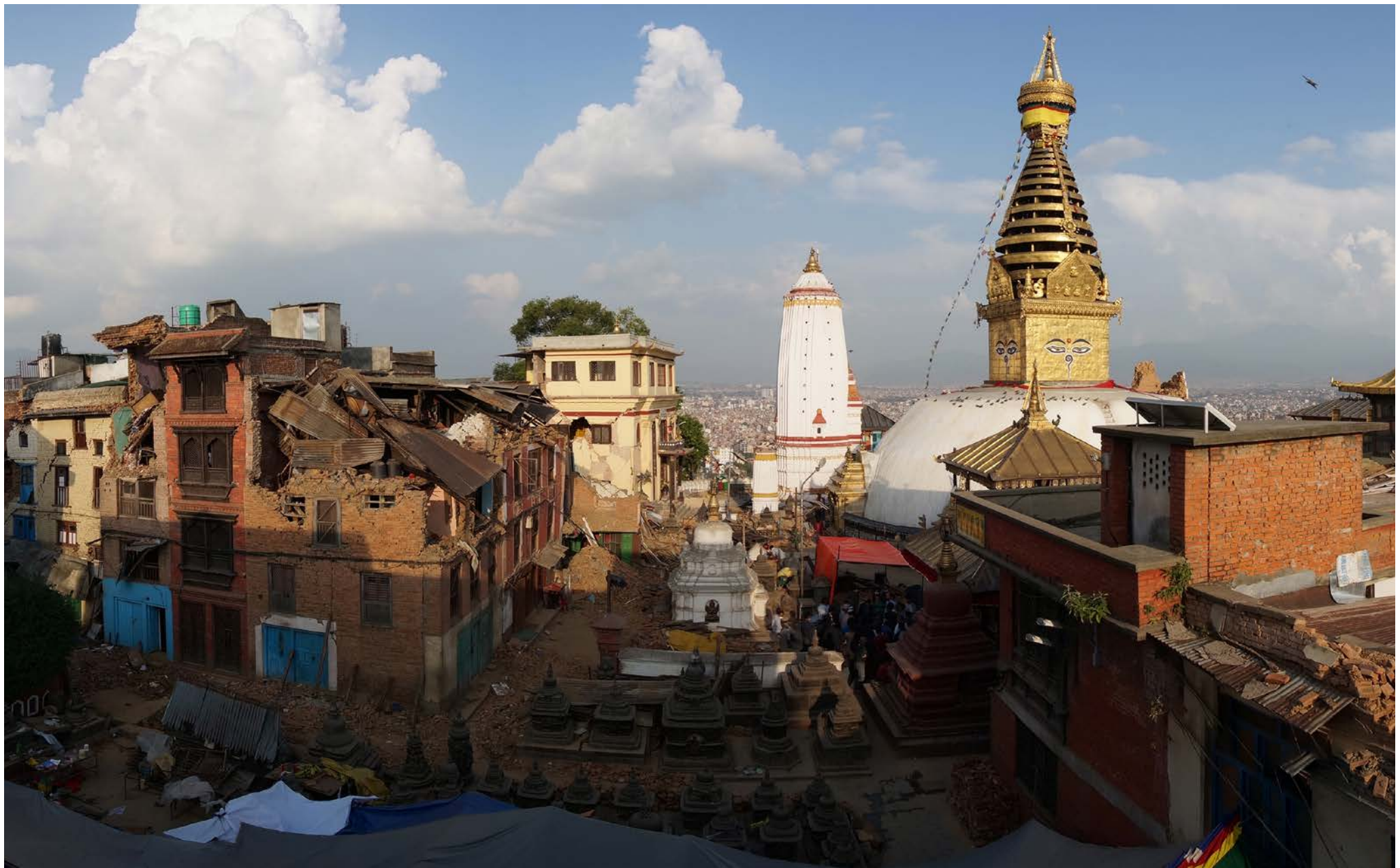
View towards the East | May 2015
