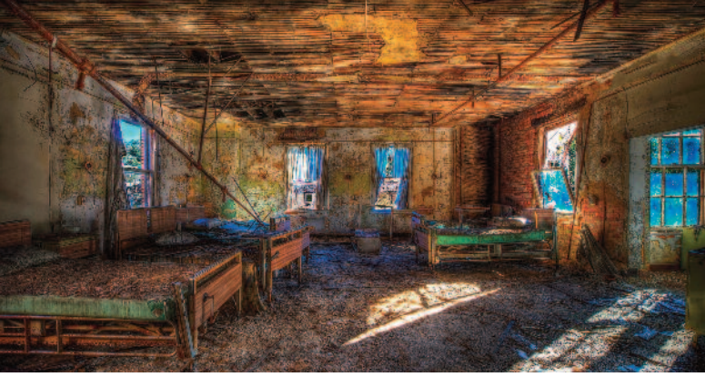
Abandoned hospital in Pittsburgh (USA) © Brook Ward/Flickr.com*
