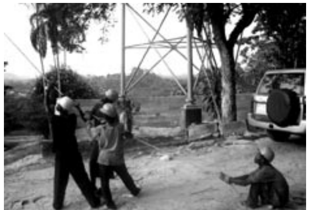
Local development works, Bong County : UNDP Liberia
