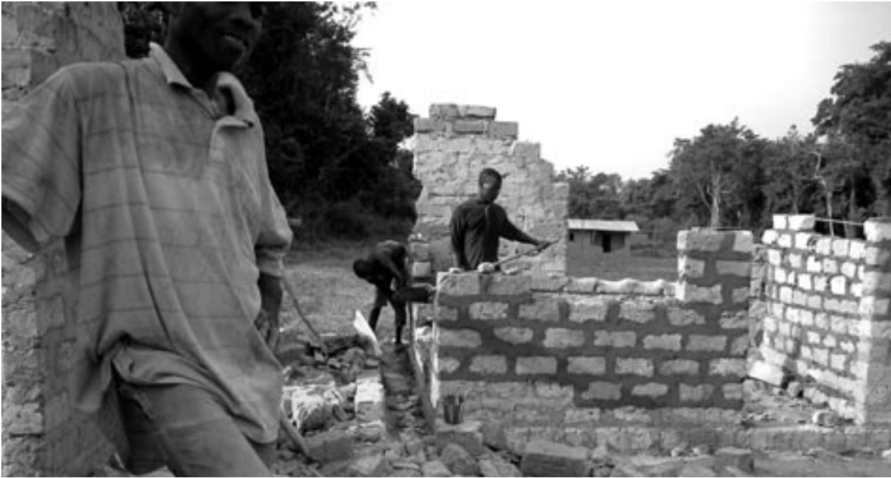
Rebuilding works in the outskirts of Monrovia : UNDP Liberia
