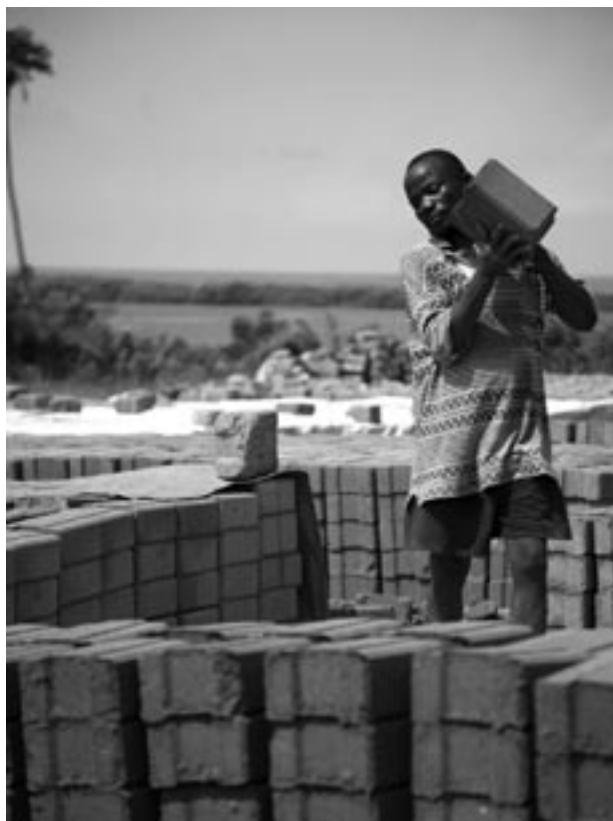
Traditional Liberian bricks being stacked at a brick factory in Monrovia : UNDP Liberia
