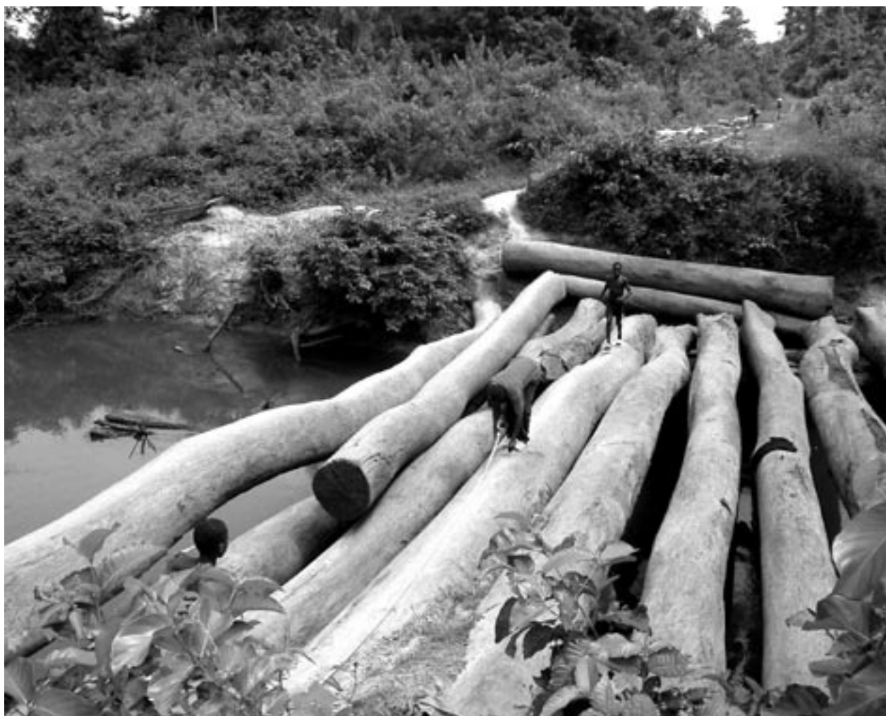
An old bridge, Nimba County : UNDP Liberia
