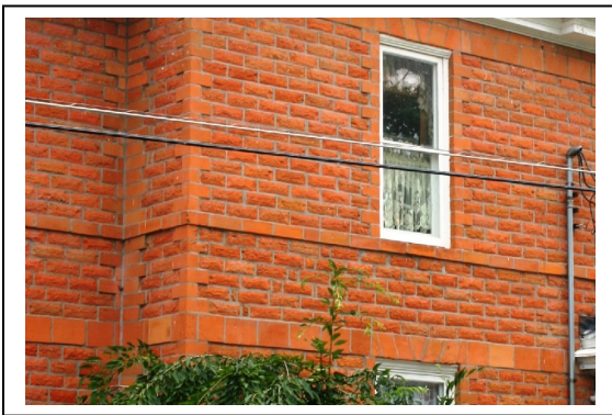
Fig- 2 : Brick Masonry building
