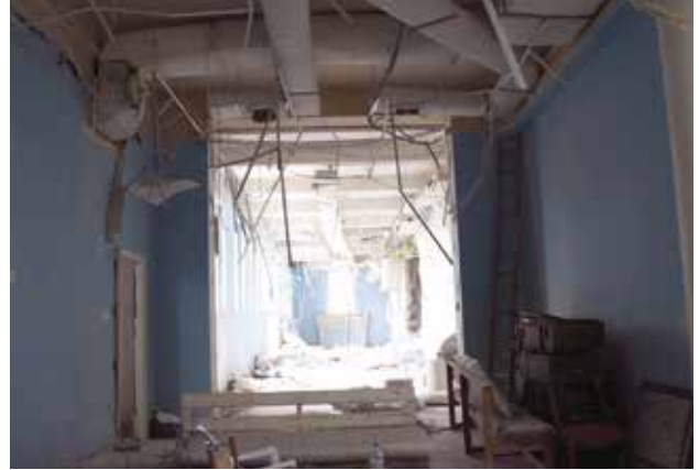
▲ DAMAGE AT THE MUSEUM OF PALMYRA © UNESCO
