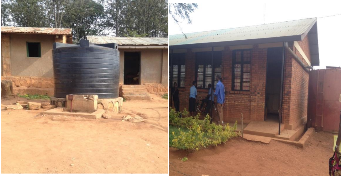
Figure 3: Rainwater harvesting system in one of the Primary school in Gatsibo District
