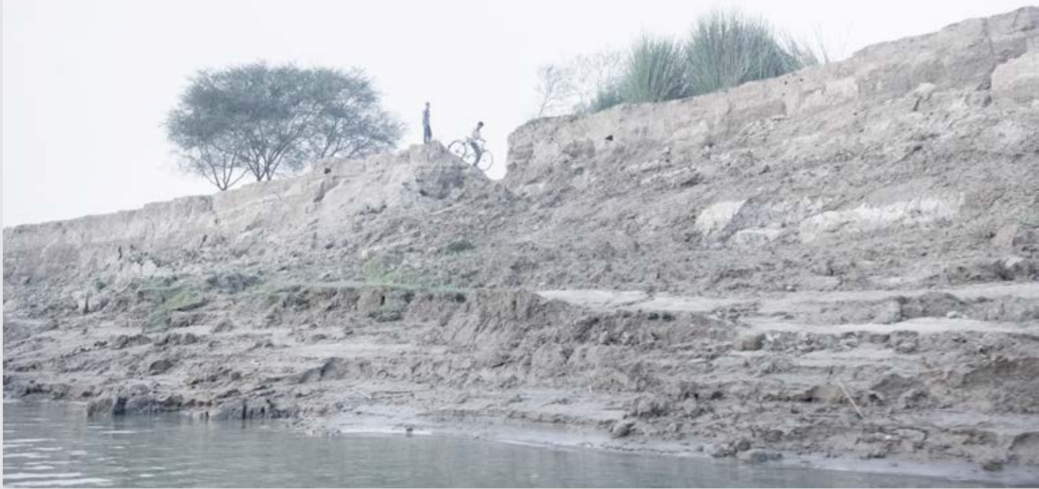
Two men advance cautiously along a river bank that has collapsed.
